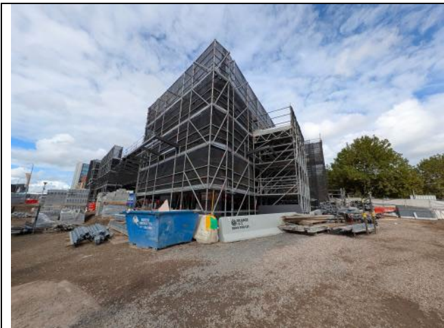
Figure 7 – Bankstown Station - Brick works and block works, roofing, utilities works ongoing on Sydney Trains side plaza areas.
