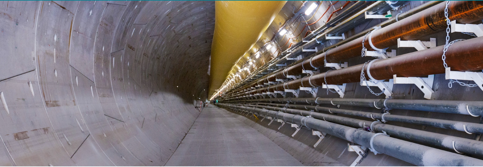
The tunnel floor (invert) behind TBM Jessie.
