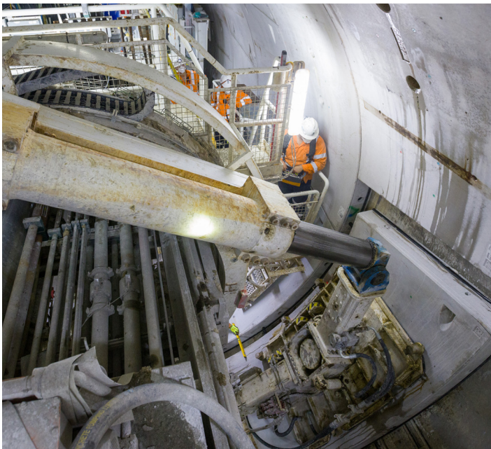
A concrete segment is installed in the tunnel on TBM Ruby.
