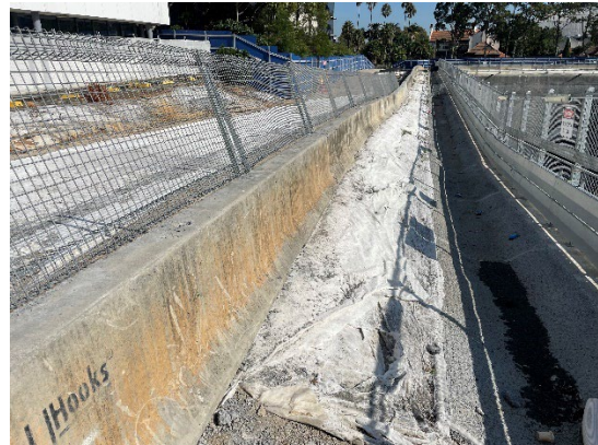
Figure 1.8 Concrete barriers moved to separate different portions of the site (SOP).
