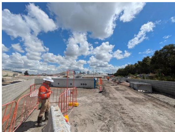
Figure 2.14 – Clyde MSF East: BioBasin construction ongoing.
