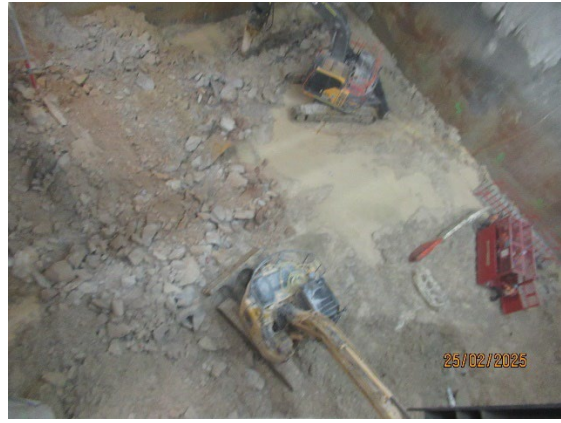
Figure 3.8 Pyrmont West: Excavation under the low roof of the acoustic shed.
