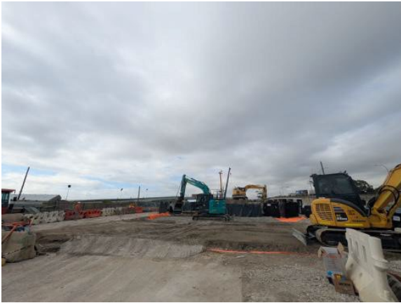
Figure 2.9 – Clyde Dive: Piling pad preparatory works for HV protection slab.
