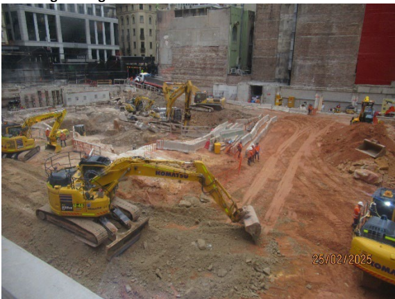
Figure 3.3 Hunter St West: Removal of spoil and footings.
