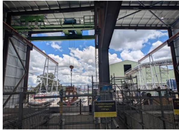
Figure 2.16 – Rosehill Site: Segments lifted via gantry crane.
