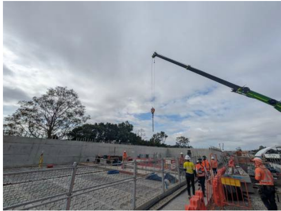
Figure 2.10 - Clyde Dive Site: Plank placement on deck above Dive structure.
