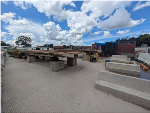
Figure 2.15 – Rosehill Site: Refurbishment and maintenance works of cross passage ramps.
