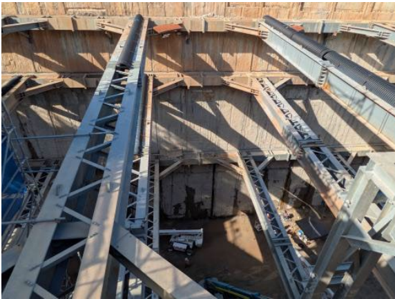
Figure 2.1- Parramatta Site: Eastern Station Box - D wall rectification works.
