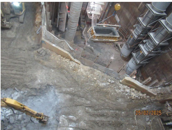
Figure 3.5 Pymont East: Shaft excavation by rock hammers.
