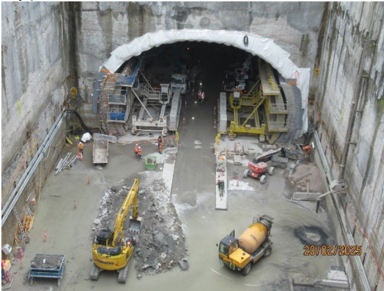
Figure 1.3. Concrete lining FRP works for the central cavern (Five Dock).
