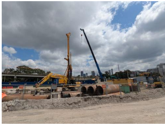
Figure 2.12 – Clyde MSF West: Piling works for future flood relief culvert.
