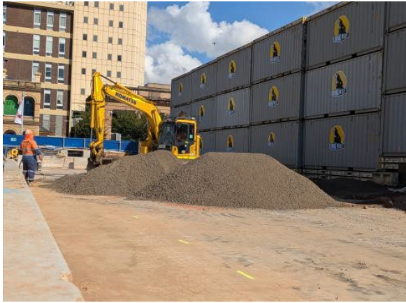
Figure 2.3 – Parramatta Site: Piling pad preparatory works, adjacent to containers.
