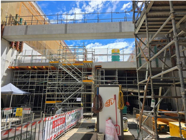
BRD – Station box showing beam installation and FRP.
