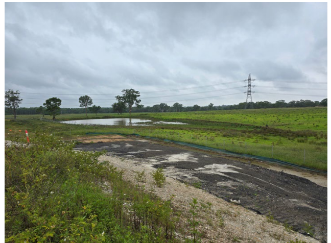
SMF – Northeast sump and pump adjacent to LV road construction.
