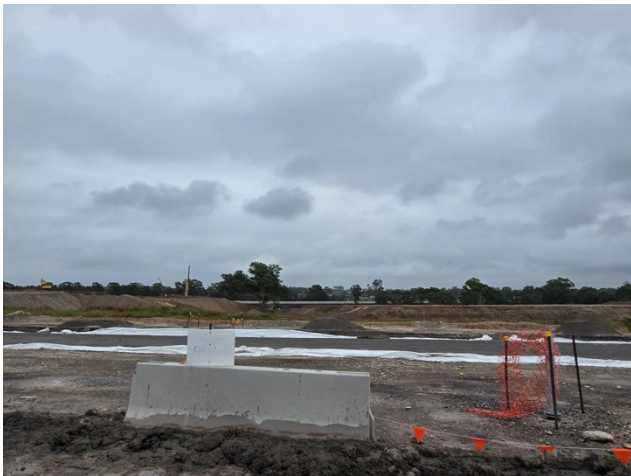
SMF – Permanent stockpile relocation works continued.
