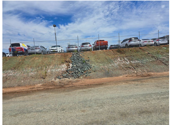
BRD – An opportunity for improvement was discussed with PLM to minimise erosion of the embankment from the LV carpark.
