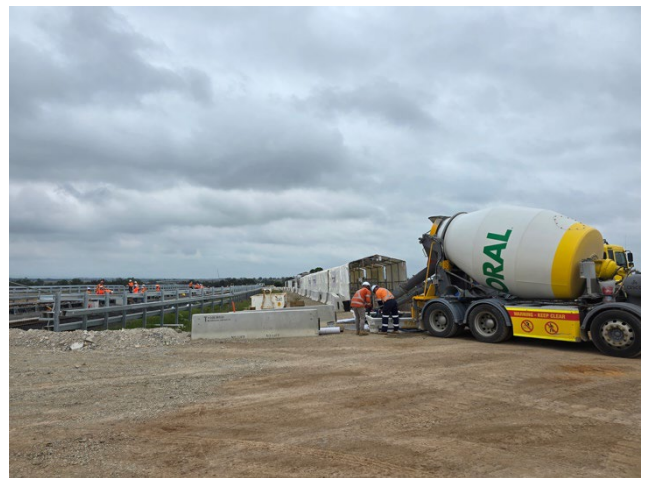
Luddenham to M4 – Concrete washout in designated trays (good practice).
