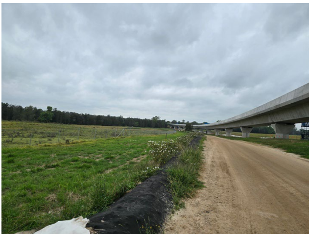
Luddenham to M4 – Weed maintenance continued to be delayed.
