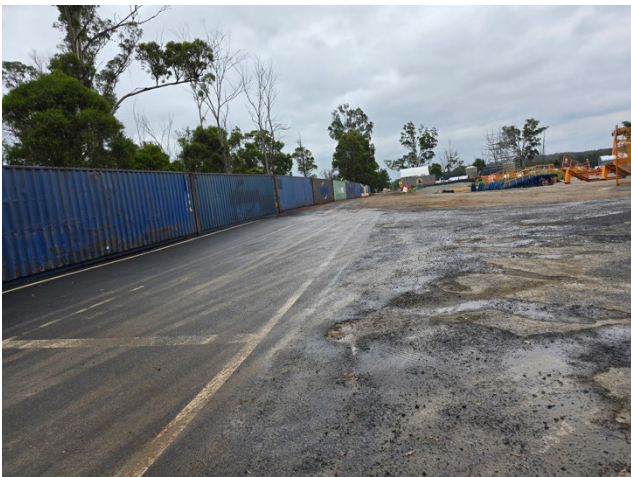
BSF – Installation of the noise wall was completed.
