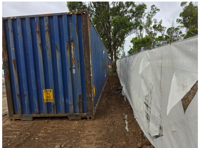
BSF – Additional ESC was required behind the noise wall.
