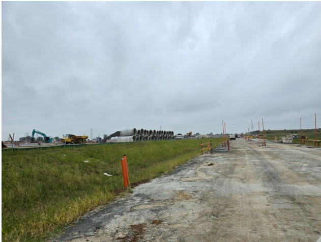
SMF – Permanent drainage works continued.
