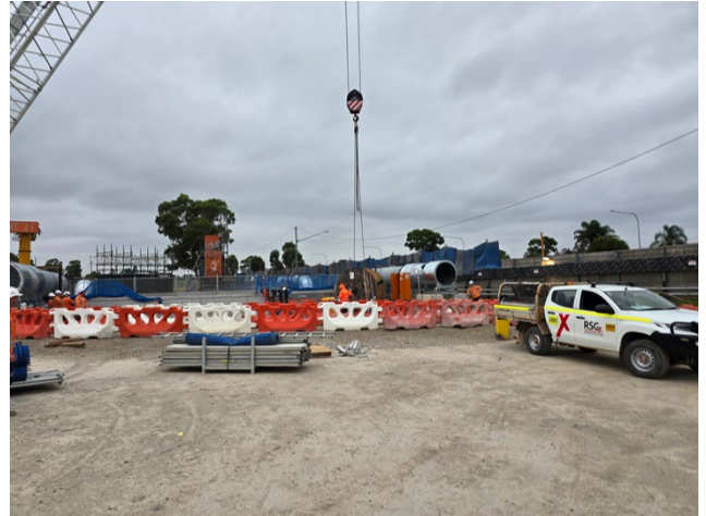
CMSF – It was noted that ventilation installation had commenced.
