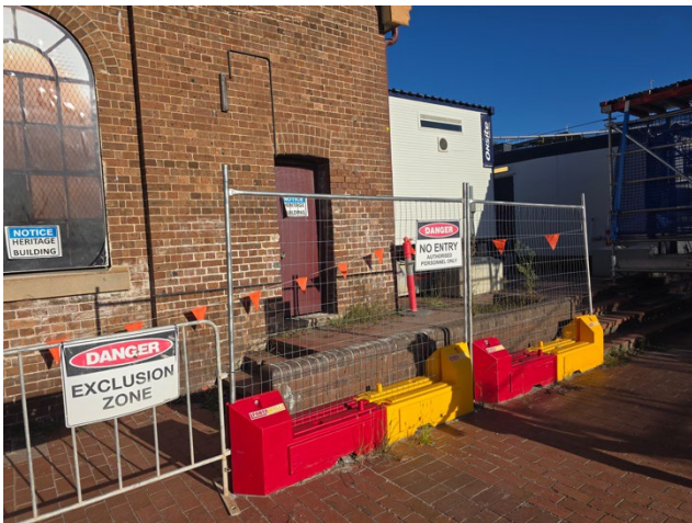
STM – Protection of the heritage building was maintained.
