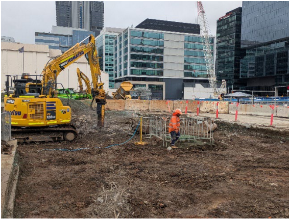
Figure 2.3 – Parramatta Site: Archaeological Zone 8 breakout of footings underway with dust suppression.
