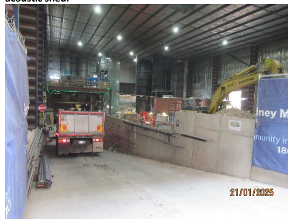
Figure 3.6 Hunter Street East: Trucks accessing the spoil shed.
