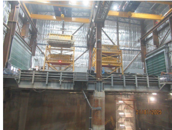
Figure 3.2 Pyrmont East: Kibbles to load trucks with spoil.
