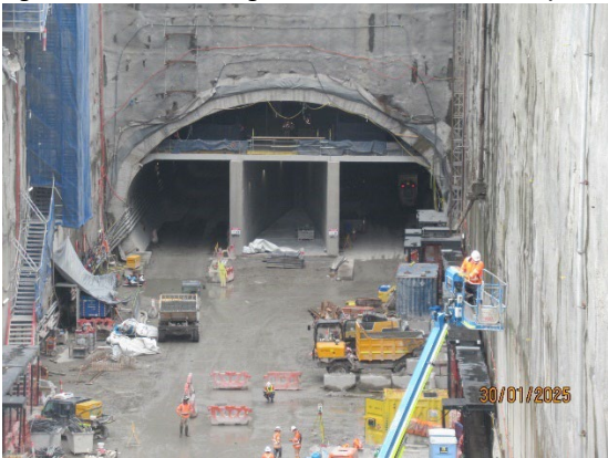
Figure 1.5 Station Box and Plenum (Burwood North).
