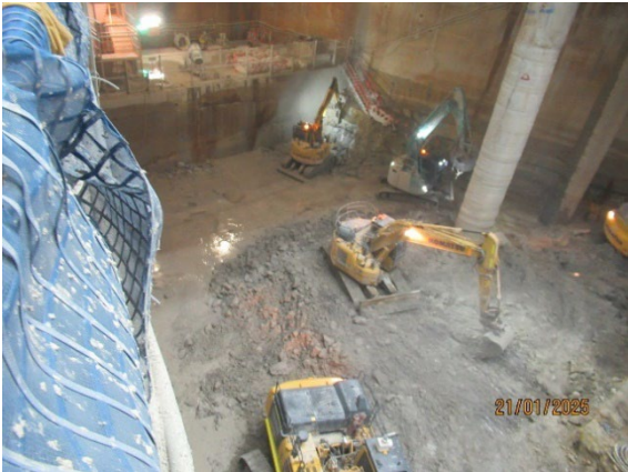
Figure 3.1 Pyrmont East: Shaft excavation by rock hammers.
