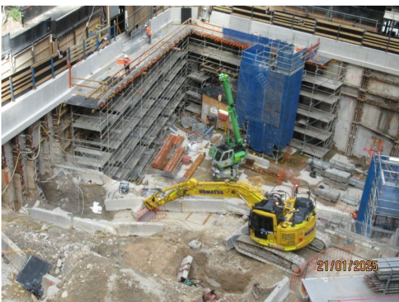
Figure 3.5 Hunter Street East: Works in the SW corner of the site.
