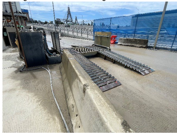
Figure 3.10 The Bays: Wheel wash in place and operating.
