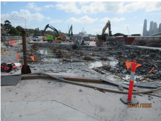
Figure 1.1 Removal of the Spoil shed slab (The Bays).
