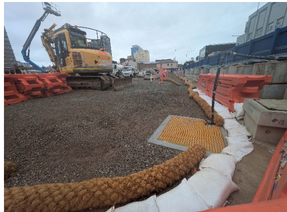
Figure 2.2- Parramatta Site: Archaeological Zone 7 backfilled. Sump and ERSED controls observed in Zone 7 area.
