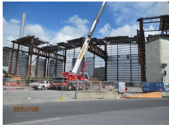
Figure 1.2 Demolition of the Segment Shed (The Bays).
