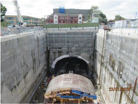
Figure 1.3. Concrete lining works for the central cavern (Five Dock).
