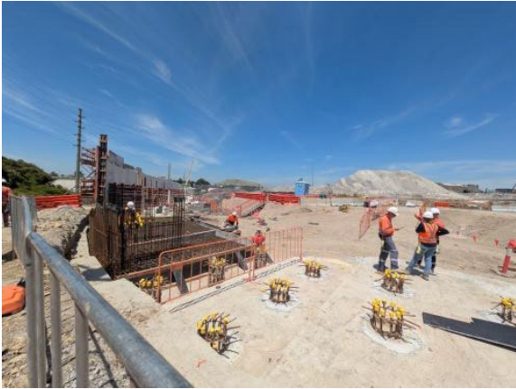
Figure 2.15 – Clyde MSF East – Section 6 - Pile break back for retaining walls.
