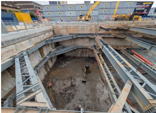
Figure 2.1- Parramatta Site: Excavation ongoing within Western Station Box.
