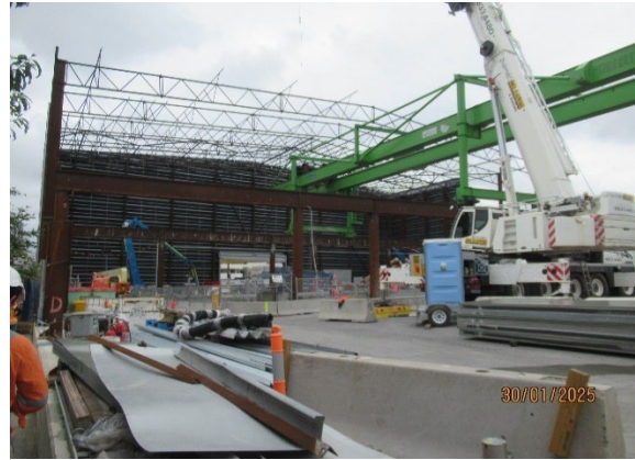
Figure 1.4 Removal of the acoustic shed (Burwood North).
