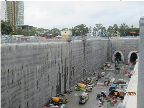
Figure 1.7 Station Box (SOP).
