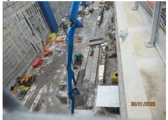
Figure 1.8 Concrete pour for lining of the Nozzles - Station Box (SOP).
