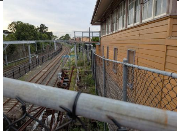
Figure 2 – Canterbury Station – Security fencing works ongoing.
