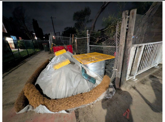
Figure 4 – Wiley Park – King Georges Road – Piles installed previously.
