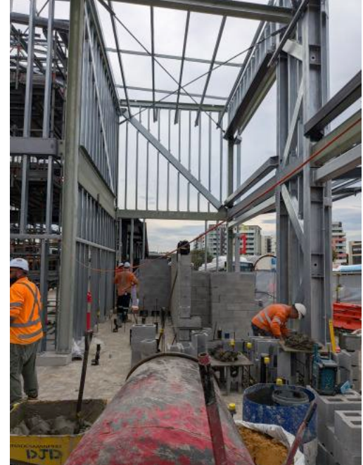
Figure 12 – Bankstown Station – Blockworks and brickwork ongoing.
