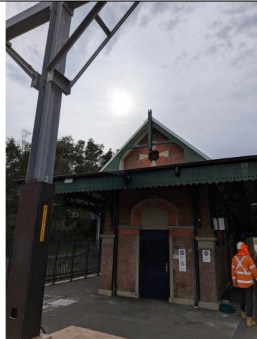
Figure 6 – Canterbury Station - Roof works complete.
