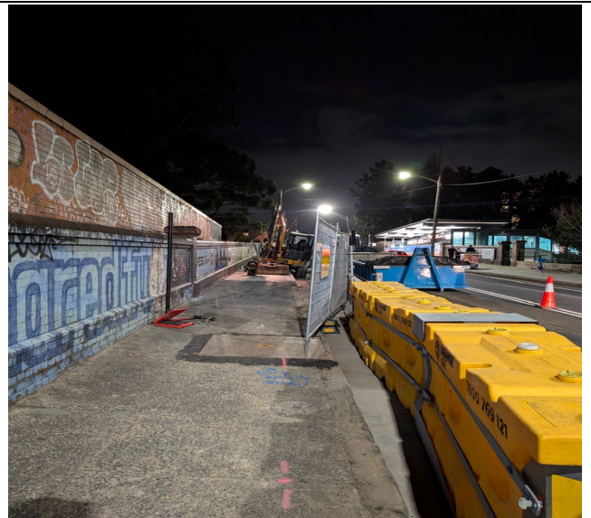
Figure 6 – Illawarra Road, Marrickville – Footpath excavation in progress.
