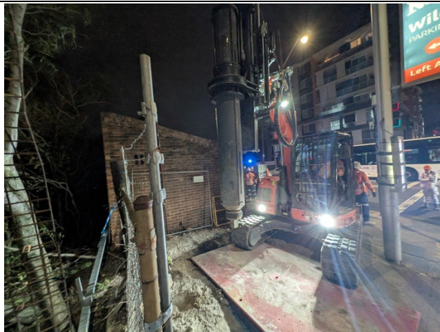
Figure 3 – Wiley Park – King Georges Road – Piling rig being setup.
