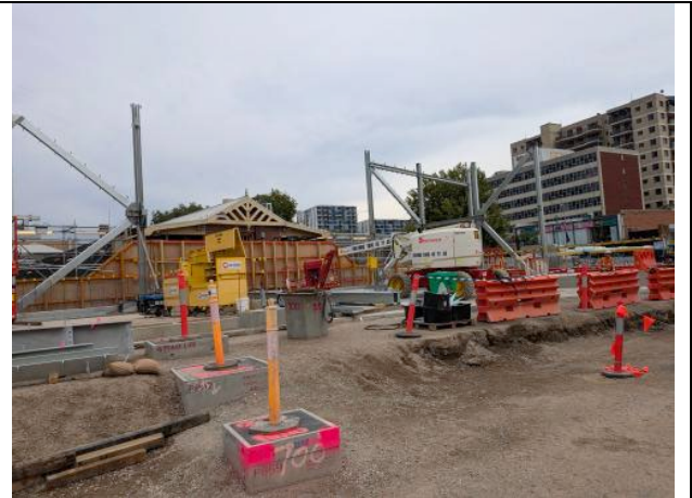
Figure 10 - Bankstown Station - Mechanical, electrical and plumbing works ongoing.
