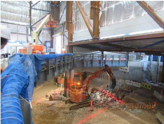
Figure 3.3 Pymont West: Shaft Excavation under the acoustic shed.
