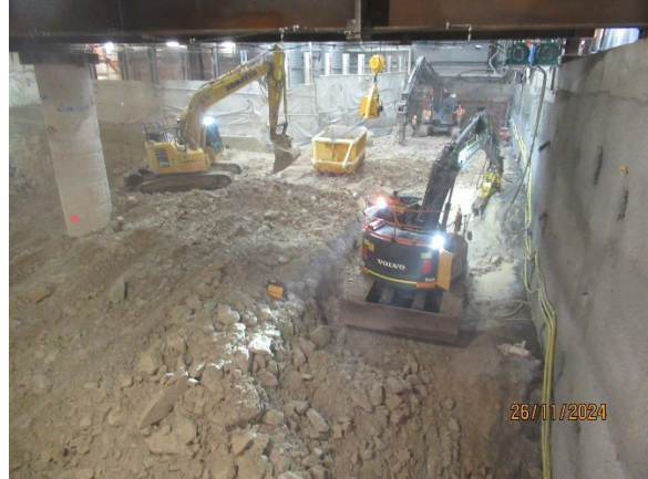
Figure 3.2 Pymont East: Shaft excavation by rock hammers.
