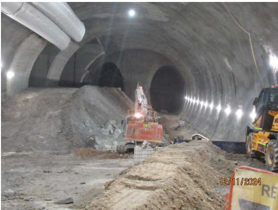
Figure 3.5 Hunter Street East: Cavern excavation and pillar support works.
