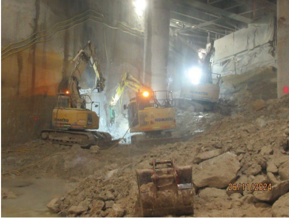
Figure 3.1 Pymont East: Shaft excavation by rock hammers.
