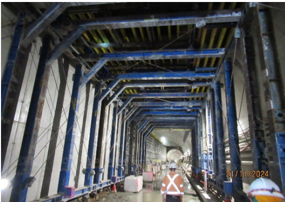
Figure 1.3 Formwork in use for the Plenum concrete pours (Burwood North).
