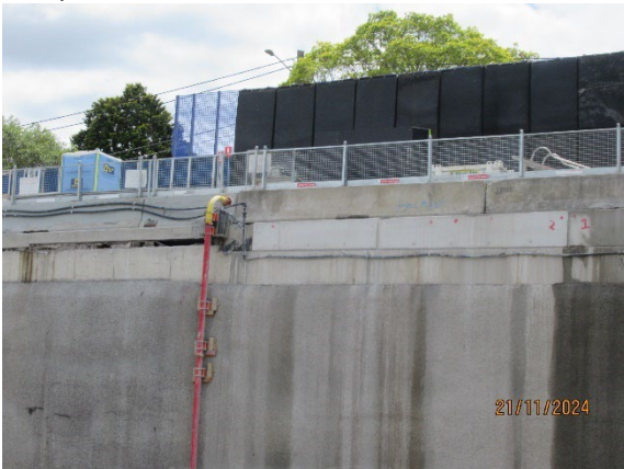
Figure 1.5 Concrete drop chute and noise matts (Burwood North).
