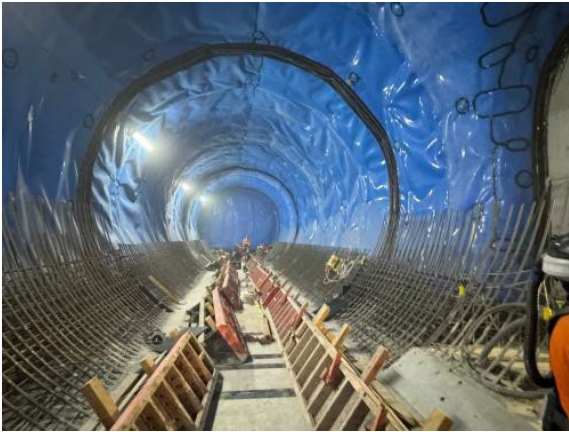
Figure 2.3 – Westmead Site: Ongoing FRP for Stub Tunnel invert slab
