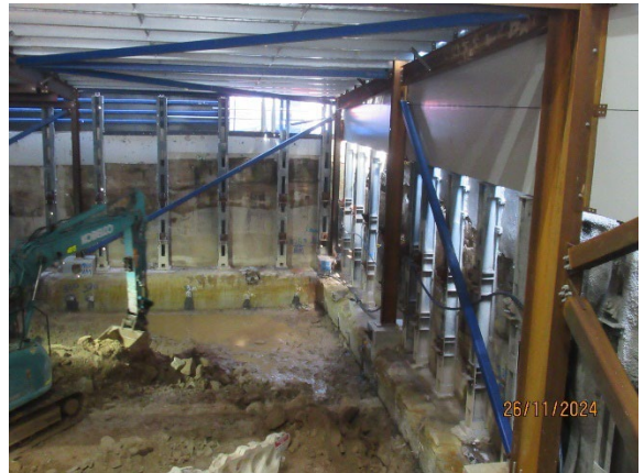
Figure 3.4 Pymont West: Excavation under the low roof of the acoustic shed.
