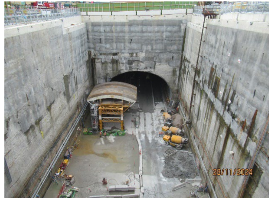
Figure 1.2 Assembly of formwork for the Central Cavern (Five Dock).
