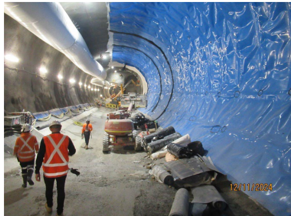
Figure 3.6 Hunter Street East: Water proofing works of tunnel turnback's.
