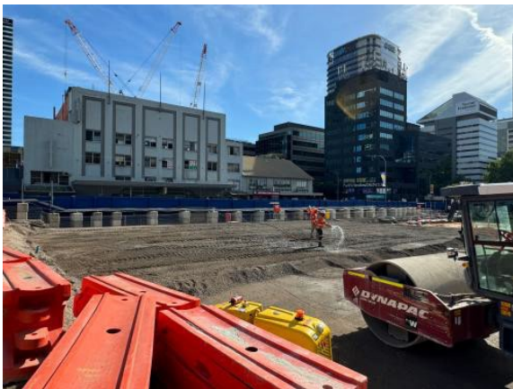
Figure 2.1- Parramatta Site: DGB backfill over cleared Heritage areas – Area 7.
