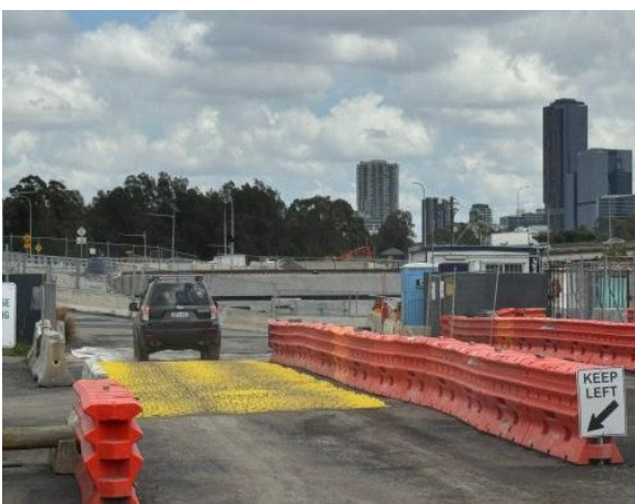
Figure 2.13 – Clyde MSF East Site: Trackout Control Mats placed at exit from MSF East Site and Offices.
