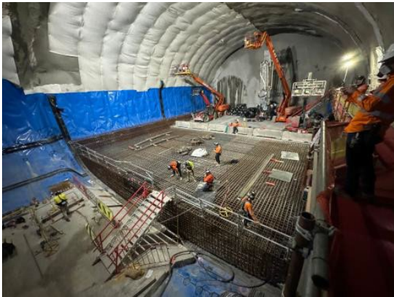
Figure 2.5 -Westmead Site: Steel reinforcement placement for the Crossover Cavern Invert Slab.
