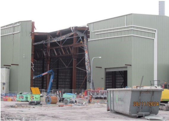
Figure 1.1 Removal of a section of the Segment Shed (The Bays).
