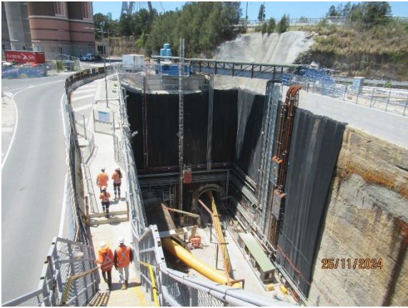
Figure 3.9 The Bays: Both TBMs now in their respective tunnels.
