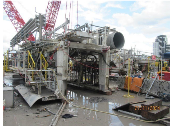
Figure 1.8 Washdown of TBM plant on the surface (SOP).
