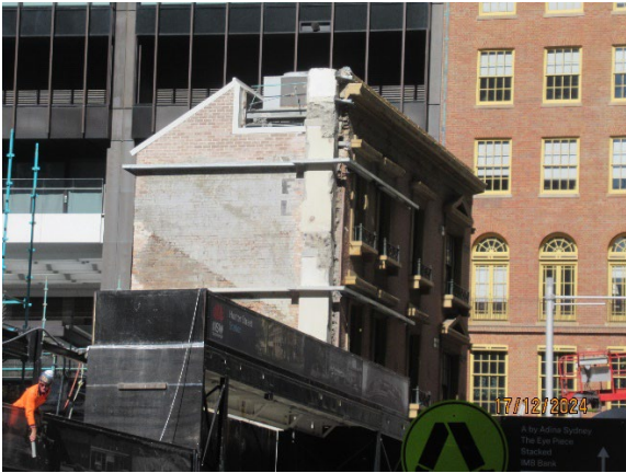
Figure 3.7 Hunter St West: Removal of buildings ongoing around Skinner's Hotel.
