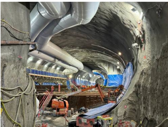
Figure 2.7 – Clyde – Crossover Cavern: Major FRP for invert slabs.
