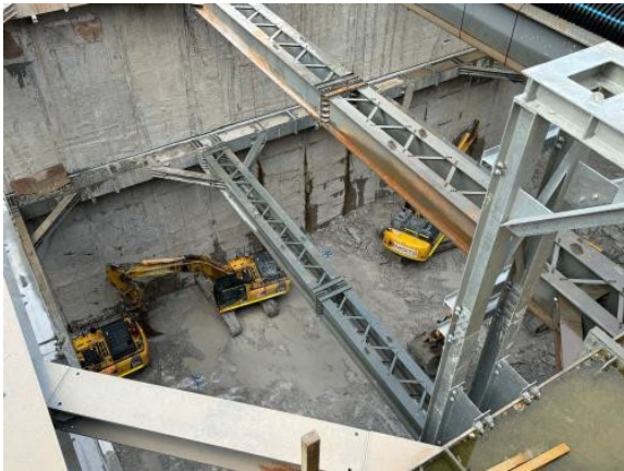
Figure 2.5 - Parramatta Site – Station Box: Hammering occurring.
