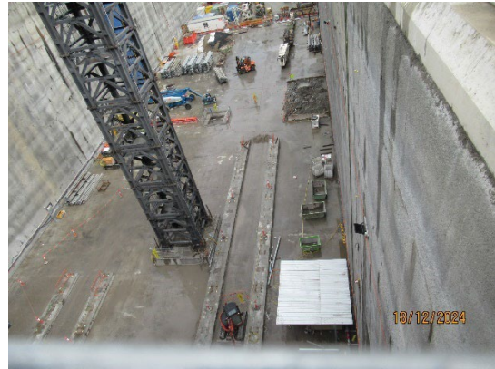
Figure 1.8 Station Box during removal of the tower crane (SOP).
