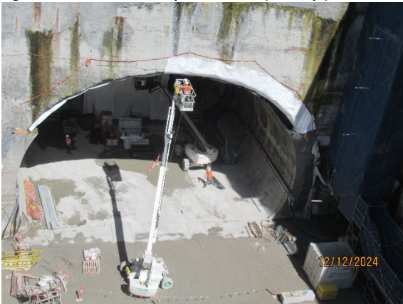
Figure 1.3. Concreting and waterproofing works for the western cavern (Five Dock).
