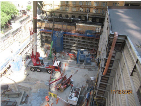
Figure 3.5 Hunter Street East: Wall support around the perimeter of the site.
