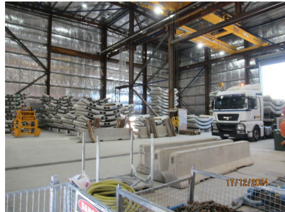
Figure 3.10 The Bays: Ongoing segment deliveries.
