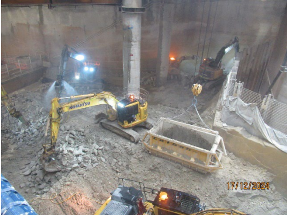
Figure 3.1 Pyrmont East: Shaft excavation by rock hammers.
