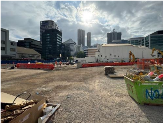
Figure 2.3 – Parramatta Site: Archaeological investigations completed within Zone 7, backfill and compaction ongoing.
