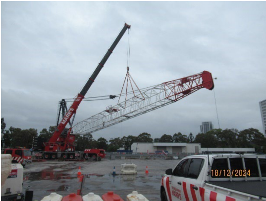
Figure 1.7 Removal of the Tower Crane (SOP).
