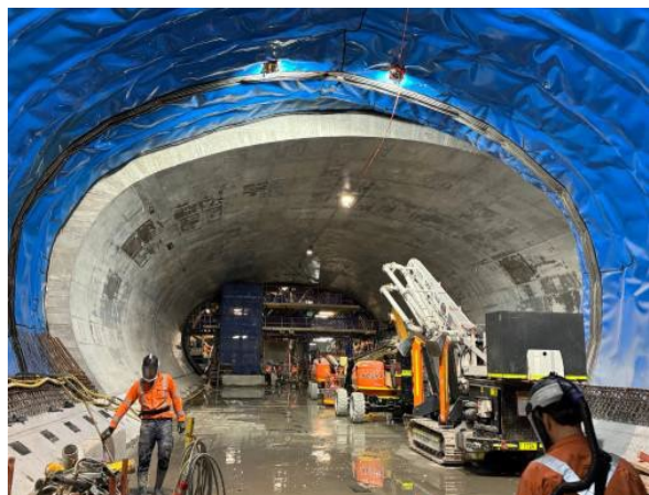
Figure 2.8 – Clyde – Crossover Cavern: Large mobile formwork structures for wall / roof pours.
