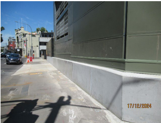
Figure 3.3 Pyrmont West: Shaft B-Class hoarding removed. shed.
