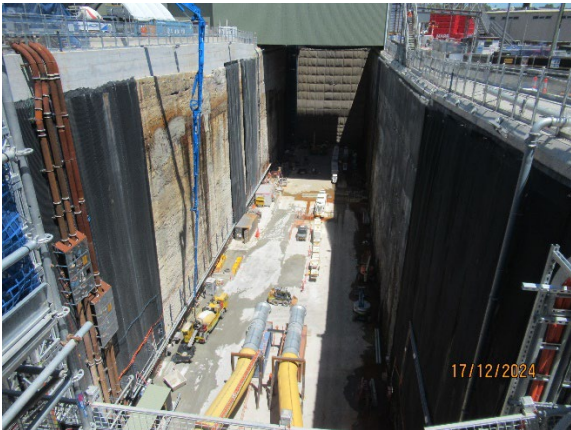
Figure 3.9 The Bays: Ongoing TBM support activities in the station box.
