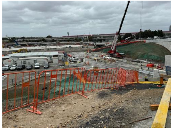
Figure 2.10 – Clyde MSF West: Polymer application had commenced (Unwin St Diversion).
