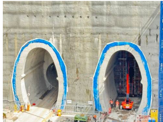
Figure 2.2- SOP Site: Nozzle FRP works at Tunnel RT02.
