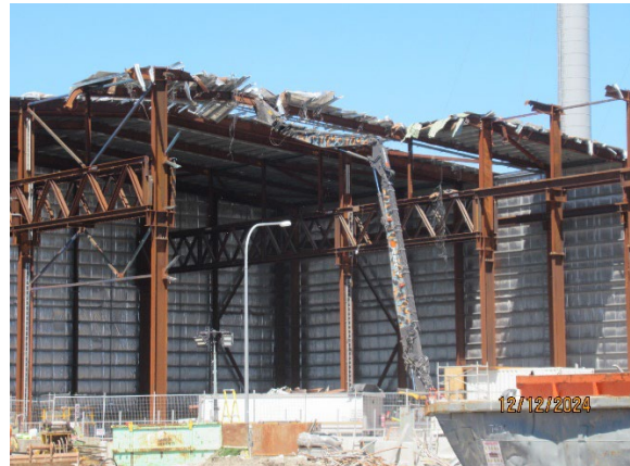
Figure 1.2 Demolition of the Segment Shed (The Bays).
