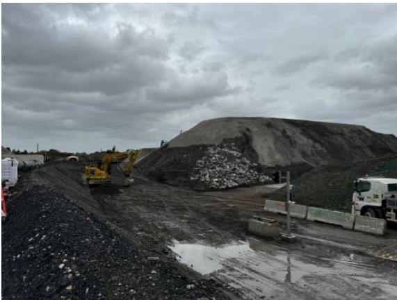
Figure 2.11 – Maintenance being undertaken on internal haul roads, to trim and re-seal ahead of the Christmas Site Shutdown.
