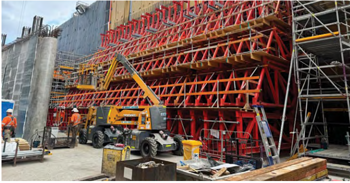
Perimeter Walls of the St Marys Station box being formed.
