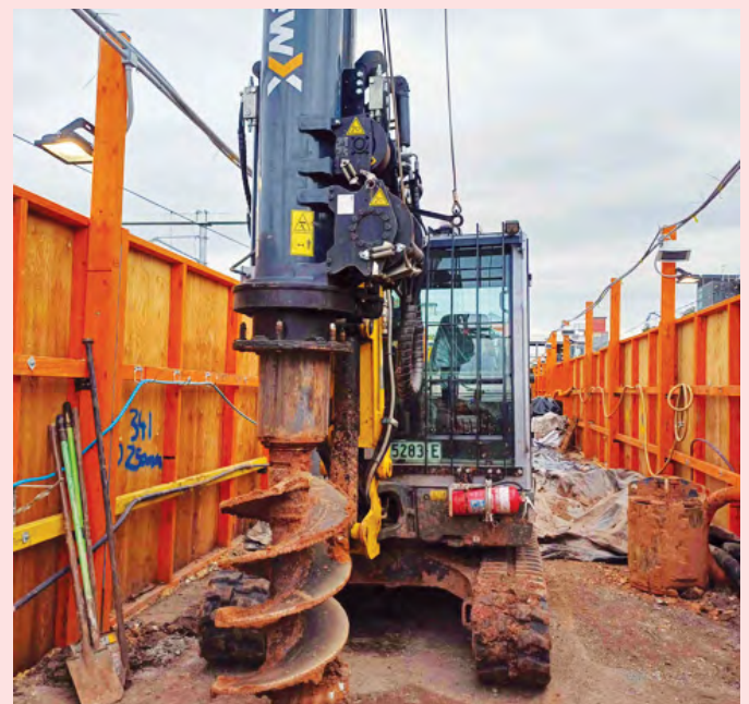
Piling rig fuelled by Hydrotreated Vegetable Oil.
