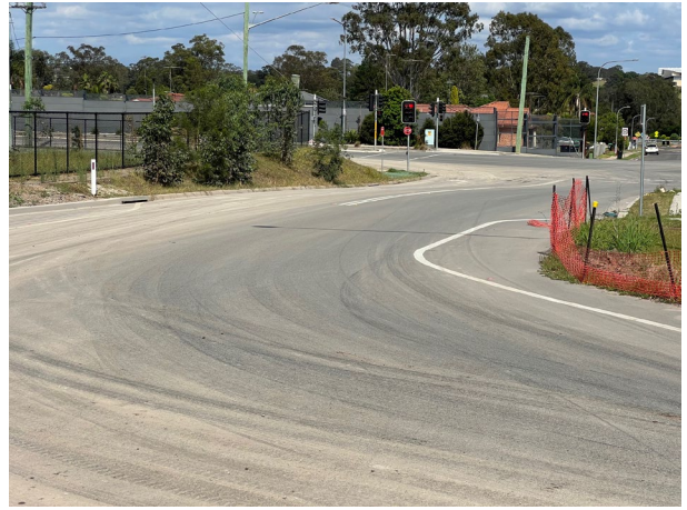
Claremont Meadows: Mud was observed tracked from the HV exit point to Gipps Street
