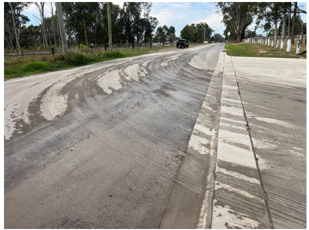
Bringelly: Mud tracking controls were inadequate during the inspection
