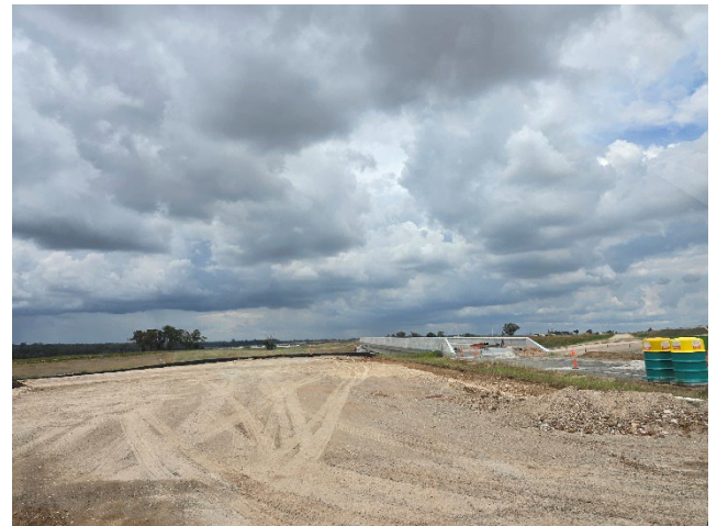
Portion 3 – ERSED bunds installed, preparation for laydown continued
