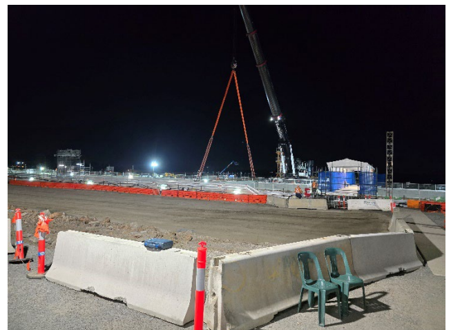
BFD – Beam placement in the box
