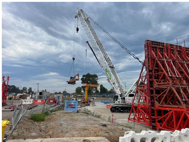
Claremont Meadows: Equipment is being progressively lifted out of the tunnel shaft
