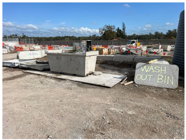
Bringelly: The concrete washout was later formalised with appropriate resources to contain slurry
