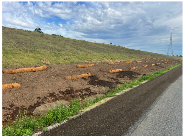
Patons Lane: Salt tolerant vegetation species have been planted on the batters where hydromulch has failed
