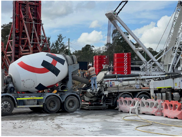
Claremont Meadows: Concrete pouring activities were ongoing during the inspection
