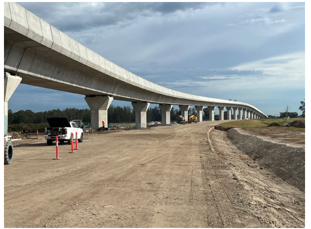
Luddenham North: Northwards view of the completed viaduct
