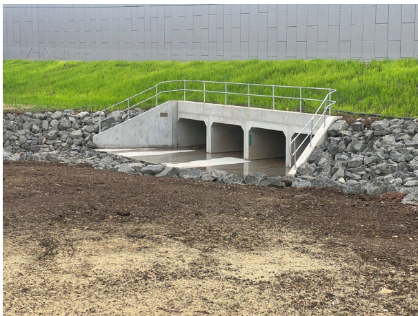
M12 Bridge: The four cell culvert was desilted
