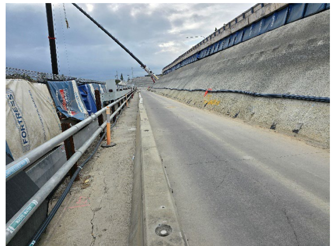
STM – Haul route was maintained
