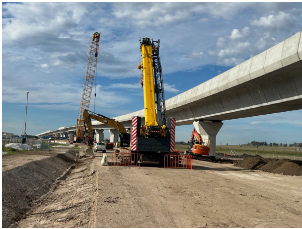
Luddenham North: Parapet work continues on the viaduct
