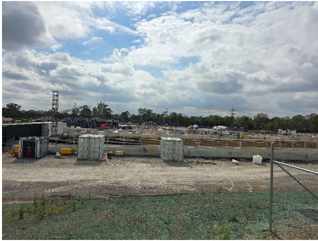
OHE -Box and concrete batch plant
