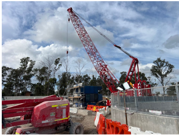
Bringelly: Noise barriers were placed around this crane as a precautionary measure
