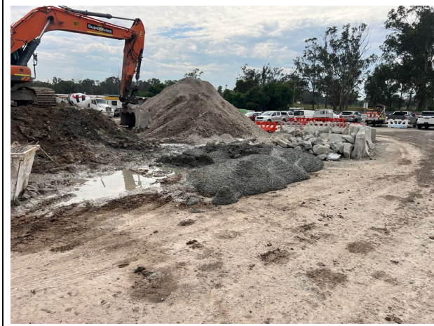
Bringelly: Concrete was washed out in a non-designated area without the appropriate controls
