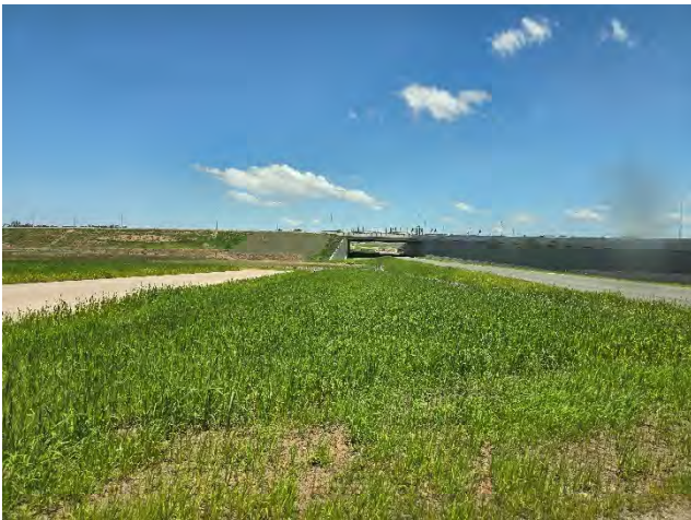
Portion 4 – Site had been handed over to PLM.
