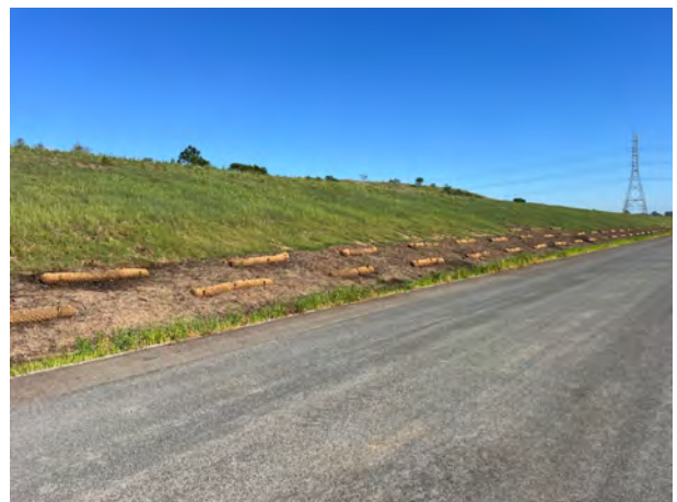
Patons Lane: Salt tolerant species were observed to still be alive on the Patons Lane batter.
