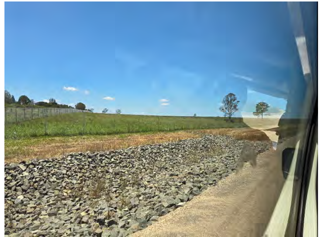
Portion 3 – ERSED rock lined swales were maintained.
