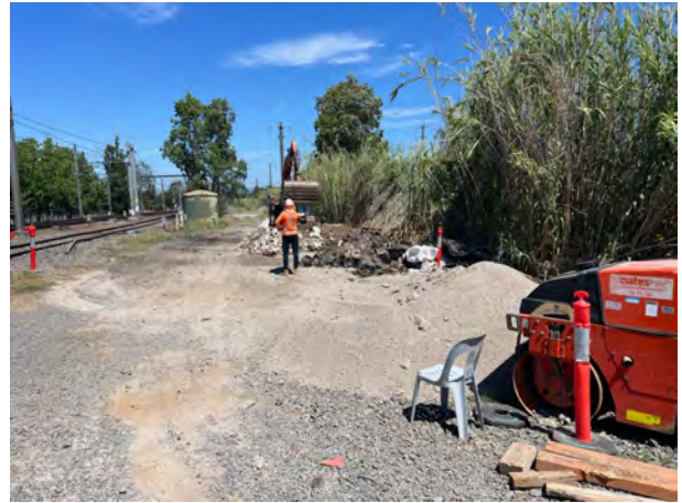
Laydown Area 1: Material was being loaded out from laydown area 1.
