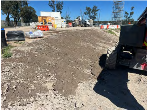
Bringelly: Batters were reshaped awaiting polymer application.
