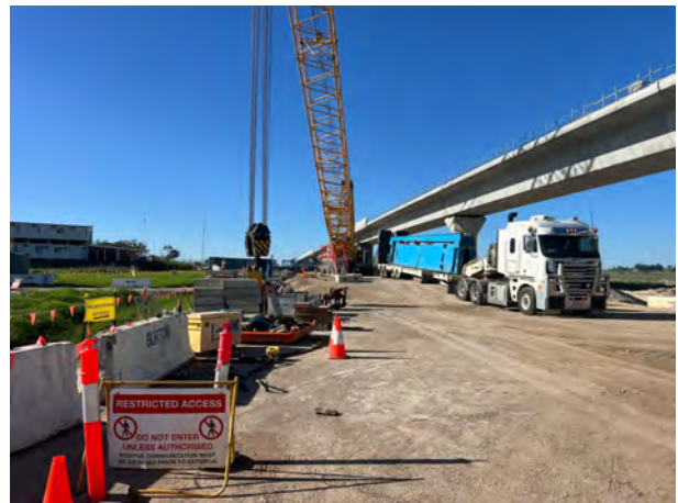
Luddenham North: The gantry was dismantled and transported off site.
