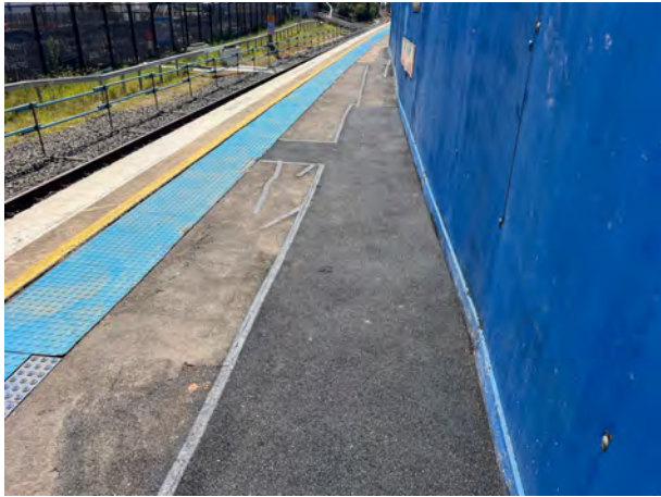
Platform 1/2: Additional asphalt was provided to prevent pooling of rain water.
