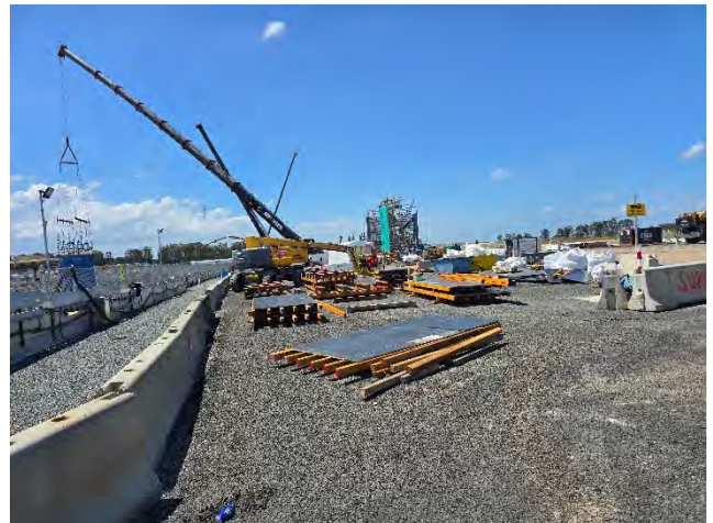
BFD – Pannels being lifted for concrete pours.
