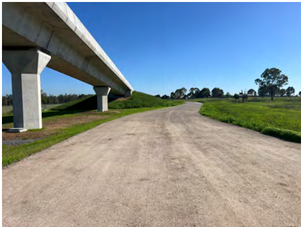
Defence: The haul road is of high quality and should hold up to rainfall.
