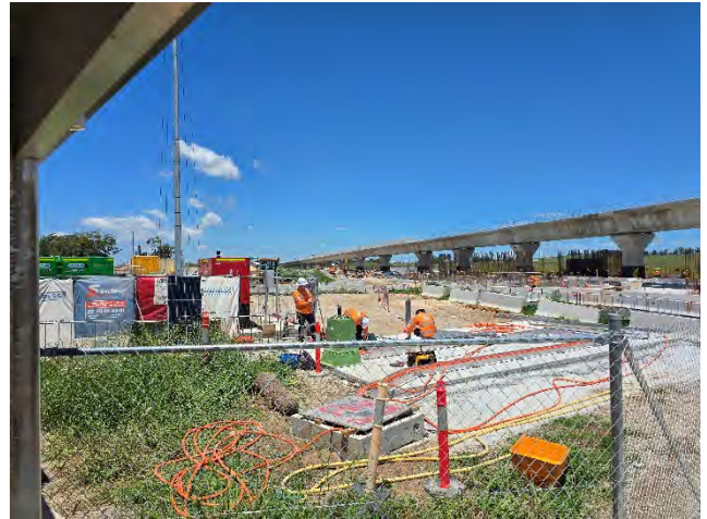
LUD – Works to connect to mains power had commenced.
