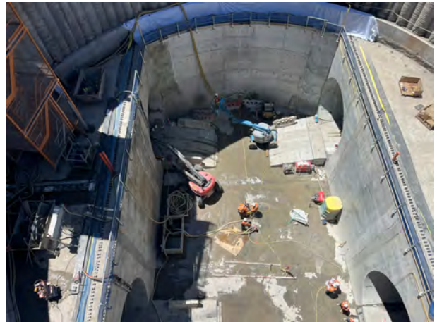
Claremont Meadows: All concrete works in the portal are complete.
