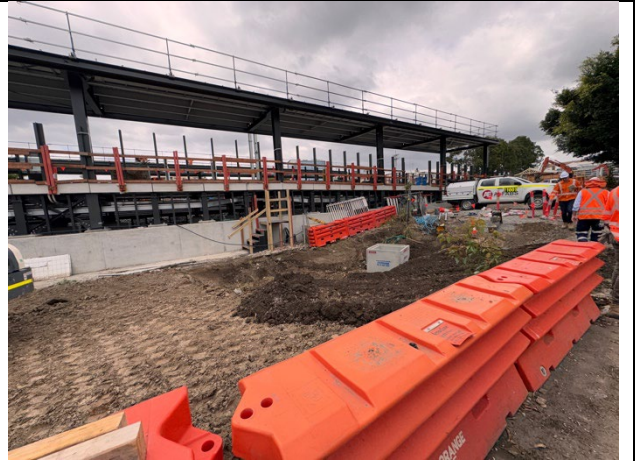
Figure 8 – Bankstown Station – Culvert backfilling nearly complete
