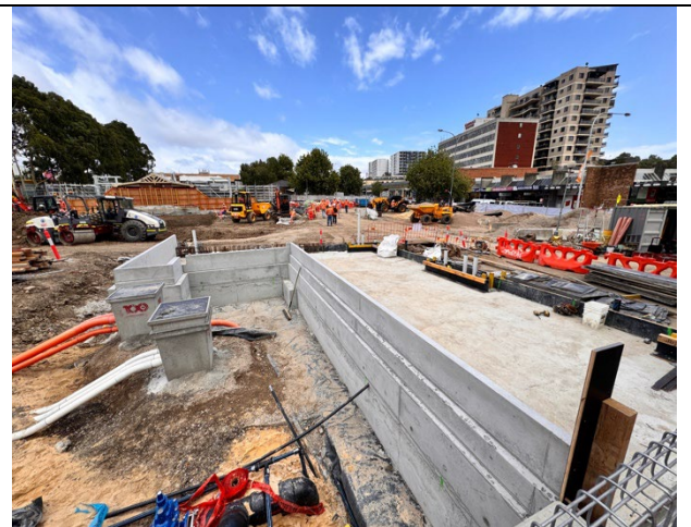
Figure 16 – Bankstown Station – Metro Service Building Concrete pour completed
