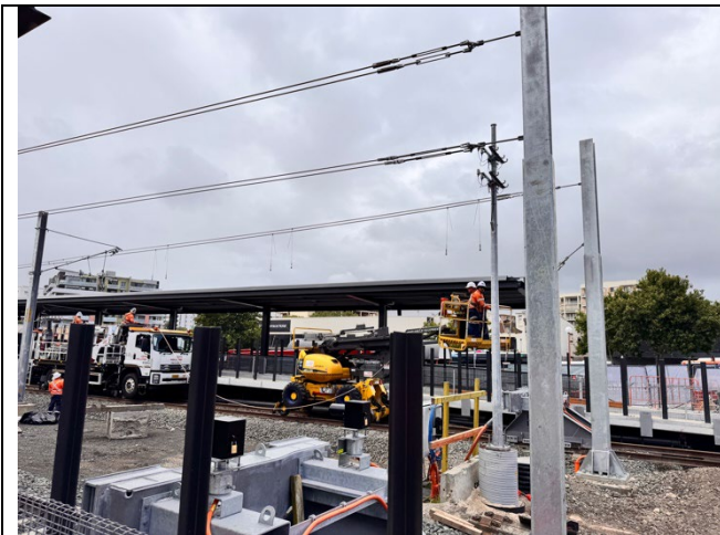
Figure 15 – Bankstown Station – Overhead wiring works in progress
