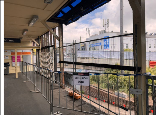
Figure 7 – Exclusion Zone in place after removal of Parcels Office
