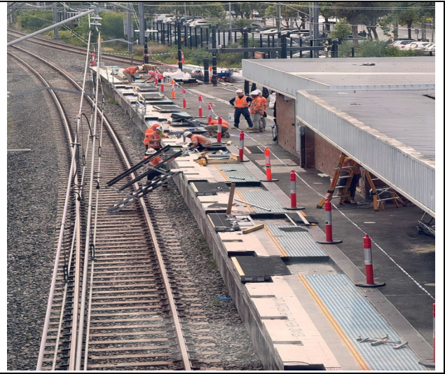
Figure 6 – Punchbowl Station – Mechanical gap fillers being installed
