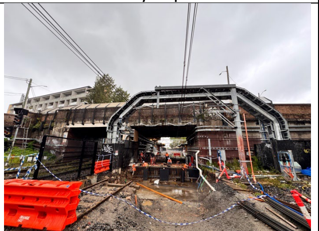
Figure 10 – Marrickville Station – Services being installed under tracks
