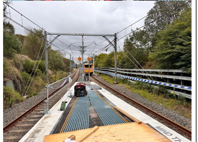
Figure 14 – Belmore Station – Track tamping and regulating being undertaken
