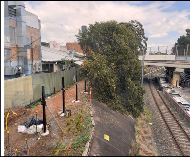
Figure 5: Lakemba Station – Security fencing installation ongoing
