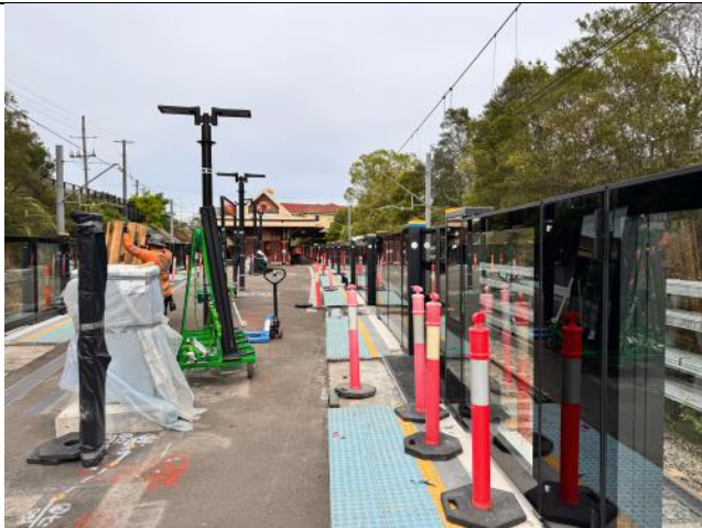
Figure 3 – Belmore Station – Platform screen doors and mechanical gap fillers installation ongoing.
