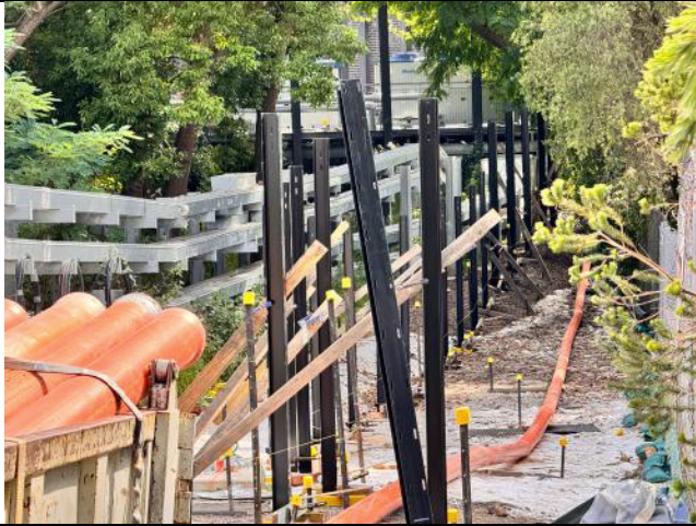
Figure 1 - Hurlstone Park – Security fencing installation ongoing.
