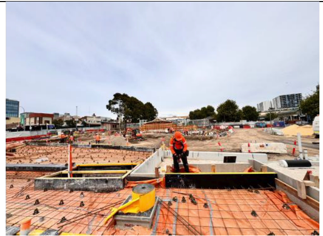
Figure 4 – Bankstown Station – FRP works.
