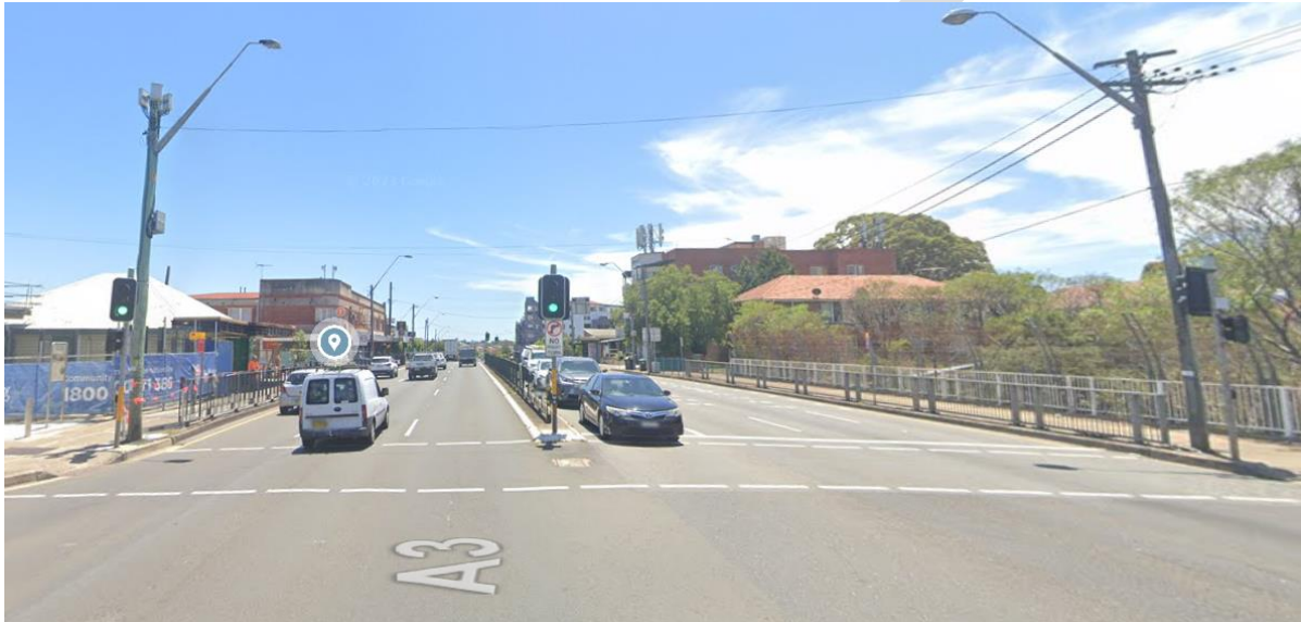
Figure 48: King Georges Road Bridge (Source: Google Maps)
