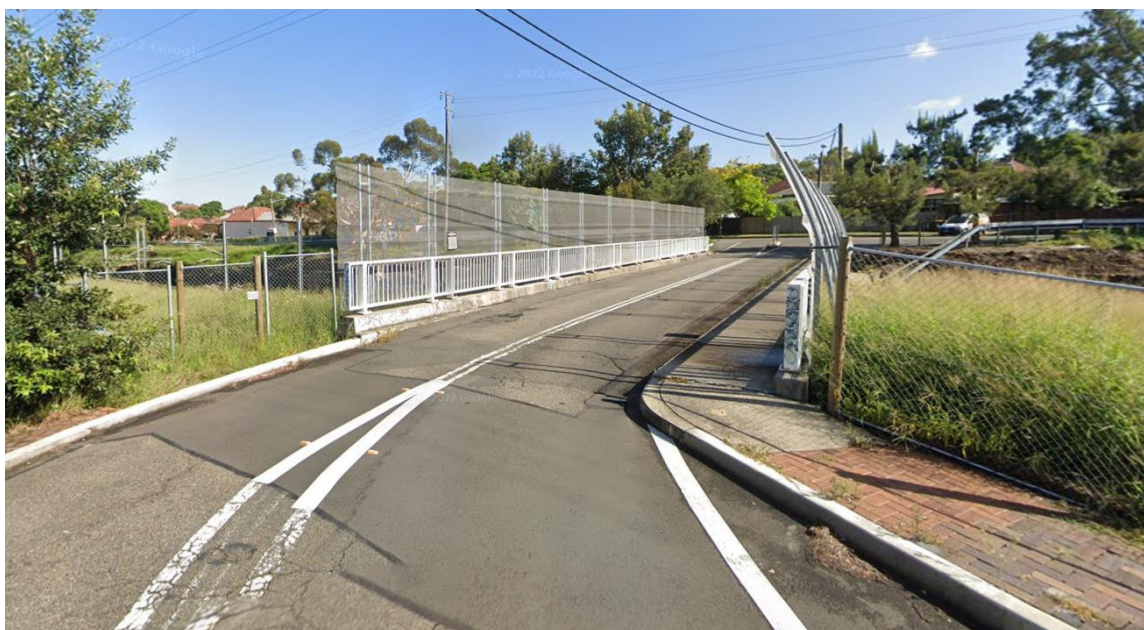
Figure 34: Albermarle Street Overbridge, with Depression era brick paving visible on the right (east) side (Source: Google Maps)
