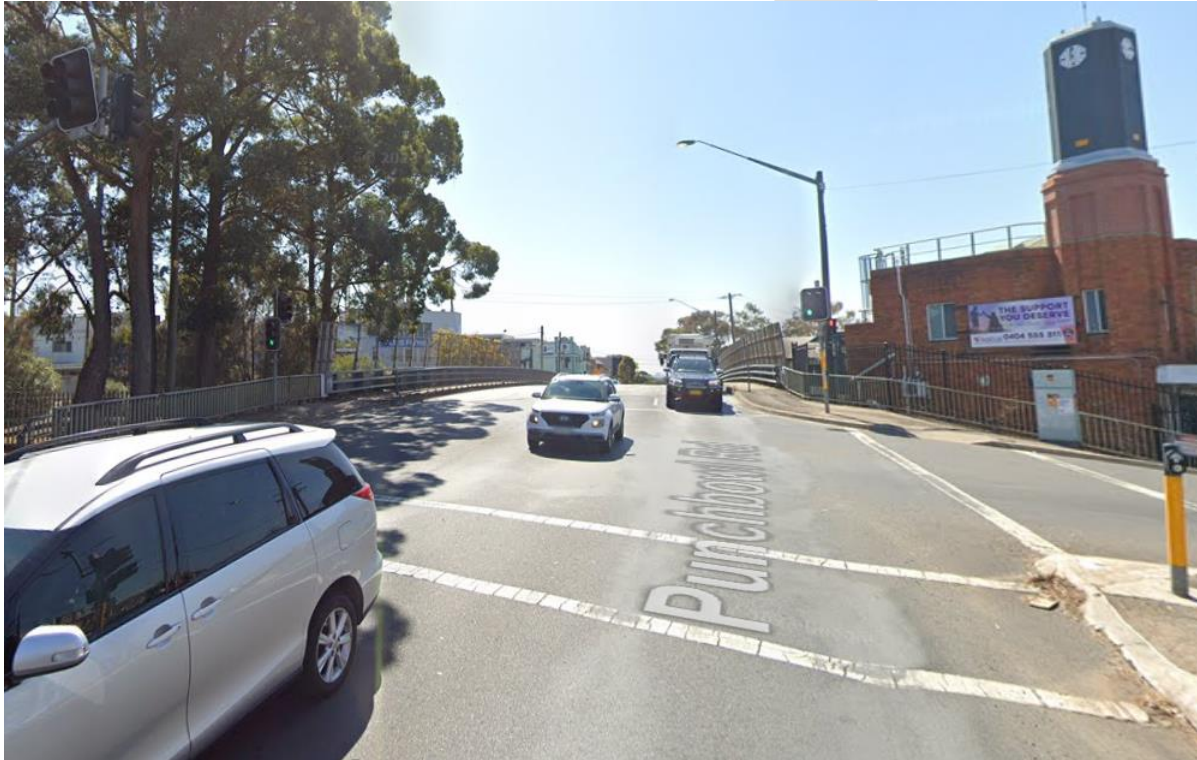
Figure 46: Punchbowl Road Bridge (Source: Google Maps)
