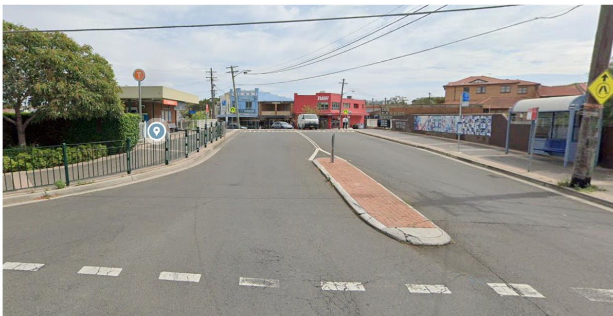
Figure 38: Duntroon Street Bridge (Source: Google Maps)
