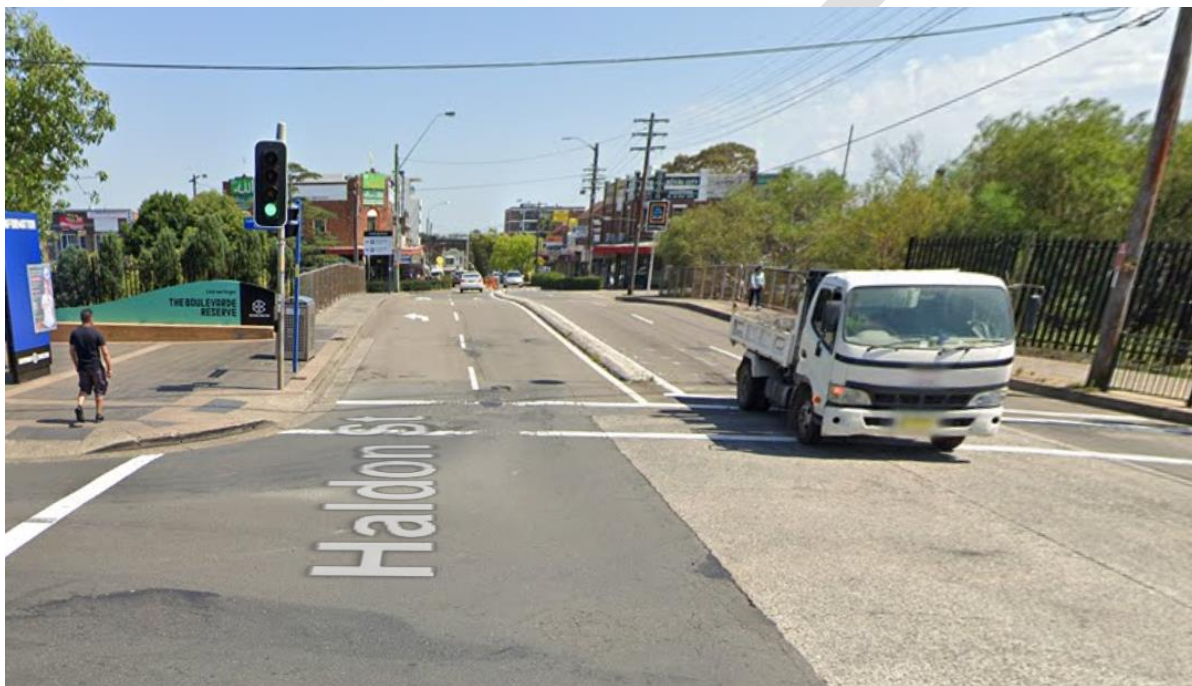
Figure 44: Haldon Street Bridge (Source: Google maps)
