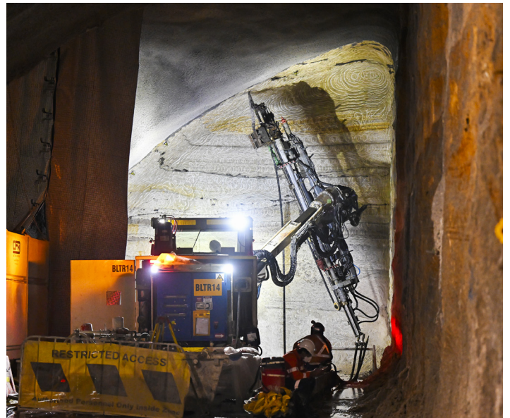
Installing rock bolts in the cavern roof to stabilise the ground.
