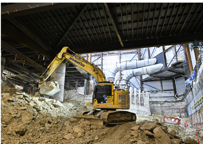
Excavators are used to remove spoil in the station shaft.
