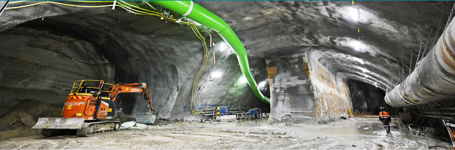
Excavation of the cavern at Pymont Station.
