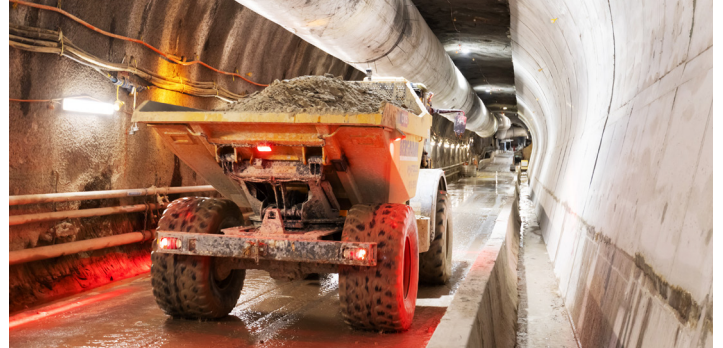
Excavated material is removed from the Hunter Street turnback tunnel.
