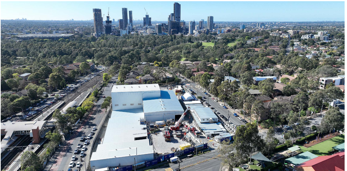
Bird's-eye view: Westmead Metro Station under construction
