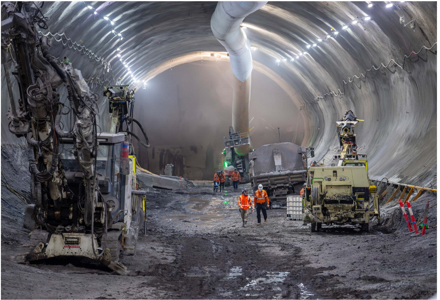
Excavation complete, rockbolting and shotcreting underway at Westmead
