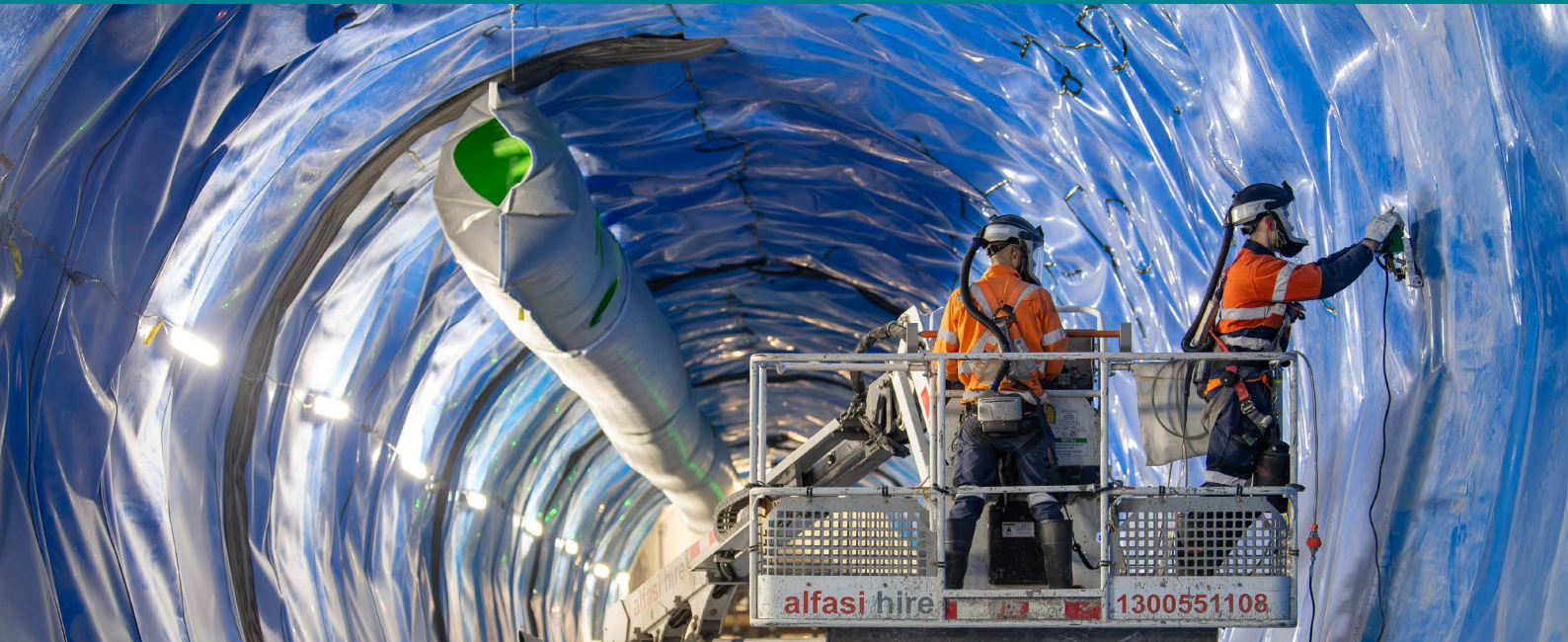
Tunnel waterproofing underway at Westmead
