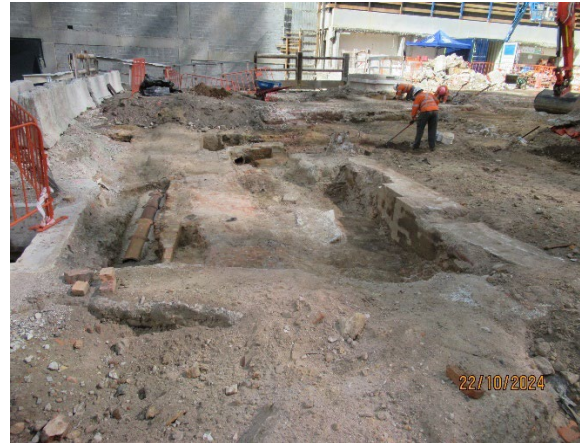
Figure 3.8 Hunter Street West: Archaeological Excavations adjacent the former De Mestre Place.
