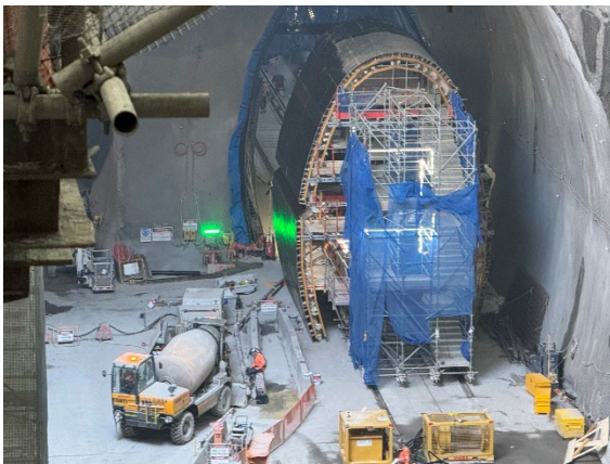
Figure 2.5 -Westmead Site: Nozzle formwork assembly in base of station box.
