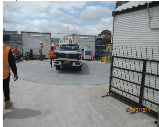
Figure 1.4 Site sheds set up at the south shaft (Burwood North).
