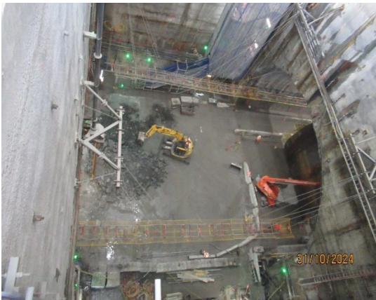
Figure 1.3 Formwork being assembled in the western shaft (Five Dock).
