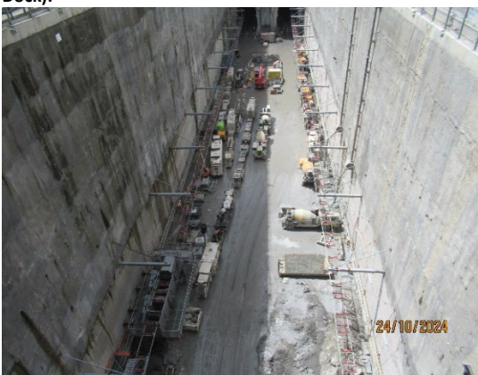
Figure 1.5 Works in the station box (Burwood North).
