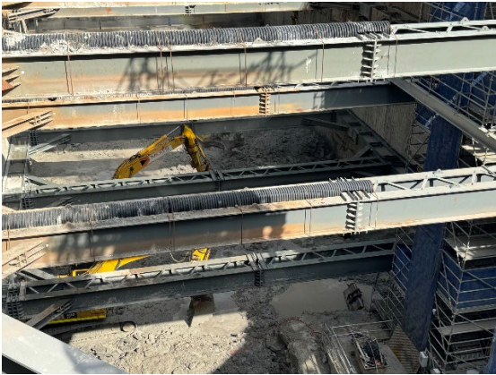
Figure 2.3 – Parramatta Site: Station Box - Sprinklers used during sandstone breakout.
