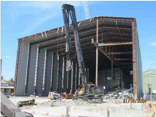
Figure 1.1 Removal of the north end of the Spoil Shed (The Bays).
