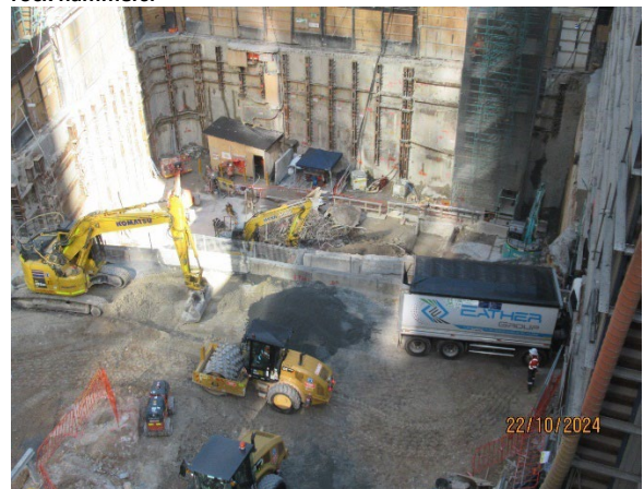
Figure 3.6 Hunter Street East: Piling pad construction.
