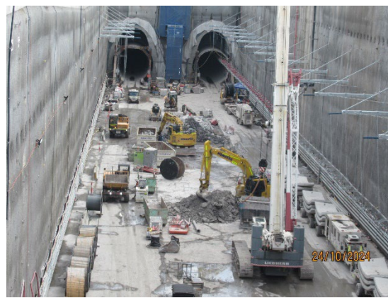
Figure 1.6 Activities in the station box (North Strathfield).
