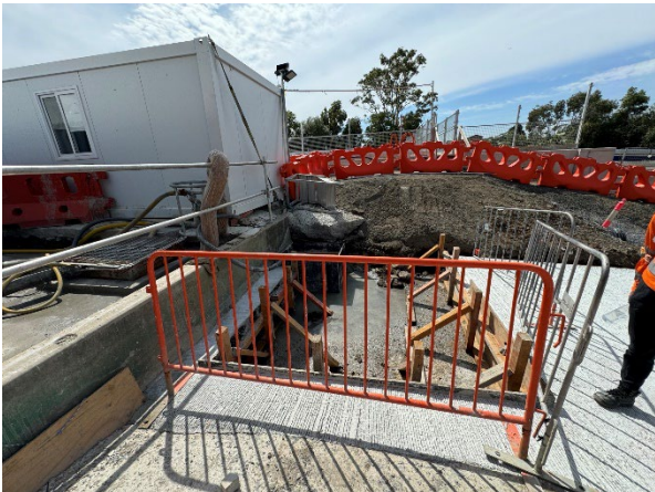
Figure 2.11 – Clyde Dive Site: Washdown sump for grout pump under construction.
