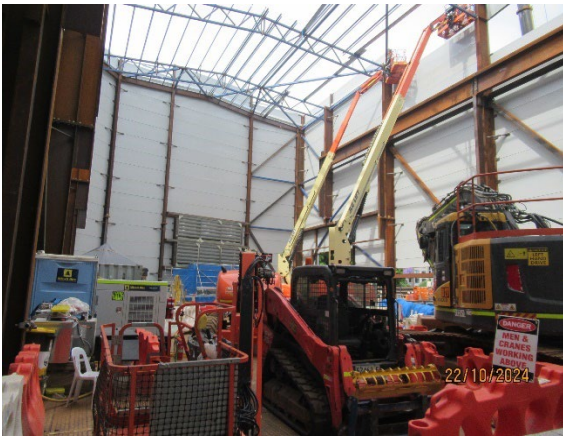
Figure 3.3 Pyrmont West: Construction of the acoustic shed.
