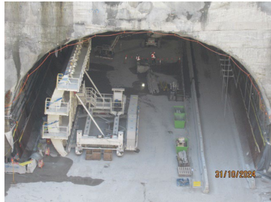
Figure 1.2 Concrete pour for the invert of the Central Cavern (Five Dock).
