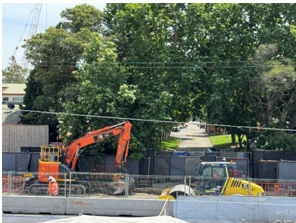
Figure 2.13 –Unwin Street Road works underway.
