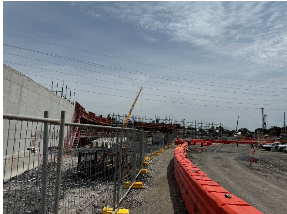
Figure 2.14 – Clyde MSF East Site: Retaining wall construction and backfill ongoing.
