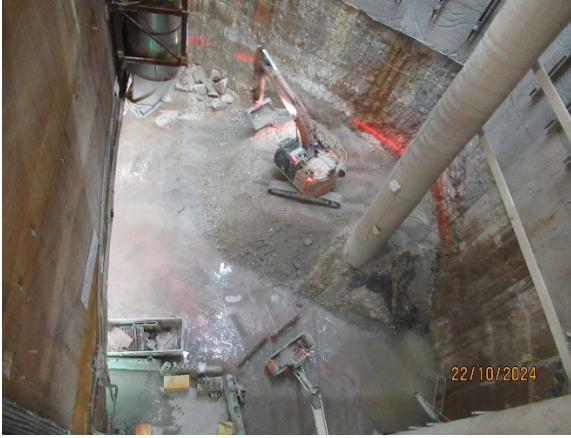
Figure 3.1 Pyrmont East: Base of the shaft-cavern excavation by roadheaders.
