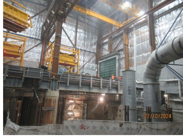
Figure 3.2 Pyrmont East: Inside the acoustic shed showing kibbles and gantry crane.
