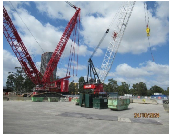
Figure 1.8 Tower crane and crawler crane in operation (SOP).
