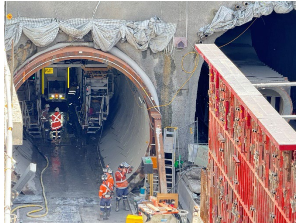
Figure 2.10 –Clyde Dive: Lining Erection Machine (LEM) works ongoing.
