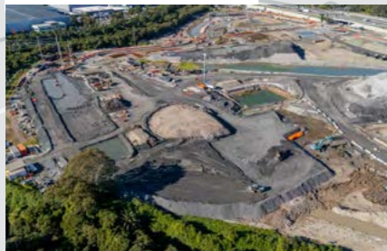
Clyde Stabling Maintenance Facility
