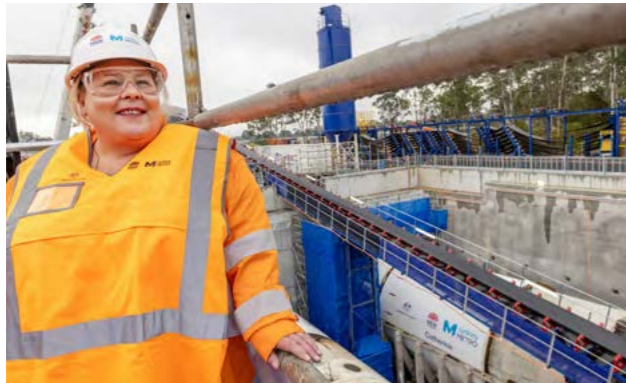
Image: Catherine White at TBM launch at Orchard Hills.
