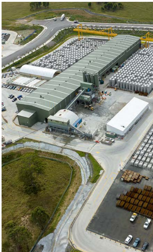
Image: Sydney Metro's precast segment manufacturing plant at Eastern Creek.
