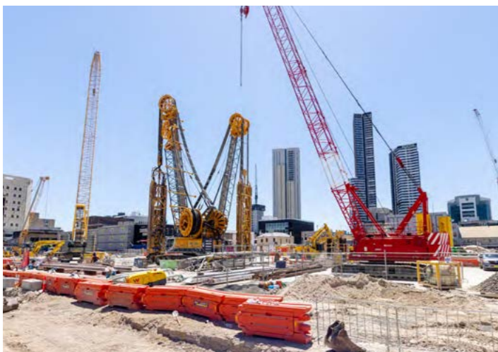
Image: Excavation work at Parramatta.
