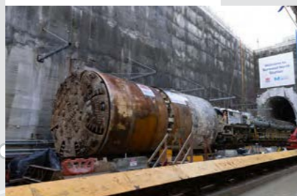
Burwood North Station
