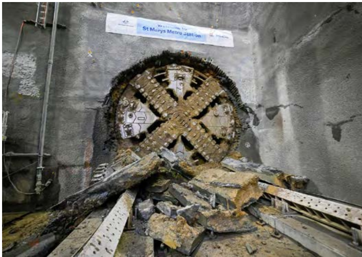
Image: TBM Marlene's final breakthrough at St Marys Station.
