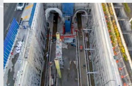
North Strathfield Station
