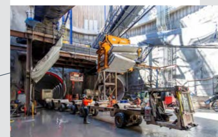
Airport Business Park Station
