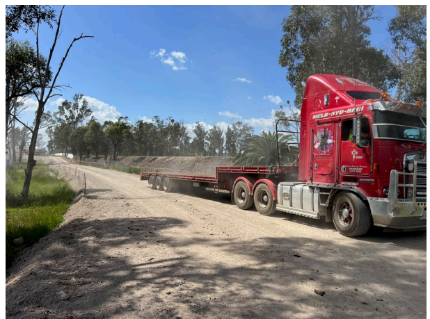
Bringelly – The internal haul roads were dusty during the inspection, ER requested water carts to be available as required to manage the dust levels
