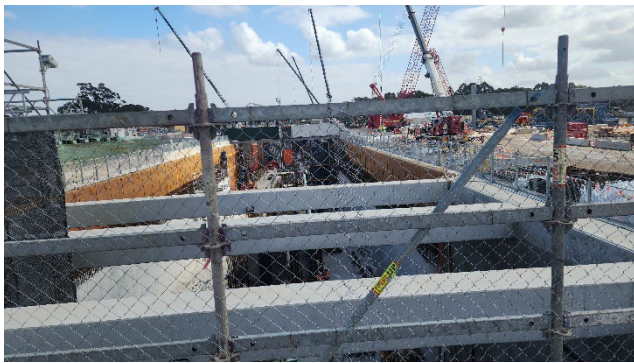
OHE -Water proofing and concrete pours in the box continued
