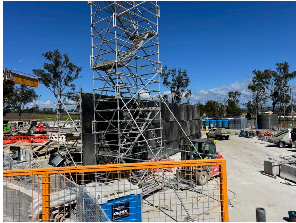
Bringelly – The noise wall remains in place to accommodate OOHW pours
