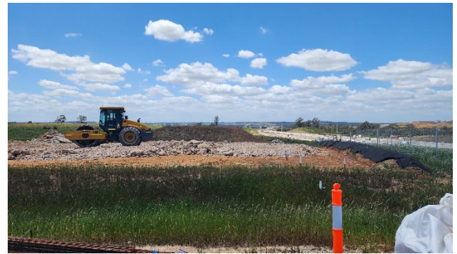
Portion 3 – ERSED bunds installed, preparation for laydown continued
