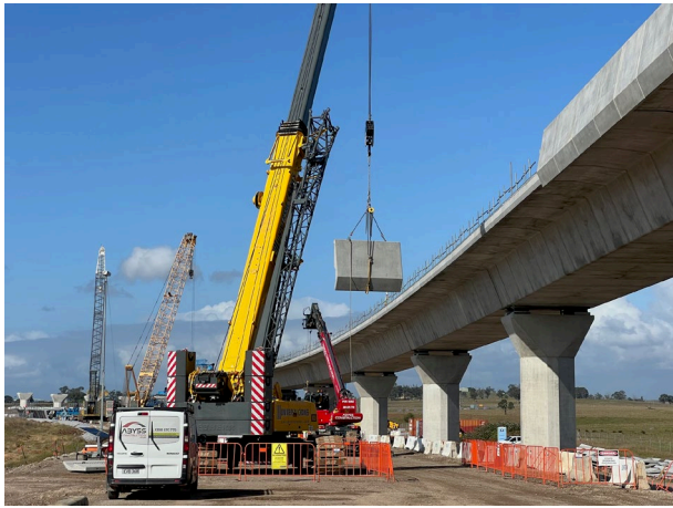
Luddenham North – Parapets being lifted onto the viaduct
