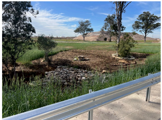
Blaxlands Creek - Rehabilitation of Blaxlands Creek has been successful
