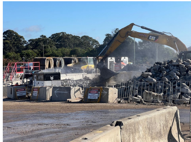
Claremont Meadows – Water cannons were in operation during waste concrete loadout
