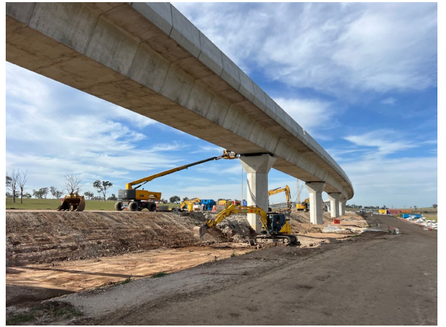
Luddenham North - Viaduct works continue in a southwards direction
