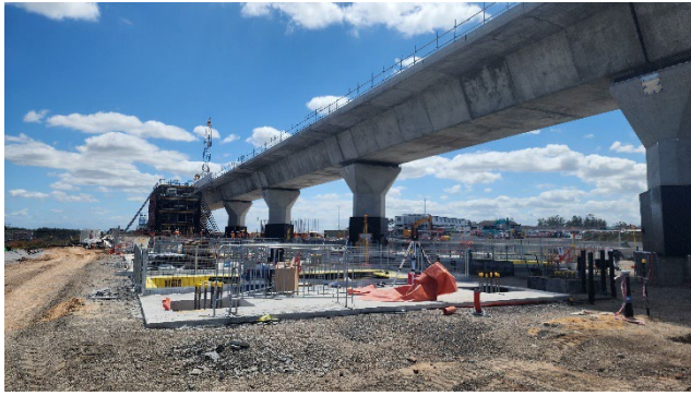
LUD – Lift shaft construction and FRP continued
