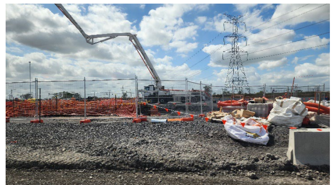
ORH – Form-Reo-Pour (FRP) continued for the substation
