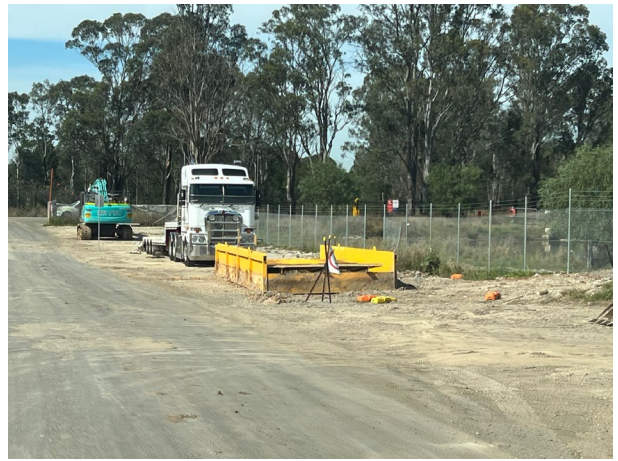
Patons Lane - Two wheel washed were removed, one at Patons Lane, the other at Lansdowne Rd
