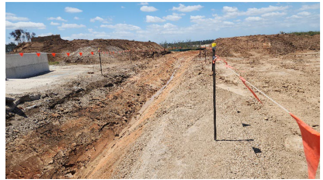
BFD – redirection of clean water swale under construction
