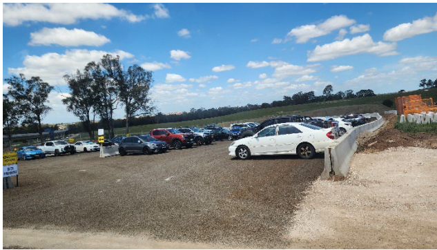
Portion 3 – Car park had been chip-sealed
