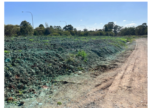
Orchard Hills – The remaining topsoil has been sprayed with polymer
