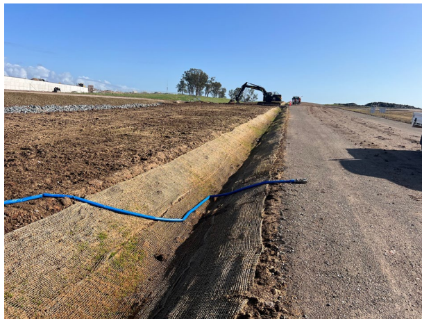
M12 Bridge - Works progress on the permanent drainage lines
