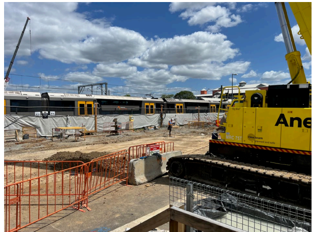
Compound - Piling works progressed without incident in the compound
