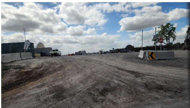
SMF – Laydown areas were maintained
