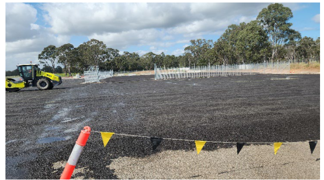
OHE – sealing contractor overflow carpark
