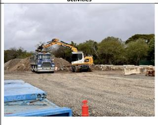
Figure 4: Belmore Triangle – Concrete waste loadout in progress
