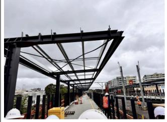
Figure 1: Bankstown Station – platform works including canopy and platform screen doors in progress
