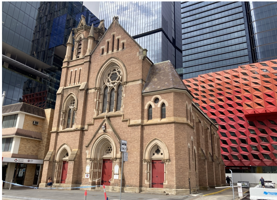
Figure 9: View to north and west elevation of Leigh Memorial Church showing narrow leadlight windows and timber doors which are demonstrative of the inward focus of the Church in terms of views.
