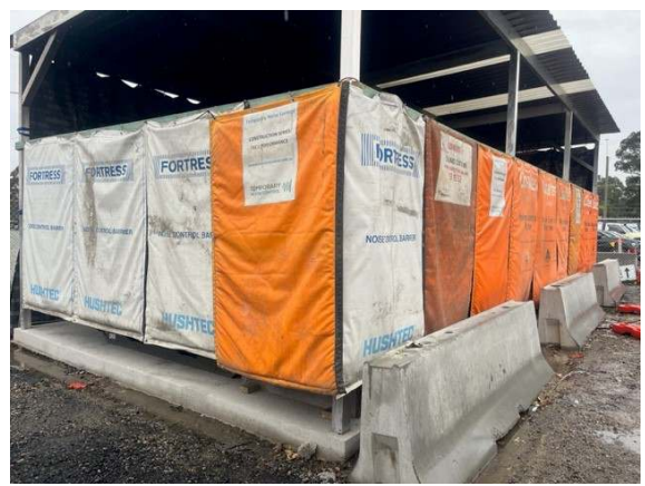
Photos 18 & 19: Generator relocation underway after identified non-compliance with NMLs
