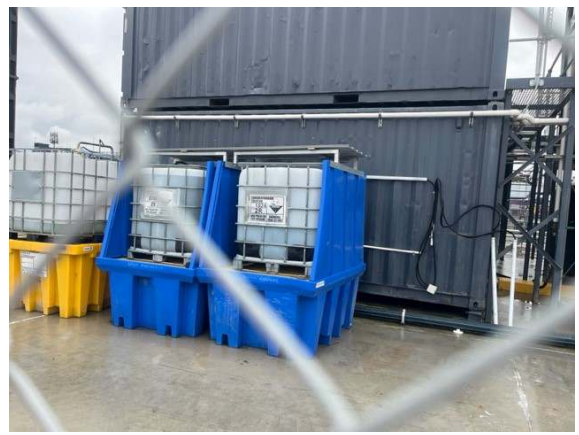
Photos 5 & 6: St Mary's Water Treatment Plant (WTP) with bundled IBCs of treatment chemicals. Discharge from the WTP is to sewer under a Trade Waste Agreement (TWA) with Sydney Water. The CEMP and relevant Sub-plans have been recommended for update to identify the TWA and relevant conditions for implementation, including water quality monitoring.
