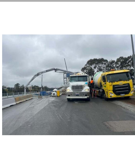
Photo 12: A concrete pour to the station box was underway
