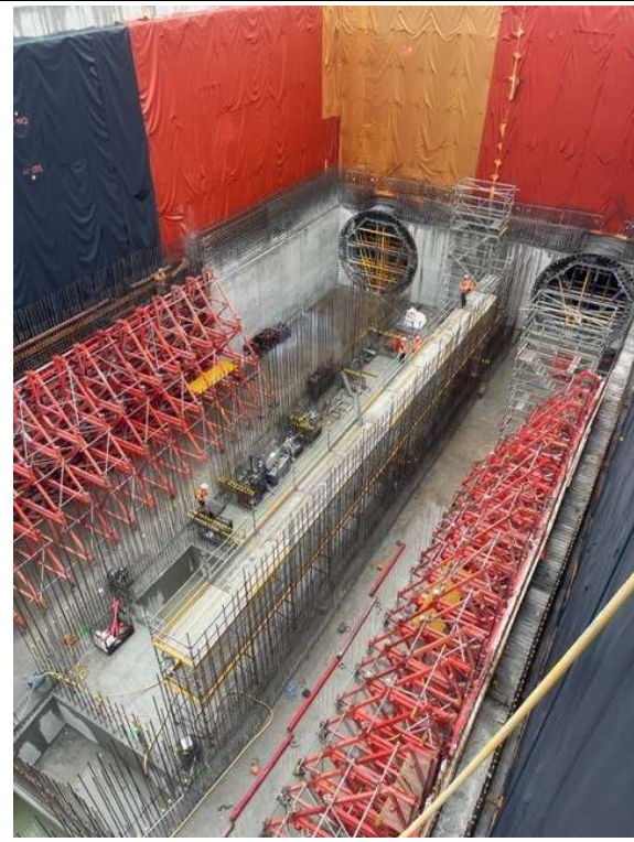
Photos 10 & 11: Form Reo Pour (FRP) and waterproofing were underway inside the station box. Dewatering from sumps to the WTP. Groundwater monitoring remained the responsibility of the SBT contractor at the time of the audit and the SSTOM Groundwater Monitoring Program was undergoing review.
