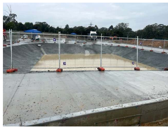
Photo 23: Boral concrete batching plant sediment basin – Water for reuse
