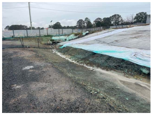
Photos 16 & 17: Polymer application and geofabric observed on batters to reduce dust and erosion risk
