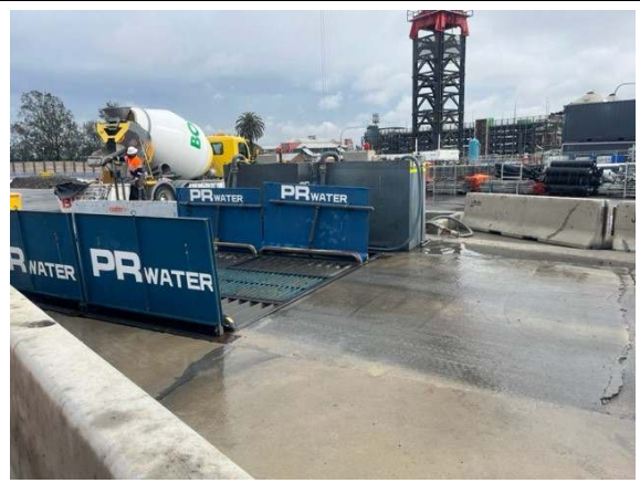
Photos 14 & 15: Wheel wash in place on hardstand site access, utilising recycled water. No tracking or sediment build-up observed.
