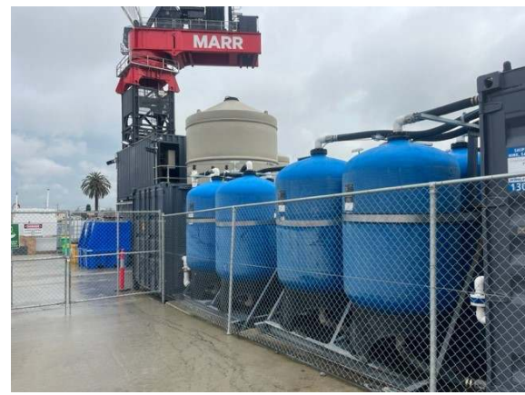
Photos 5 & 6: St Mary's Water Treatment Plant (WTP) with bundled IBCs of treatment chemicals. Discharge from the WTP is to sewer under a Trade Waste Agreement (TWA) with Sydney Water. The CEMP and relevant Sub-plans have been recommended for update to identify the TWA and relevant conditions for implementation, including water quality monitoring.
