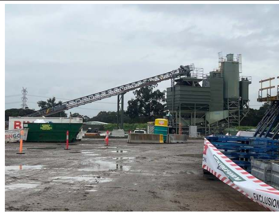
Photo 21: The Boral concrete batching plant remained under Construction
