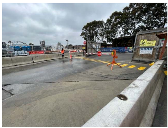
Photos 14 & 15: Wheel wash in place on hardstand site access, utilising recycled water. No tracking or sediment build-up observed.
