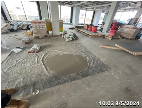
Photo 15 Concrete Mat was used.
