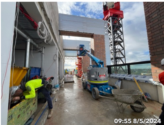
Photo 3 Works at Level 9
