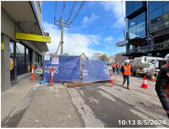
Photo 27 Crows Nest ISD Works - works was delineated and sediment controls implemented.
