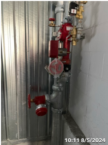
Photo 23 Fire Hydrant Installed
