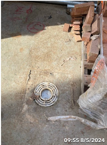
Photo 4 Building internal drains were Installed with waste trap
