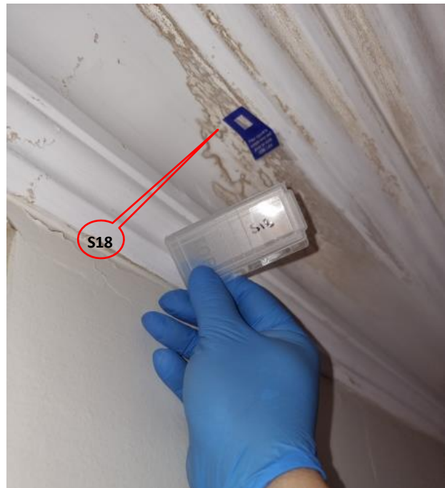
Photograph A.18: Level 1, Room 7 North
