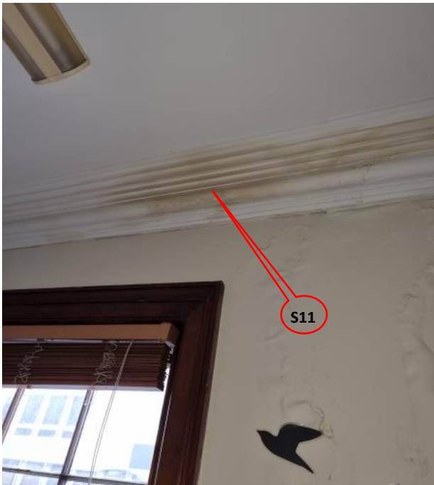
Photograph A.11: Level 1, Room 1, Sample S-11
