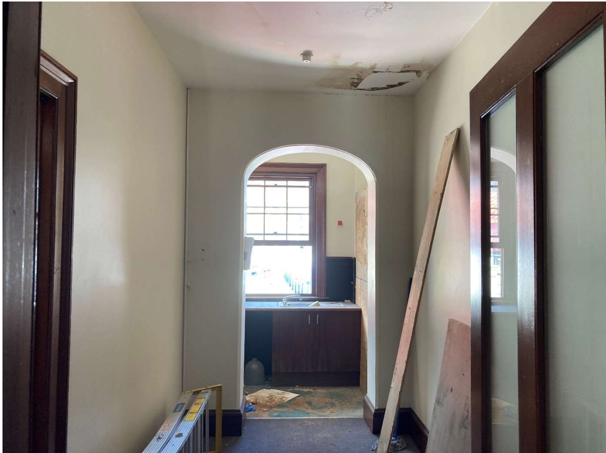
Figure 4-11: General view of first floor hallway looking to kitchenette at rear.
