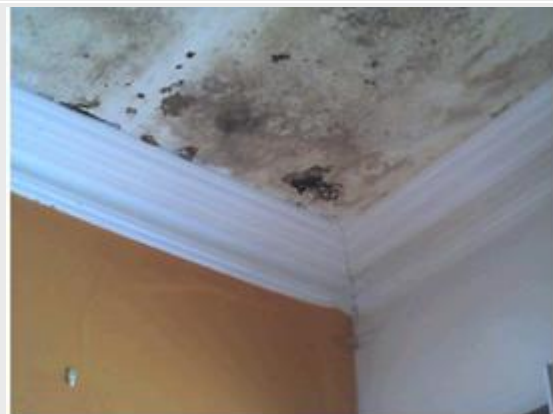
Dark blue shades indicate possible damp wall surface on corner cornice and the west wall
