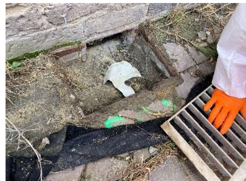
Figure 4-18: Horizontal grated pit adjacent to sub-floor wall vent.
