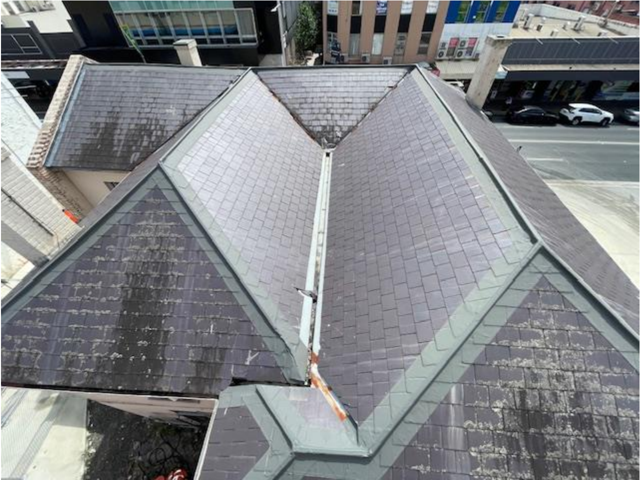
Figure 2: Main slate roof
