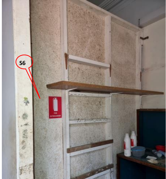
Photograph A.6: Shop 45, Sample S-6
