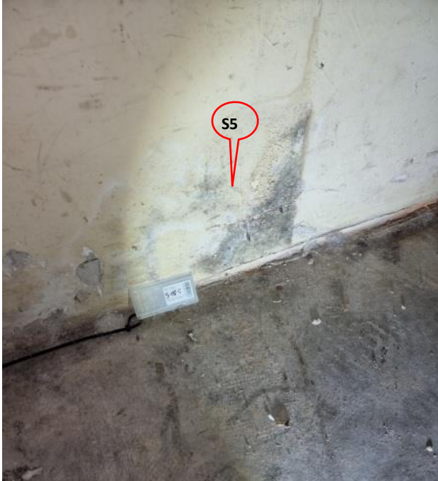
Photograph A.5: Shop 47 Sample S-5
