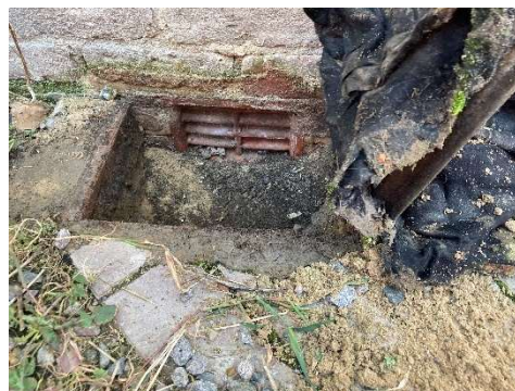
Figure 4-19: Detail view of sub-floor vent and relationship to external ground level.
