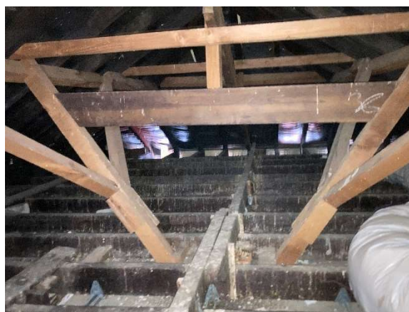
Figure 4-25: Roof structure viewed from within the manhole.
