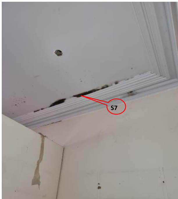
Photograph A.7: Shop 45, Sample S-7
