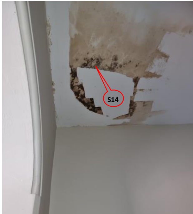
Photograph A.14: Level 1, Room 3, Sample S-14
