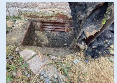
Existing sub floor wall vent; positioned below ground level
