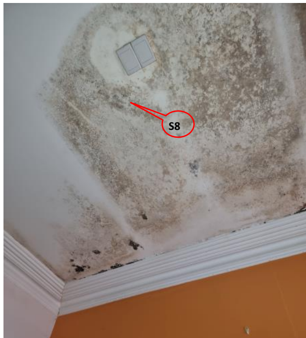
Photograph A.8: Shop 43, Sample S8
