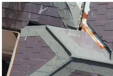
Figure 4-8: Synthetic flashing applied as a temporary measure to roof ridges.
