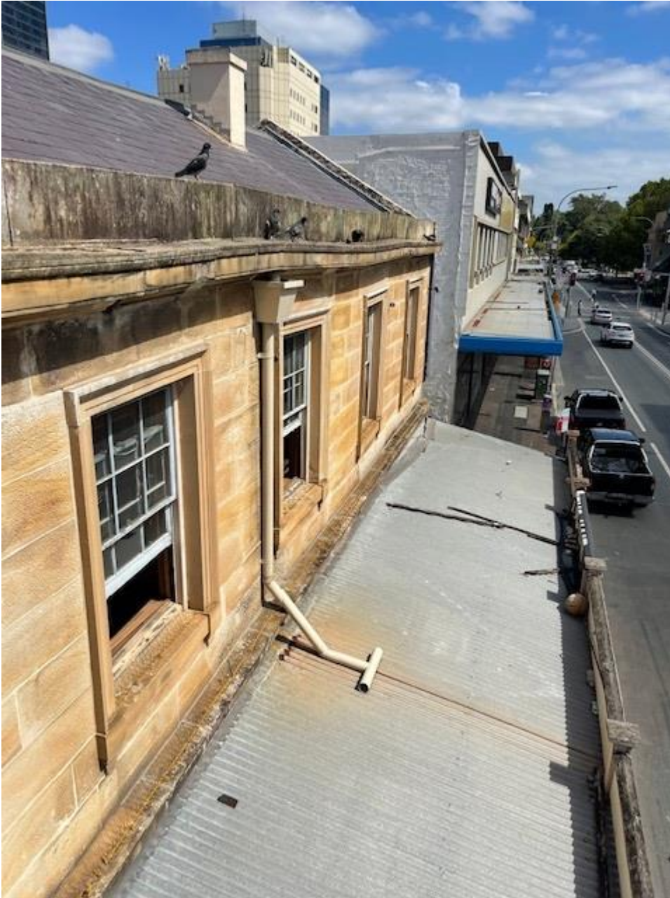
Figure 4: Front street awning metal roof
