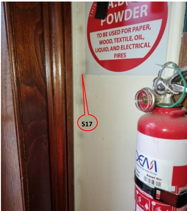
Photograph A.17: Level 1, Room 5
