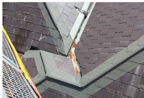
Figure 4-14: Middle box gutter and reconfigured roof structure.
