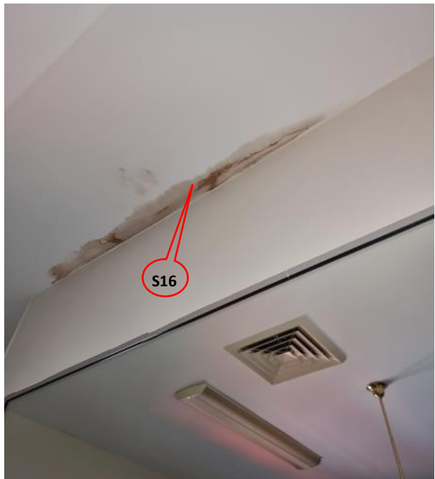
Photograph A.16: Level 1, Room 4, Sample S-16
