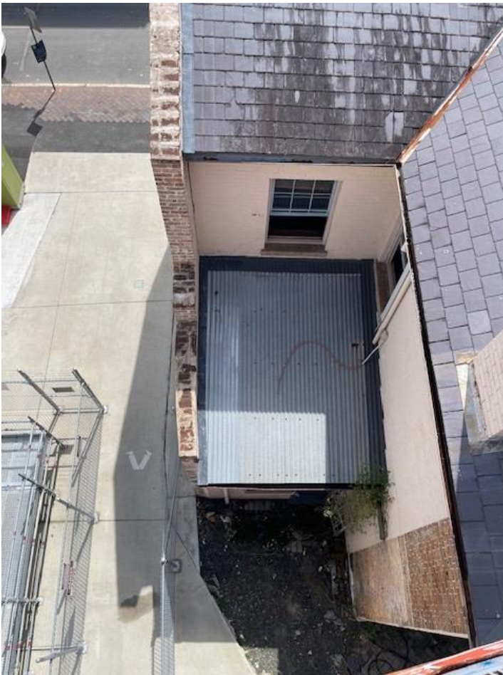
Figure 5: Lower South metal roof sheeting
