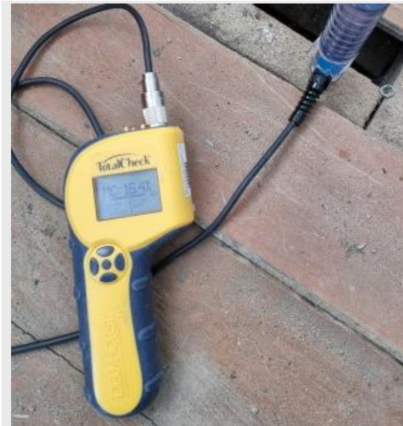
Shop 47 floor joist, 16.4% indicate at risk for mould growth
