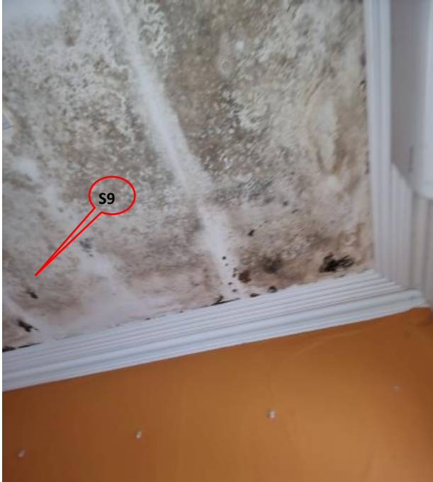
Photograph A.9: Shop 43 Sample S-9
