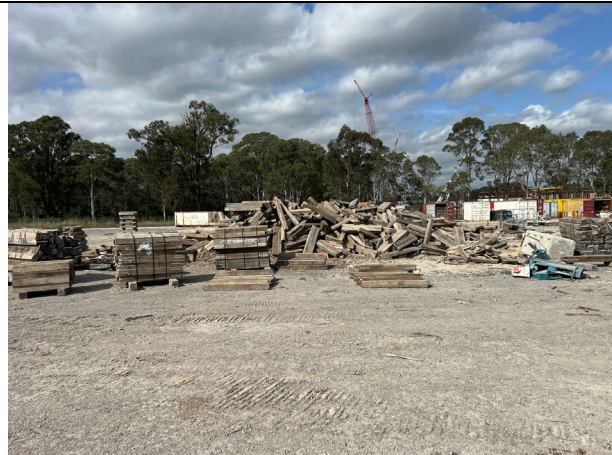
Orchard Hills – Scrap hardwood timber is stockpiled and provided to a timber recycler.
