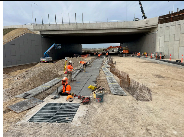
M12 Bridge – Drainage works are progressing underneath the bridge.
