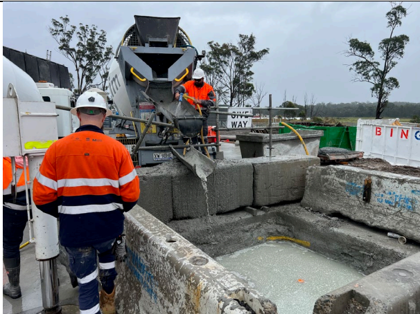
Bringelly – The concrete washout pit was effectively used during the inspection.
