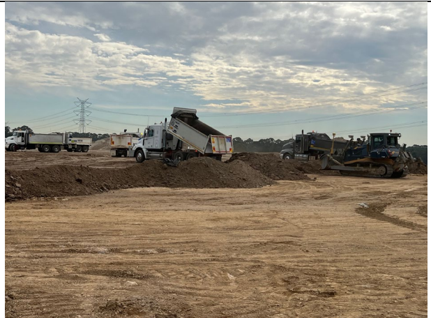
PS105 - Loading of geotechnically unsuitable material continues.
