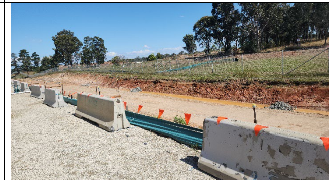
BFD – clean water swale backfilling and smaller swale constructed.
