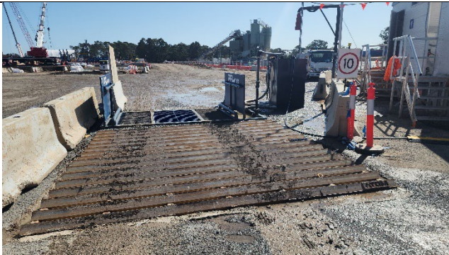
ORH -Wheel wash installed.
