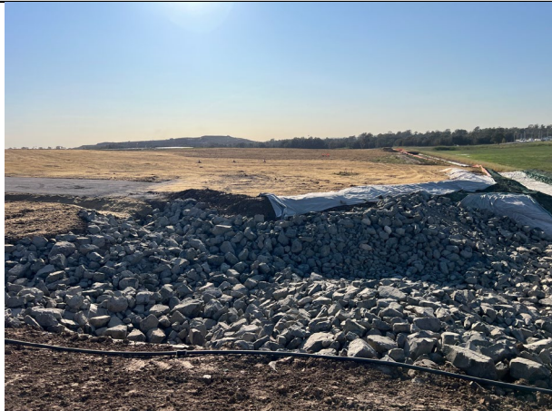
M12 Bridge - A significant portion of the catchment has been hydromulched.
