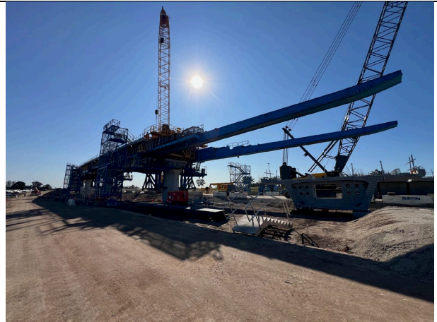
Luddenham North - Works continue on the viaduct.
