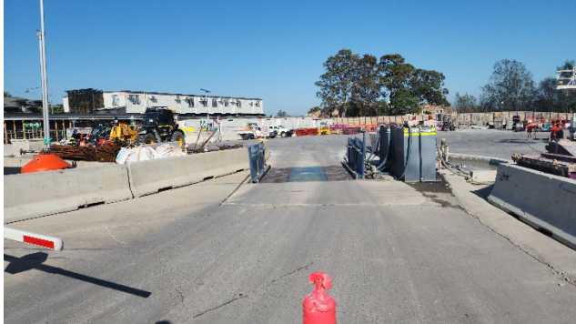
STM – Site exit wheel wash and laydown.
