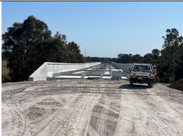
Blaxland's Creek - The bridge over Blaxland's Creek is nearing completion.
