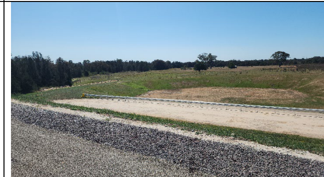
Portion 3 – retention basin noted that PLM will vegetate the basin.
