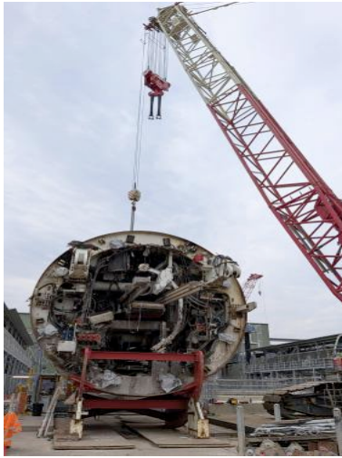
Figure 2.15: Rosehill site: TBM 2 assembly ongoing.
