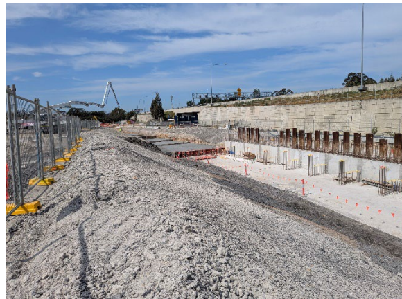
Figure 2.12: Clyde MSF East - Retaining walls and blinding layer concrete pours ongoing.
