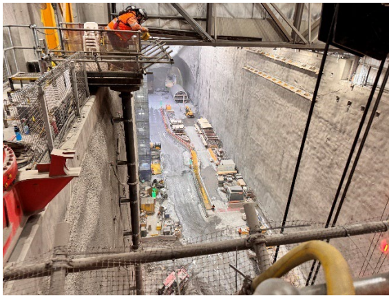
Figure 2.5 -Westmead Site: Station Box activities continuing.
