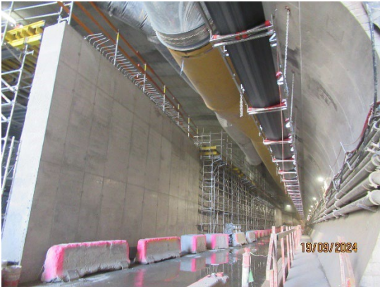
Figure 1.5 Plenum FRP works in the cross over cavern (Burwood North).
