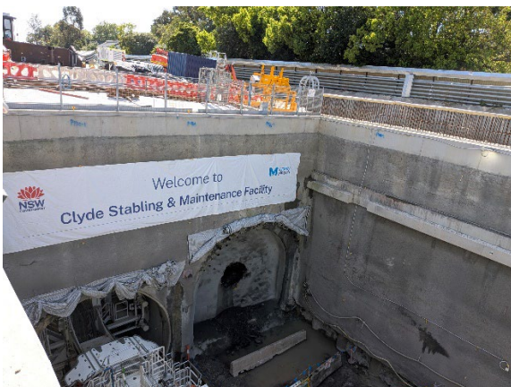
Figure 2.13 – Clyde Dive – LEM Assembly ongoing. Roadheader break through.
