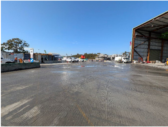
Figure 2.9 – Rosehill Site: Street sweeper mobilised and hardstand areas wet down.
