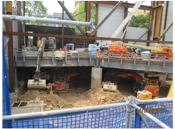
Figure 3.4 Pyrmont West: Excavation under the steel deck using rock hammers.
