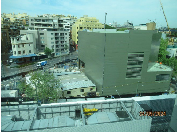
Figure 3.1 Pyrmont East: Plenum roof installed.
