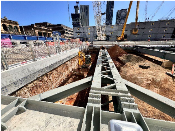
Figure 2.3 – Parramatta Site: Western Station Box excavation continuing.
