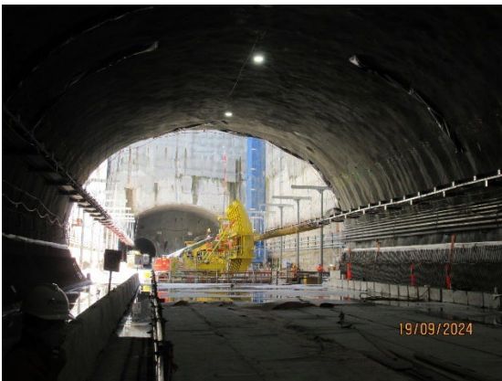
Figure 1.3 Formwork being assembled in the western shaft (Five Dock).
