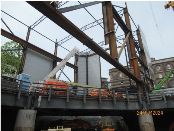
Figure 3.3 Pyrmont West: Construction of the acoustic shed.
