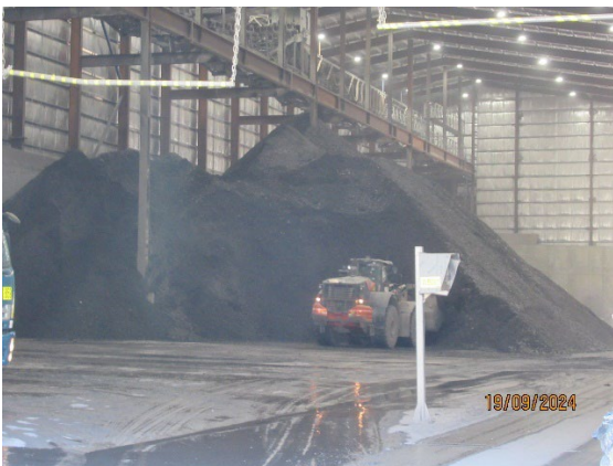
Figure 1.1 Spoil stockpile inside the Spoil Shed (The Bays).
