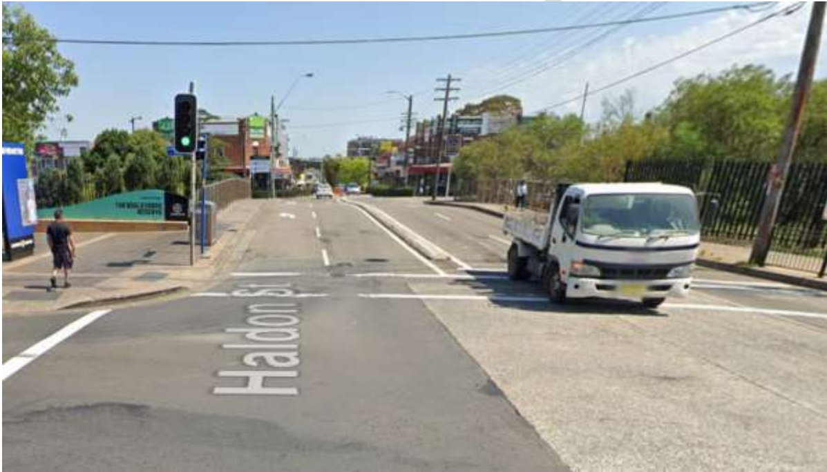
Figure 26: Haldon Street Overbridge (Source: Google Maps)
