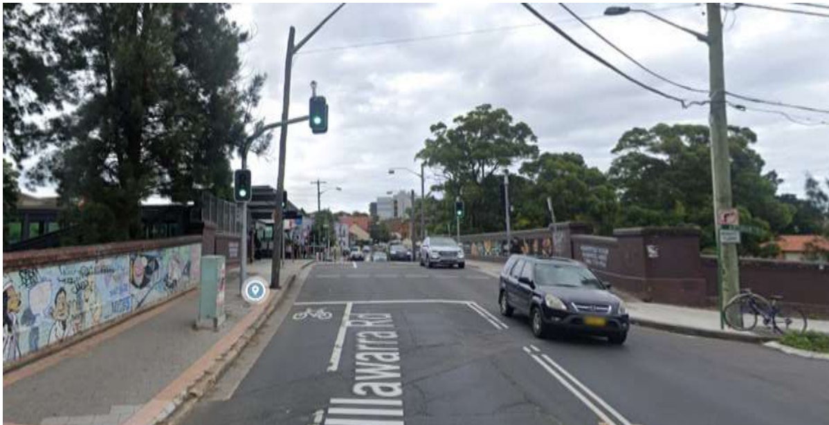
Figure 2: Illawarra Road Overbridge (Source: Google maps)
