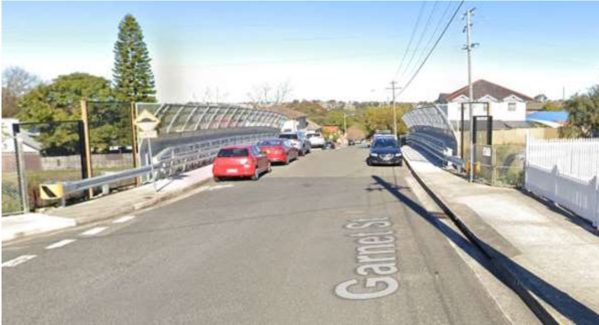
Figure 11: Garnet Street Overbridge (Source: Google Maps)
