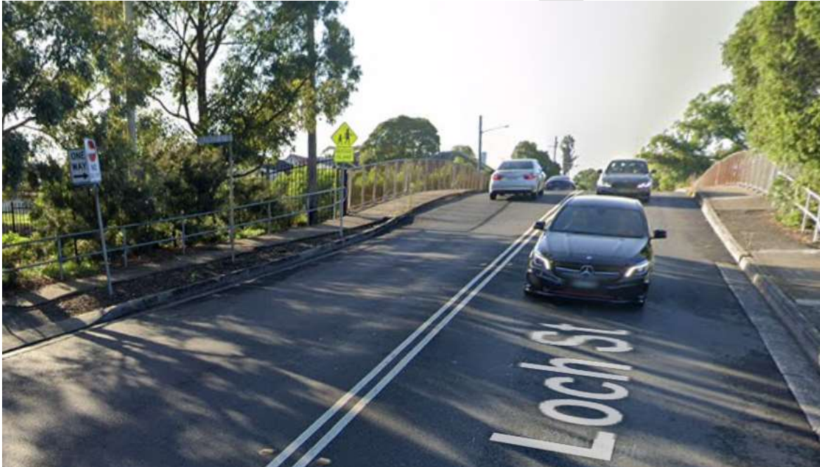
Figure 20: Loch Street Overbridge (Source: Google Maps)
