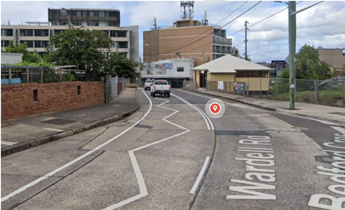
Figure 8: Wardell Road Overbridge (Source: Google Maps)
