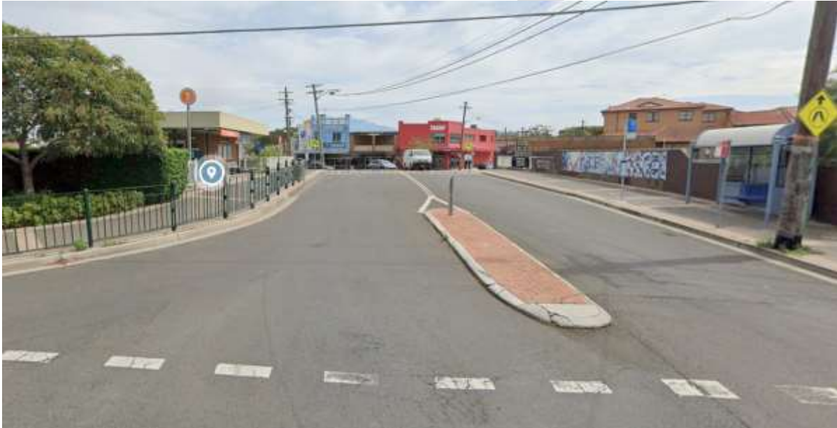
Figure 14: Duntroon Street Overbridge (Source: Google Maps)
