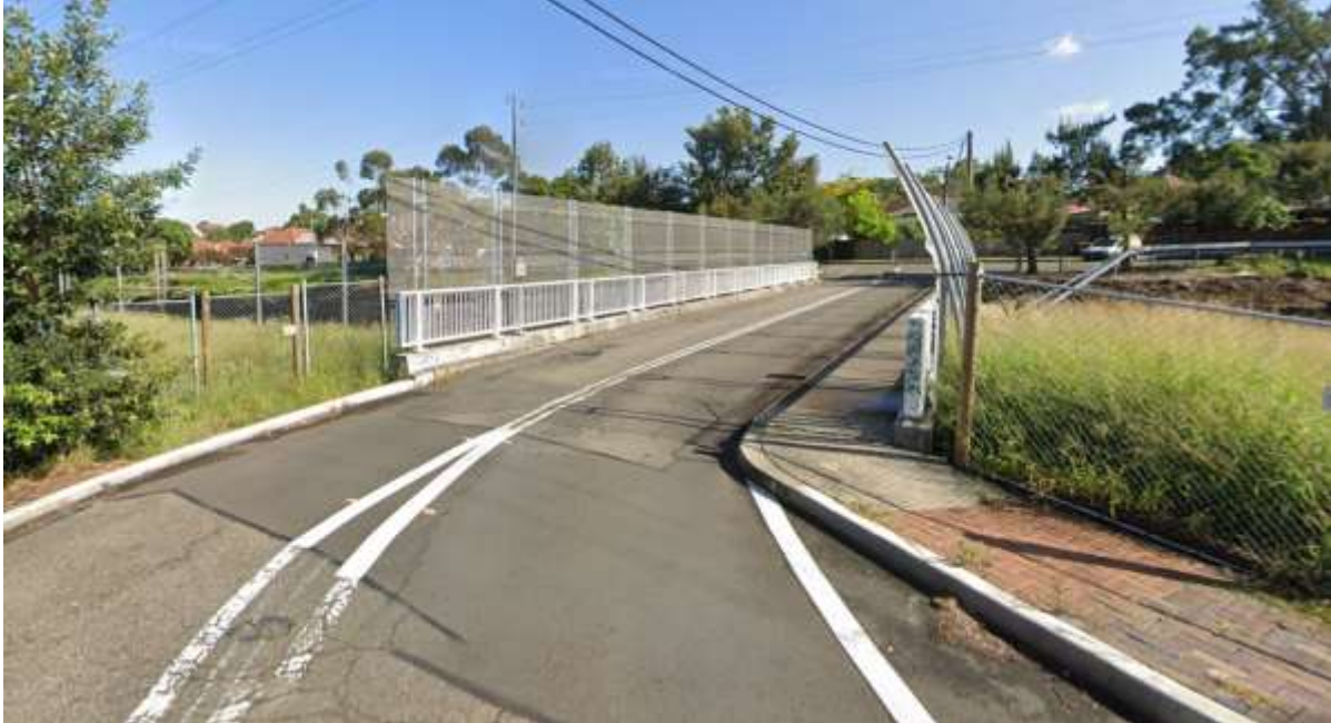
Figure 5: Albermarle Street Overbridge (Source: Google Maps)
