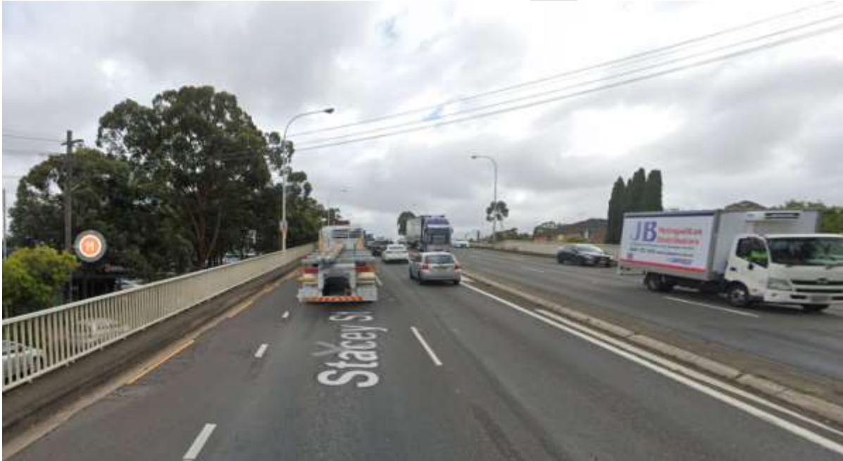
Figure 35: Stacey Street Overbridge (Source: Google Maps)
