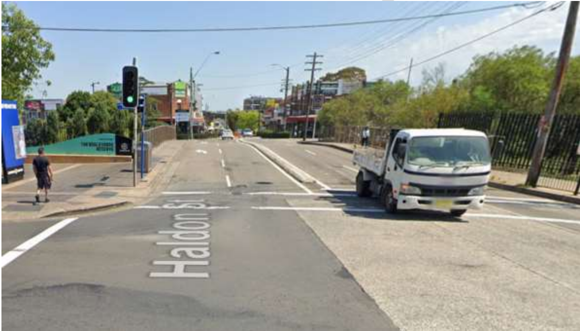
Figure 26: Haldon Street Overbridge (Source: Google Maps)
