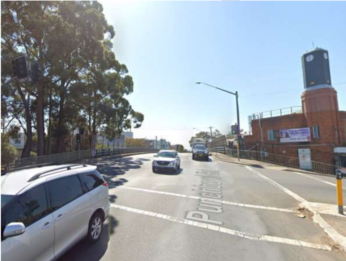
Figure 32: Punchbowl Road overbridge (Source: Google Maps)
