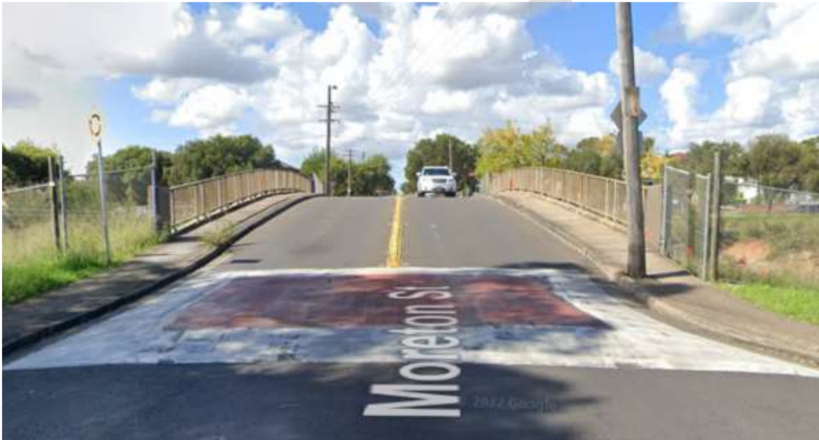
Figure 23: Moreton Street Overbridge (Source: Google Maps)
