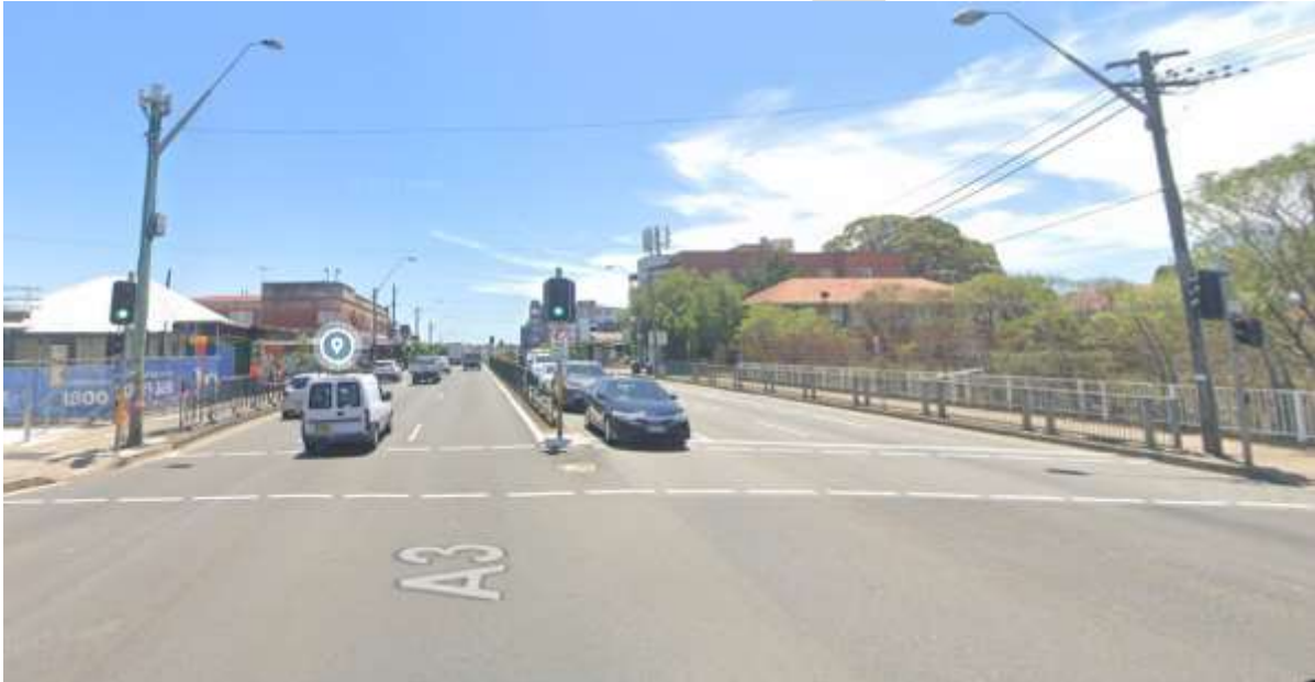
Figure 29: King Georges Road Overbridge (Source: Google Maps)
