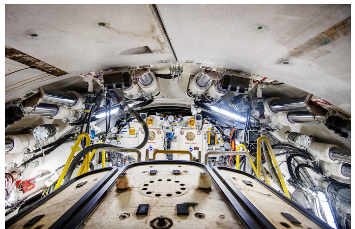
Inside TBM Jessie.
