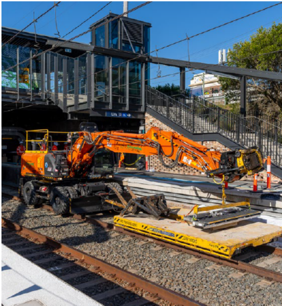
Above: Sydney Metro conversion works at Hurlstone Park
