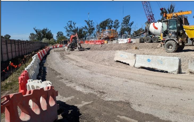
Bringelly – Condition of sealed internal haul roads in good condition.
