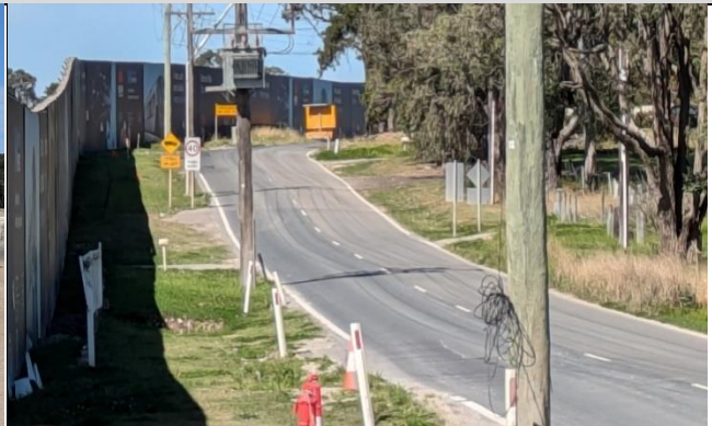
Kent road at site access – Negligible tracking from SBT.
