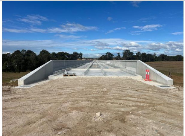
Blaxland's Creek - The bridge north of Blaxland's Creek is nearing completion
