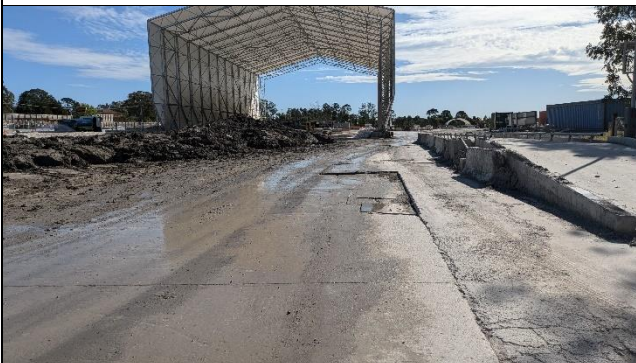
Orchard Hills south view north – Some accumulations noted on haul road from X passage spoil storage area.
