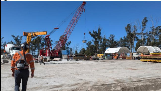
Bringelly view east to shaft – Concrete slab placed over loading/unloading areas.
