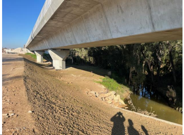
Blaxland's Creek - All disturbed areas within the catchment have now been hydromulched
