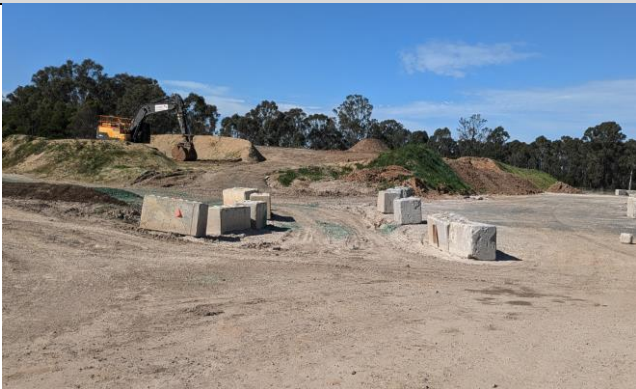
Orchard Hills – Eastern topsoil/spoil stockpile
