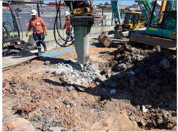
Platform 1/2 - Piles were being broken back on platform 1/2
