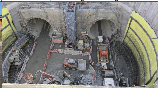
Claremont Meadows – Waterproofing underway in shaft.
