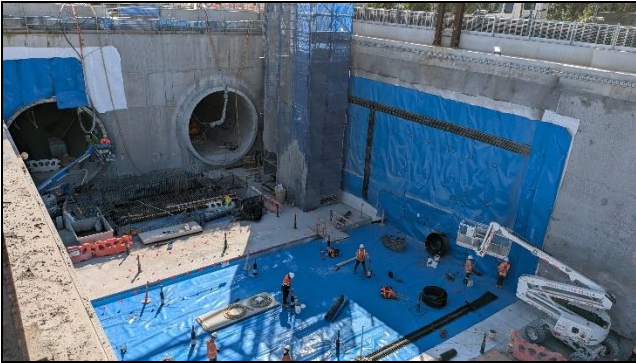
Orchard Hills tunnel portal – Waterproofing.
