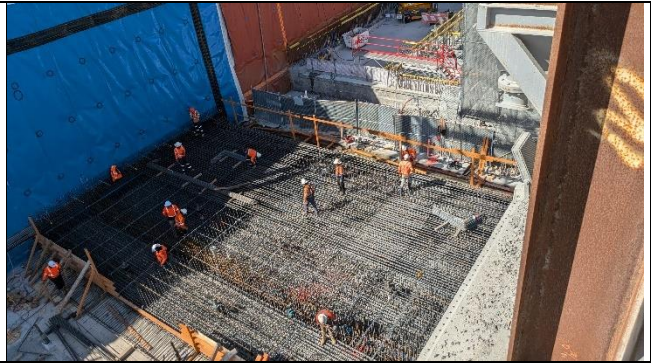
Orchard Hills tunnel portal – FRP for base slab.
