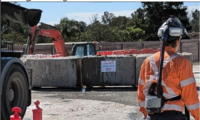
Bringelly view north east, west of shaft – Concrete washout well managed.
