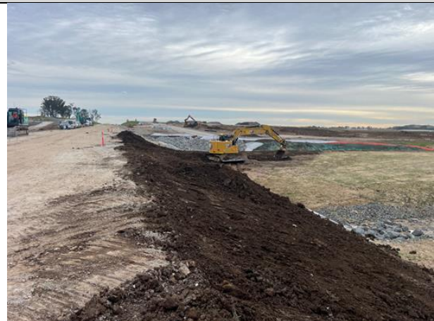
M 12 Bridge - Topsoil is being spread on the batters awaiting hydromulching
