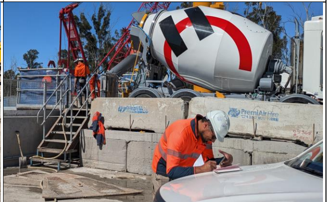
Bringelly – Concrete deliveries to drop pipe west of shaft well managed.
