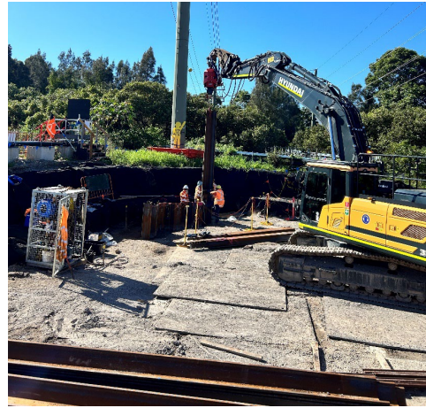
Figure 2.14: Clyde MSF Site – Water main tie in works
