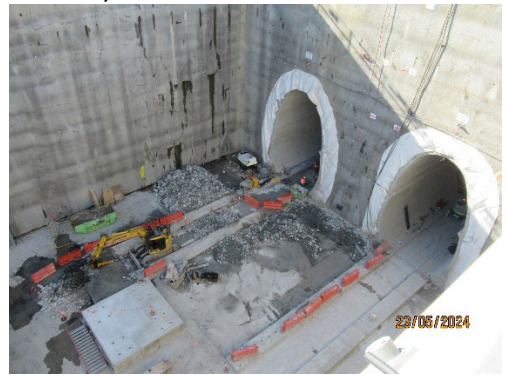
Figure 1.8 Preparation for concrete pour for the Nozzle (SOP).
