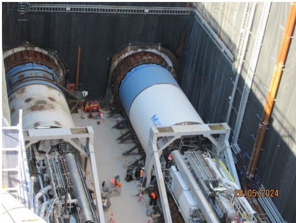
Figure 3.7 The Bays: Assembly of the TBM in the station box
