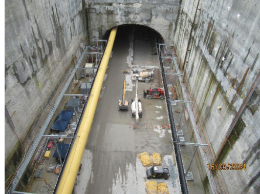
Figure 1 2 TBM supports items visible in the Western Shaft (Five Dock).
