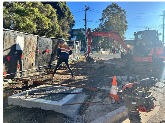
Figure 4.2 Westmead Utility Works: Telstra Pit backfill and footpath reinstatement
