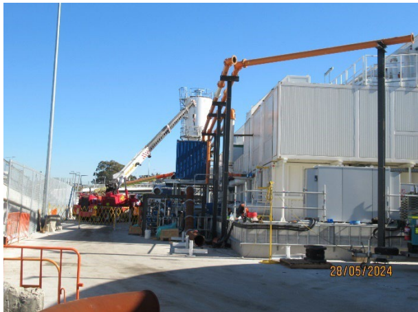
Figure 3.8 The Bays: Assembly of the Slurry Treatment Plant.
