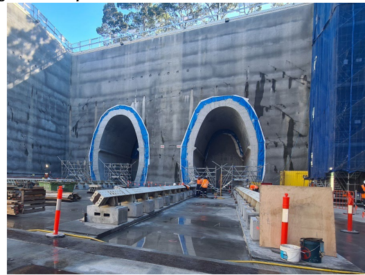
Figure 2.16: SOP Site – tunnel portal with TBM tracks
