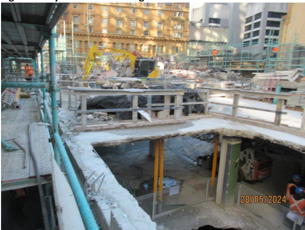
Figure 3.5 Hunter St East: Demolition works ongoing.
