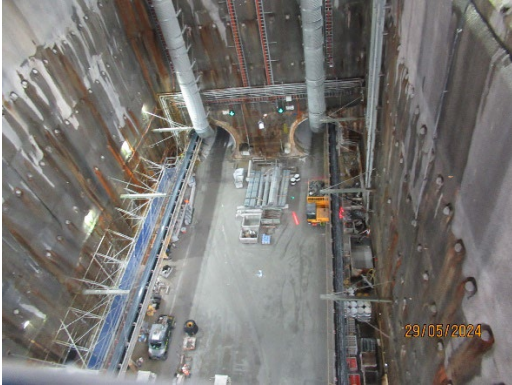
Figure 1 1 Works in the station box (The Bays).
