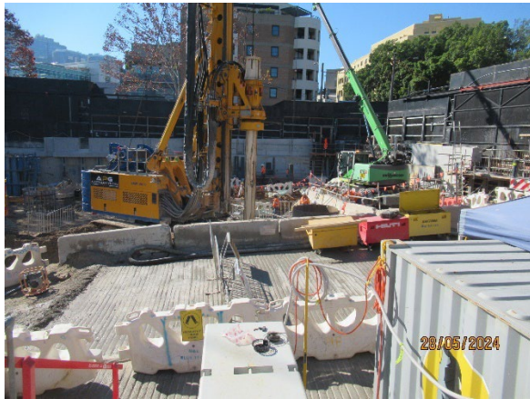
Figure 3.4 Pymont West: Piling pad completed for piling.
