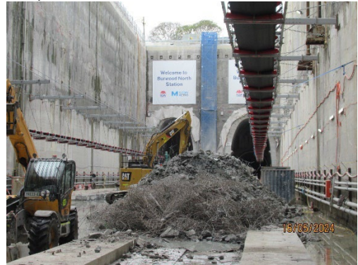
Figure 1 4 Removal of concrete plinths after TBM traverse (Burwood North).
