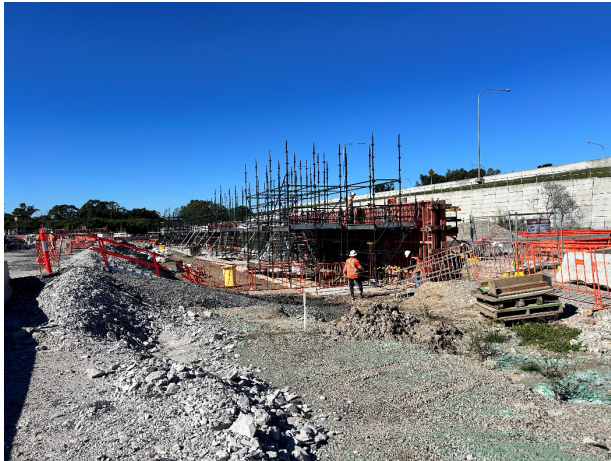
Figure 2.13: Clyde MSF Site – Utilities retaining wall FRP
