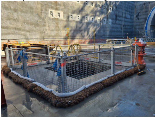
Figure 2.15: SOP Site – station box dewatering sump
