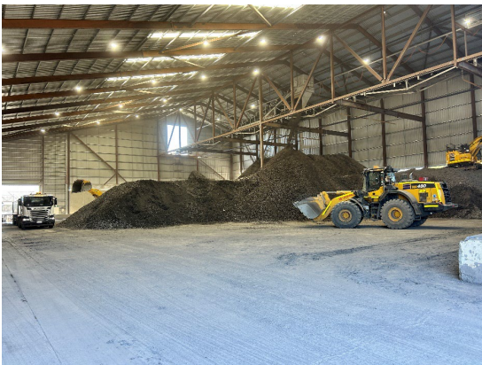
Figure 2.7: Rosehill Site – spoil shed
