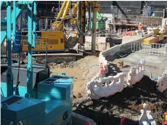
Figure 3.3 Pymont West: Piling works.
