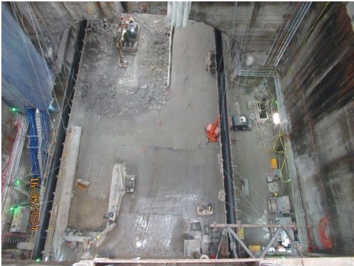
Figure 1 3 Works in the Eastern Shaft (Five Dock).
