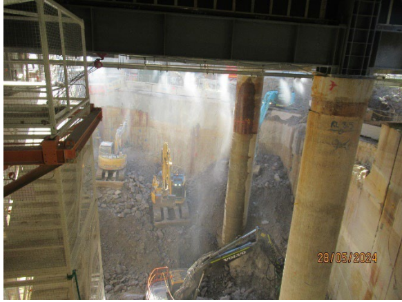
Figure 3.2 Pymont East: Excavation of sandstone using rock hammers under steel deck
