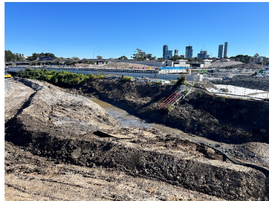
Figure 2.12 – Clyde MSF Site – A'Becketts Creek dewatering
