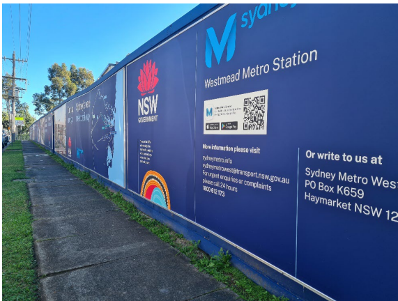
Figure 2.1: Westmead Site –Hoarding with project information
