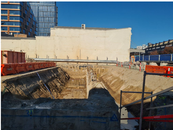
Figure 2.3: Parramatta Site – eastern Station Box excavation
