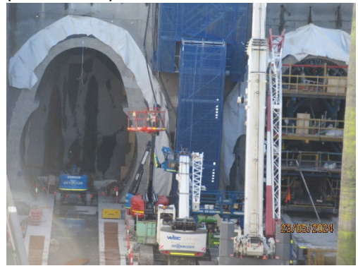
Figure 1 6 Nozzle lining works in the Station Box (North Strathfield).
