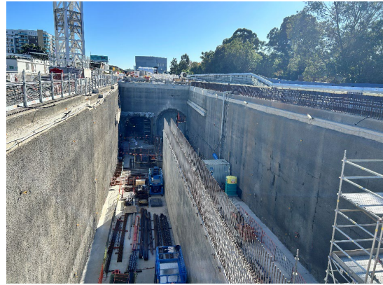
Figure 2.6: Clyde Dive site – Dive base and deflection wall FRP
