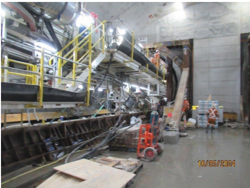
Figure 1 5 TBM 4 being prepared to re-commence tunnelling. (Burwood North).
