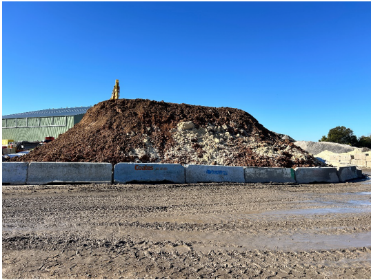
Figure 2.13: Clyde MSF Site – Parramatta ASS stockpile and treatment
