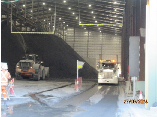
Figure 1 1 Spoil stockpiled in the spoil shed (The Bays).
