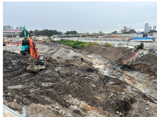
Figure 2.12 – Clyde MSF Site – A'Becketts Creek contaminated spoil removal prior to backfill.
