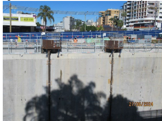
Figure 1 4 Concrete drop chutes installed (Burwood North).
