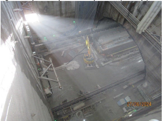
Figure 1 3 Works in the Eastern Shaft (Five Dock).
