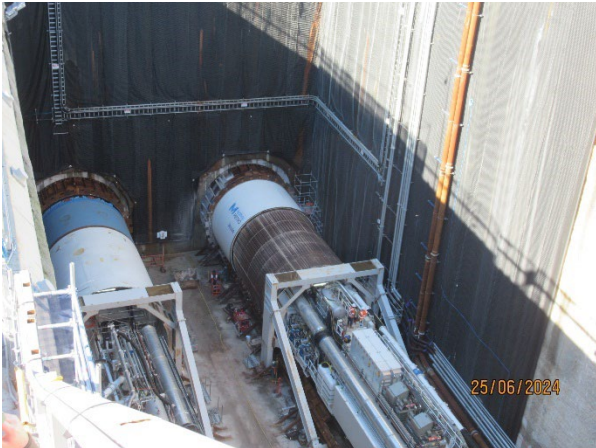
Figure 3.7 The Bays: Commencement of tunnelling of TBM Jessie
