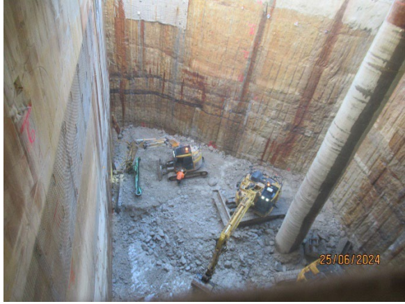
Figure 3.2 Pyrmont East: Excavation of sandstone using rock hammers under steel deck
