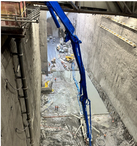
Figure 2.1: Westmead Site – Station Box base slab concrete pour
