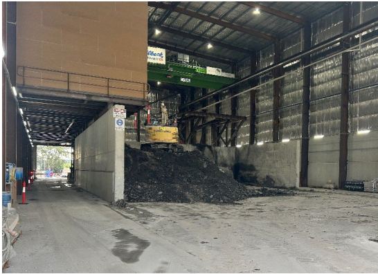
Figure 2.5: Clyde Dive site – Spoil stockpiling and load out from arrival/departure tunnels
