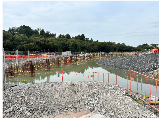
Figure 2.14: Clyde MSF Site – Retaining wall FRH and water storage in excavations
