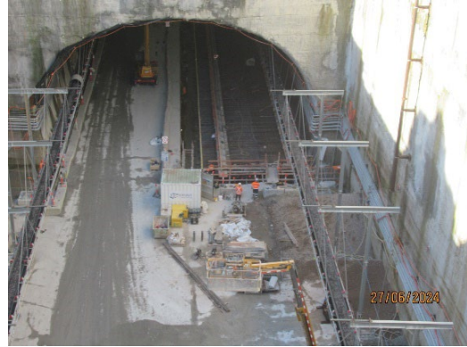
Figure 1 2 FRP for the invert of the Central Cavern (Five Dock).
