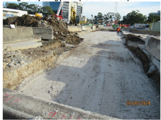
Figure 1.8 Reinstatement of sub-grade after removal of the weighbridge (SOP).
