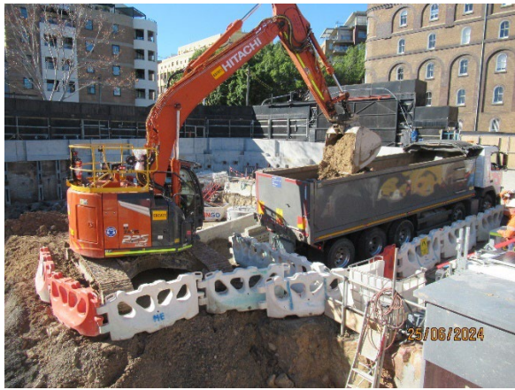
Figure 3.4 Pyrmont West: Piling pad completed for piling.
