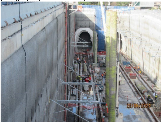
Figure 1.7 Works in the Station Box (North Strathfield)
