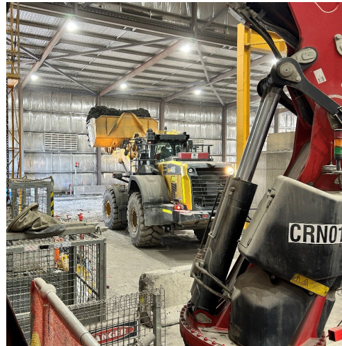
Figure 2.2: Westmead site – Spoil loading inside Acoustic shed
