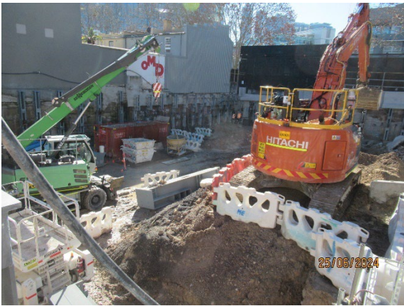
Figure 3.3 Pyrmont West: Piling works.
