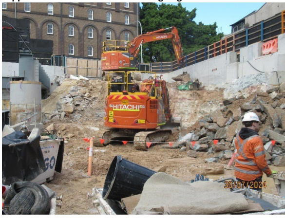
Figure 3.4 Pyrmont West: Excavation of the ramp to PBR using rock hammers.
