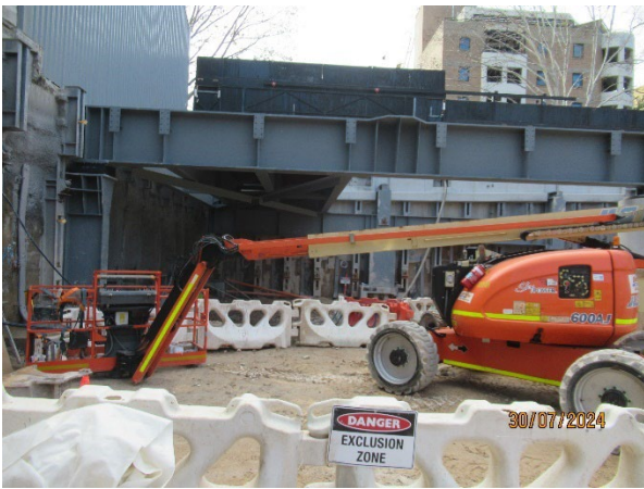
Figure 3.3 Pyrmont West: Installation for the steel deck beams.
