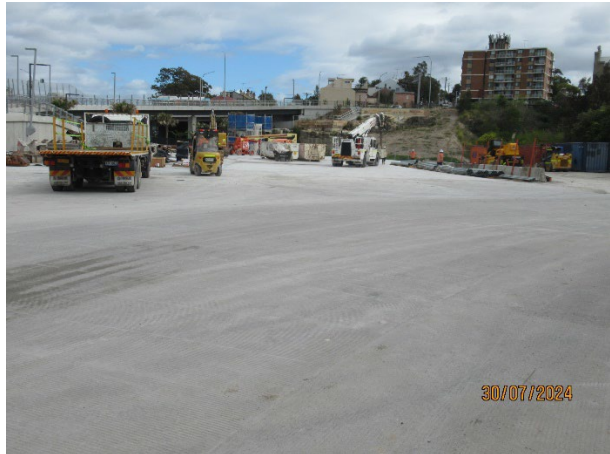
Figure 3.8 The Bays: Works to complete the Truck Marshalling facility.
