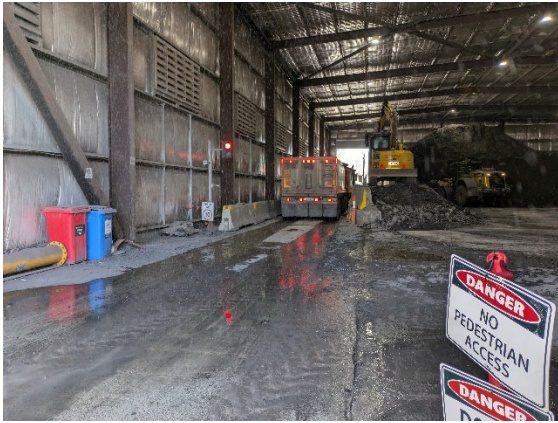
Figure 2.5: Westmead Site: Spoil loading operations within acoustic shed.
