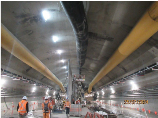
Figure 1.5 Plenum works in the cross over cavern (Burwood North).
