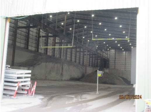
Figure 1.1 Lower volumes of spoil stockpiled in the spoil shed (The Bays).
