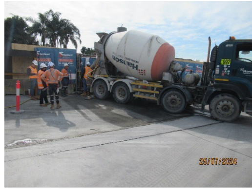
Figure 1.4 Use of concrete drop chutes (Burwood North).
