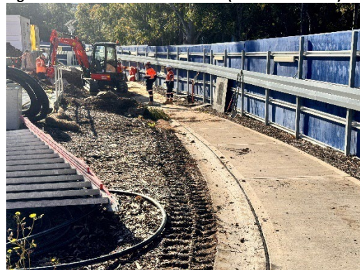
Figure 1.8 Stormwater works to redirect surface water to stormwater (SOP).
