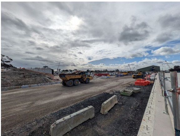
Figure 2.9: Clyde MSF West: Internal haul road completed and operational.
