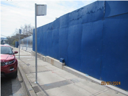
Figure 1.3 Removal of B Class hoarding from East Street (Five Dock).
