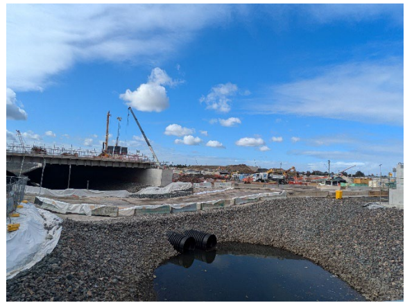
Figure 2.10: Clyde MSF West: Temporary creek crossing completed and operational.
