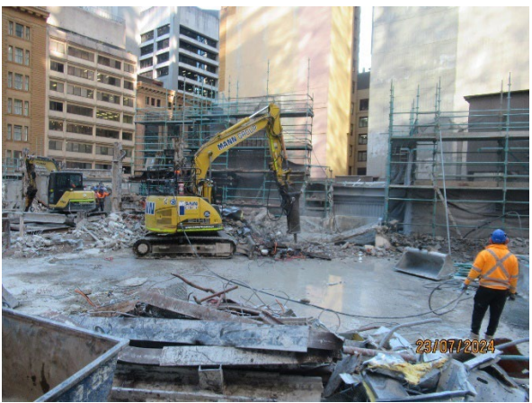
Figure 3.5 Hunter St East: Demolition works ongoing.
