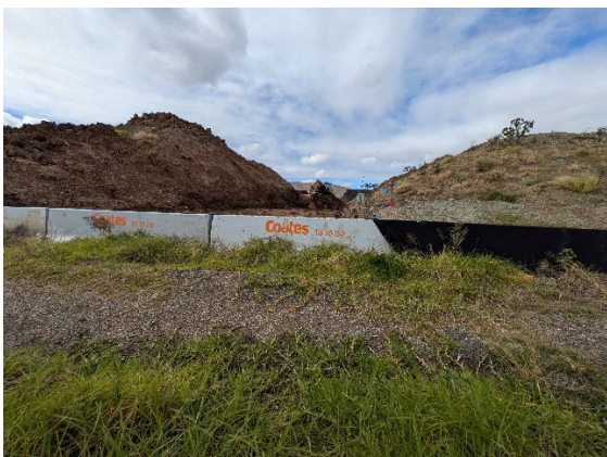
Figure 2.15: Clyde MSF East: Internal haul road works commenced.
