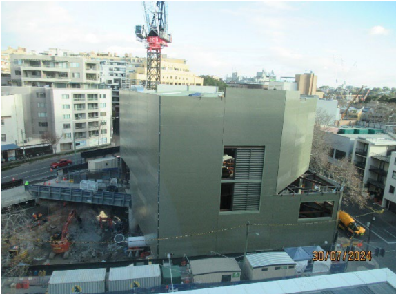
Figure 3.1 Pyrmont East: Ongoing installation of the acoustic shed.
