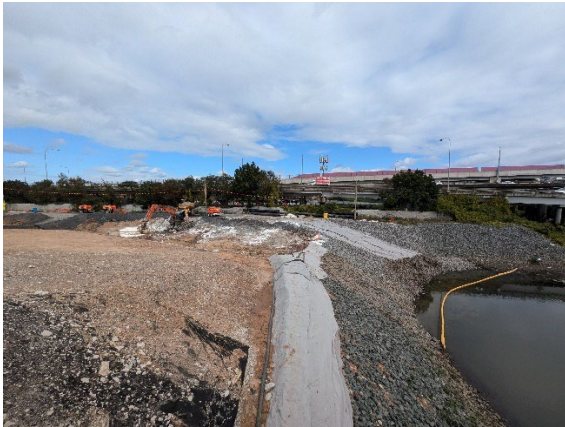
Figure 2.11: Clyde MSF West: Area 1 Swale Drain improvement works commenced.
