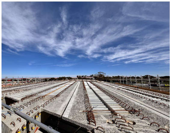
Figure 2.17: Clyde – Unwin St: Girder installation works.
