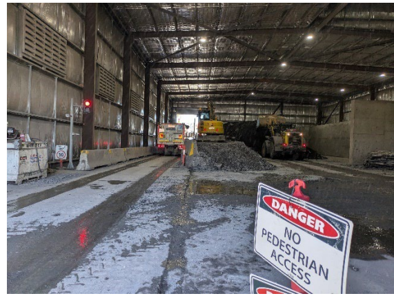
Figure 2.6 – Westmead Site: Spoil loading operations within Acoustic Shed.
