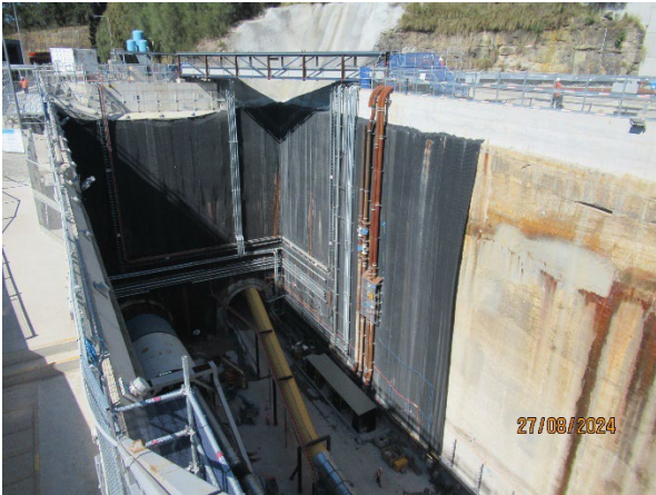
Figure 3.7 The Bays: Ongoing tunnelling of TBM Jessie.
