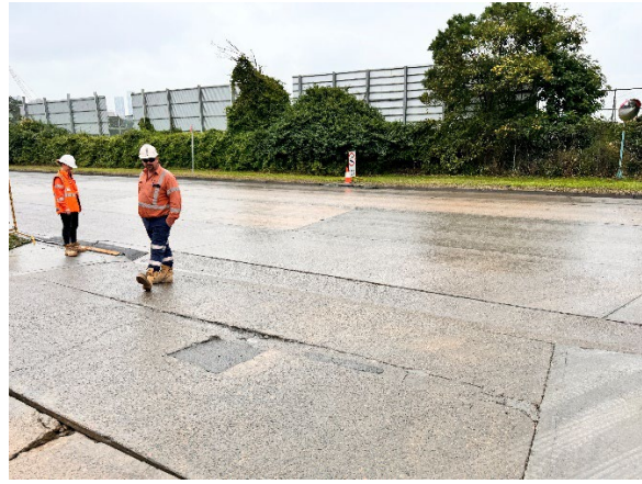
Figure 2.10 – Rosehill Site Gate: No mud tracking observed.
