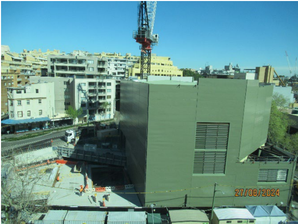
Figure 3.1 Pyrmont East: Near completion of the steel deck and acoustic shed.
