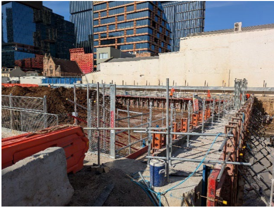
Figure 2.3 - Parramatta Site: Western capping beam poured with formwork being stripped.
