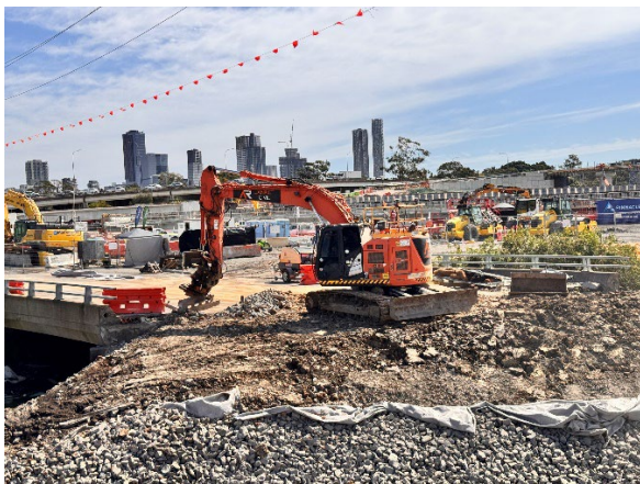
Figure 2.13: Clyde: Kay Street Bridge Demolition works continuing.
