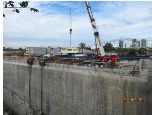
Figure 1.4 Use of concrete drop chutes (Burwood North).
