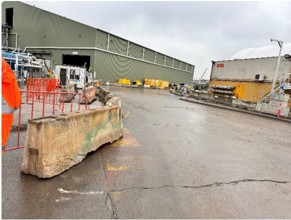
Figure 2.9 - Rosehill Site: Hardstand area observed to be tidy.
