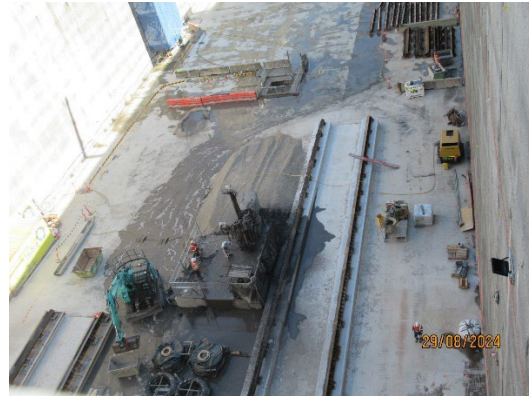
Figure 1.8 Drilling for anchors for the planned tower crane (SOP).
