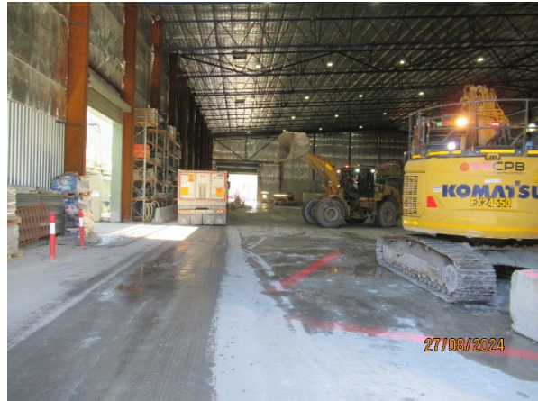
Figure 3.8 The Bays: Load out of spoil from TBM tunnelling.
