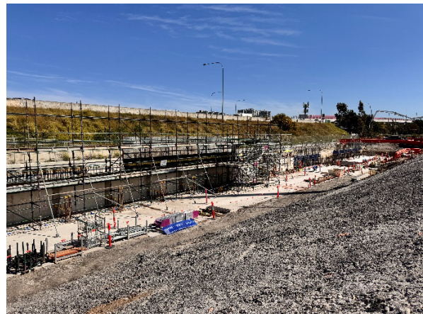
Figure 2.18: Clyde MSF East: Retaining wall works continuing.
