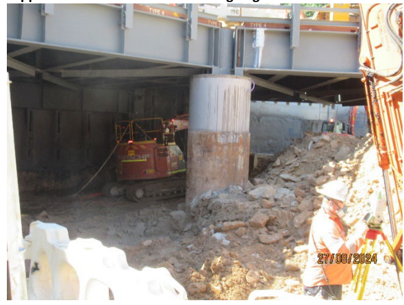
Figure 3.4 Pyrmont West: Excavation using rock hammers.
