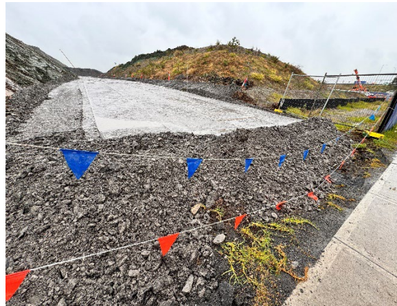
Figure 2.14 - Clyde MSF East: New internal haul road established.
