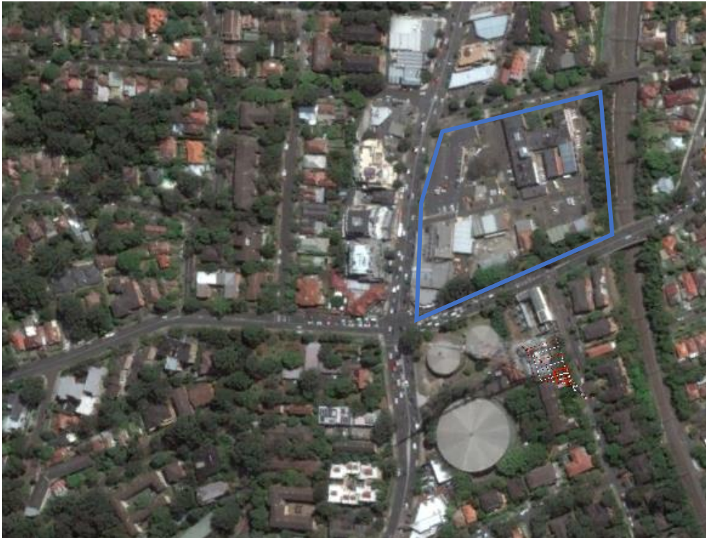
Figure 17 – Aerial Image 2016 prior to works commencing. 55
