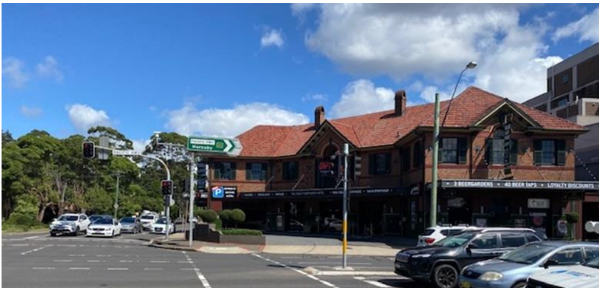
Figure 21 – South and East Elevations of Great Northern Hotel.
