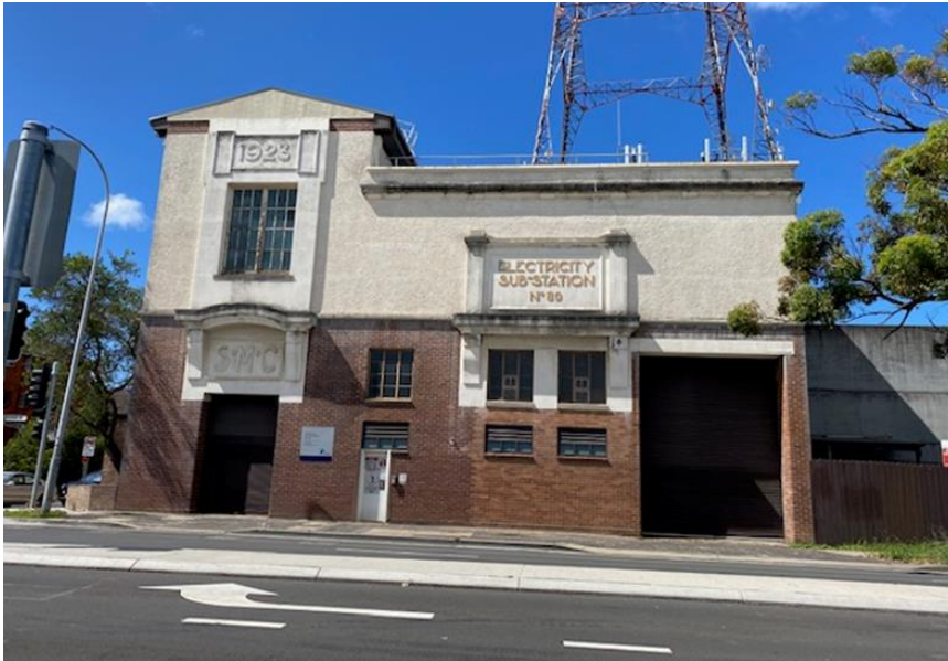
Figure 20 – North Elevation of Chatswood Zone Substation 80.
