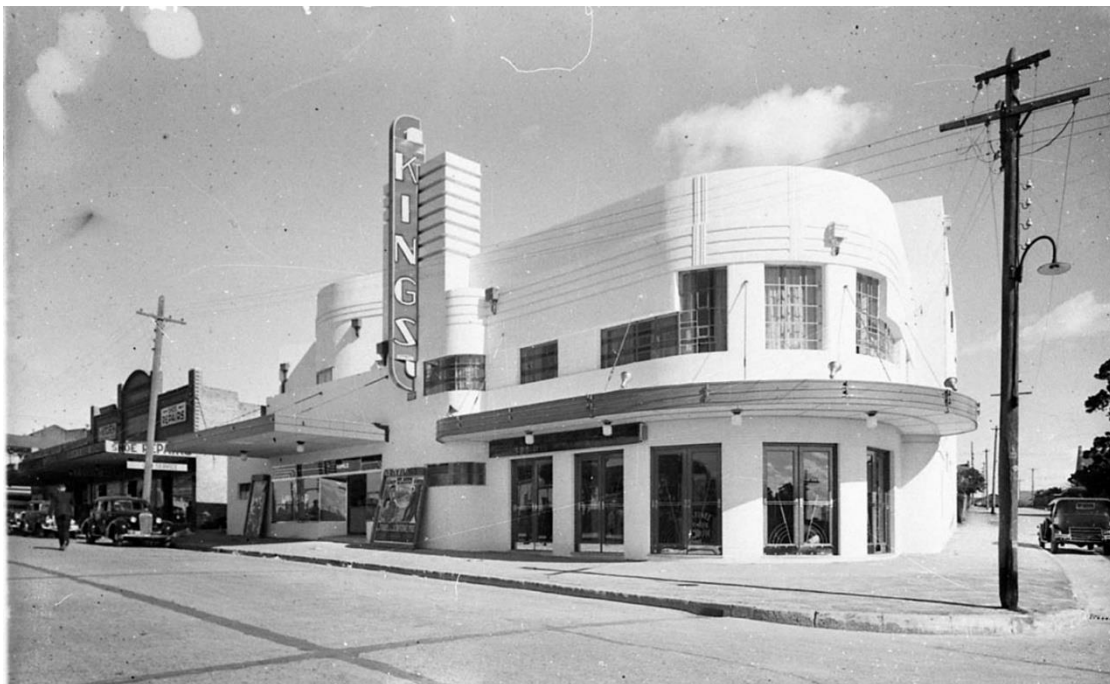
Figure 9 – The Kings Theatre in 1936. Photograph by Sam Hood (1872-1953) Source: State Library of NSW (IE1422245).
