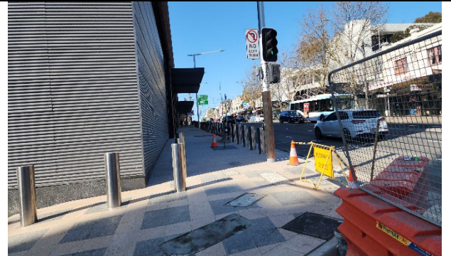
Oxley Street - AWE was cleaning out stormwater drains (flushing) as part of the completion works. Installation of bollards was complete. Pedestrian paving works were ongoing during the inspection.
