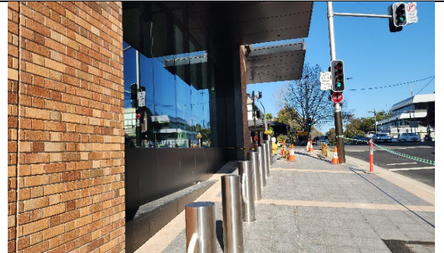
Oxley Street - AWE was cleaning out stormwater drains (flushing) as part of the completion works. Installation of bollards was complete. Pedestrian paving works were ongoing during the inspection.
