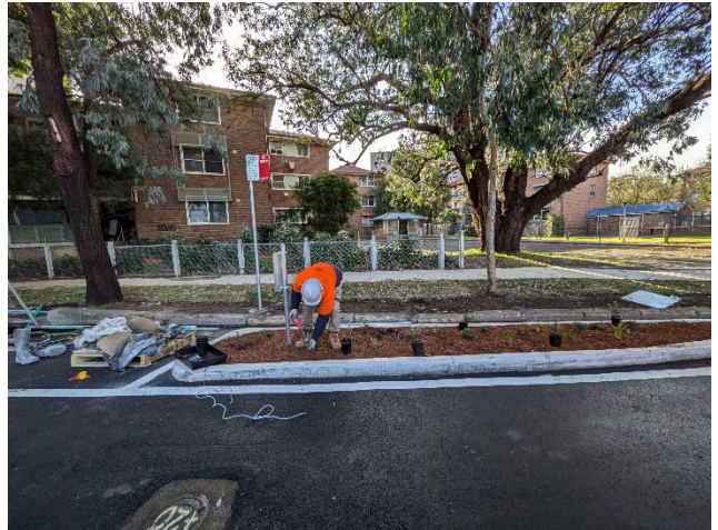
Cope Street: ATF fence removal, planting, demobilisation and clean-up underway.
