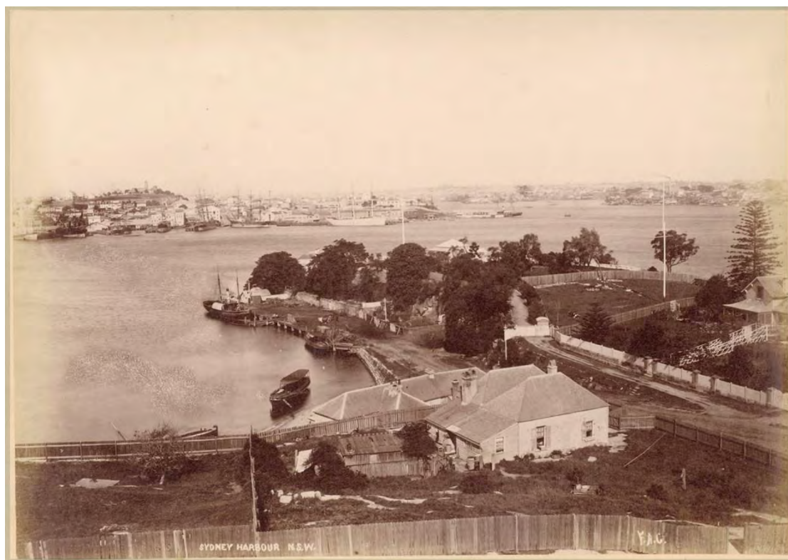
Figure 9: Looking south-west to Blue's Point, showing the roof of the Stevens' cottages in the lower part of the image and the retaining wall all along the foreshore, photograph by F A Coxhead, 1873. Small Picture File SPF/934, Mitchell Library, State Library of NSW.
