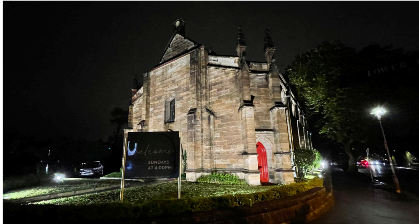
The Garrison Church with new external lighting
