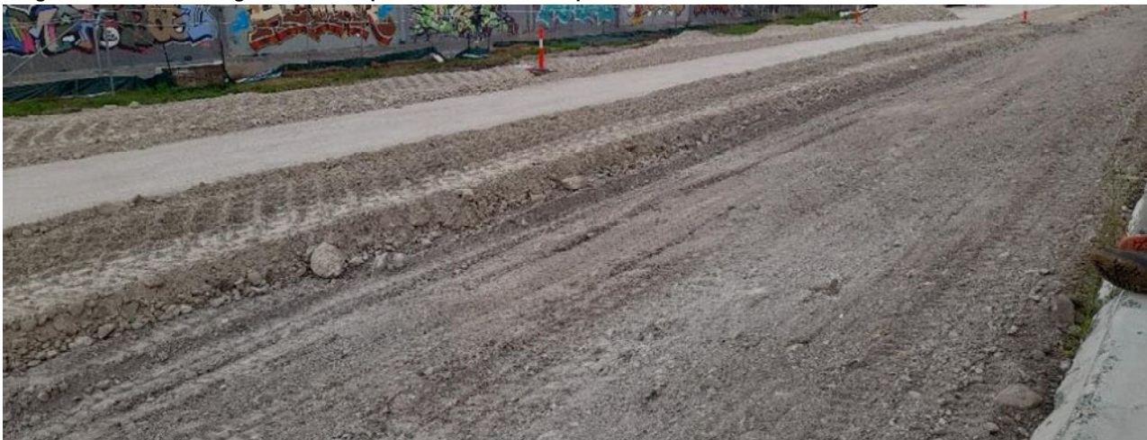
Image 6.2.2.2 View of subgrade material placed across landscaped area.
