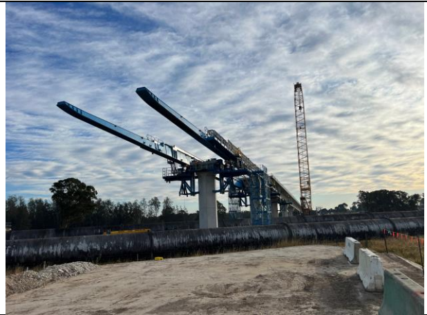
Luddenham North – The viaduct gantry crosses the Warragamba pipelines
