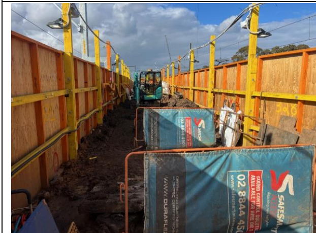
Platform 3/4 – Piling works were undertaken on the platforms with noise blankets and hoardings to reduce noise
