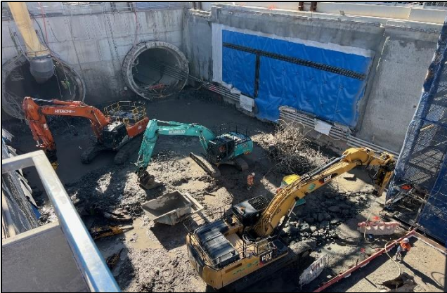
Orchard Hills tunnel portal – TBM launch slab demolition.
