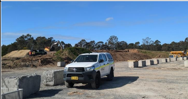
Orchard Hills – Characterisation of eastern topsoil/spoil stockpile
