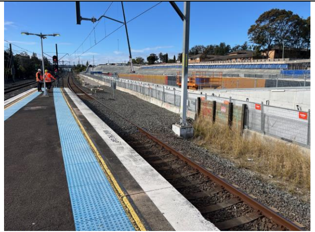
Platform 3/4 - Additional ballast has been placed to facilitate the arrival of Hydrema for WE8 and WE9 works
