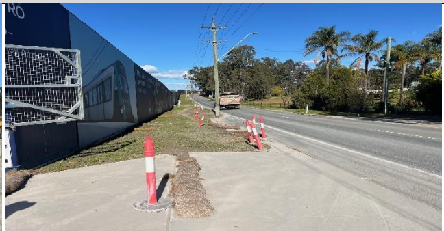
Kent road at site access – Negligible tracking.
