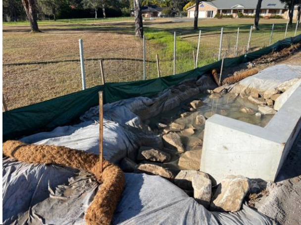
Lansdowne Rd - The access track is nearing completion and the drainage structures have been installed
