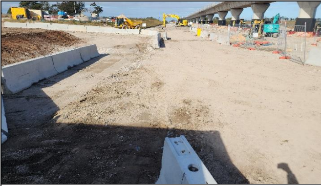
LUD – Earthworks and reduction in swale drain had occurred.
