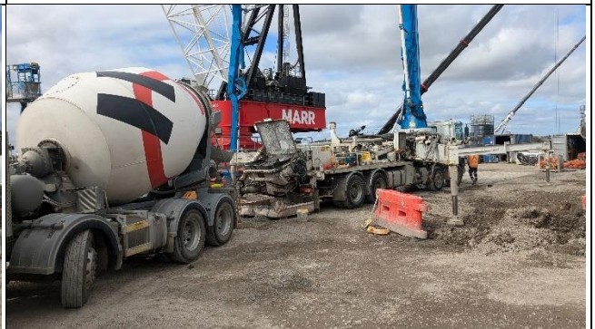
Aerotropolis view east – Concrete delivery.
