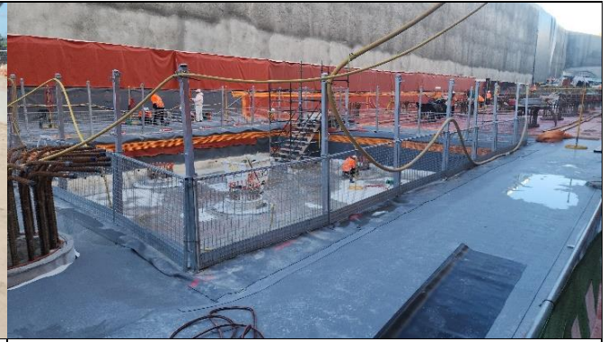
AEC – Construction of the sump and preparation for slabs
