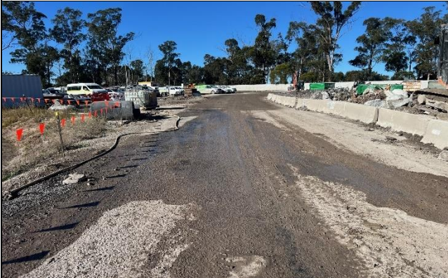
Bringelly – Condition of sealed internal haul roads improved.
