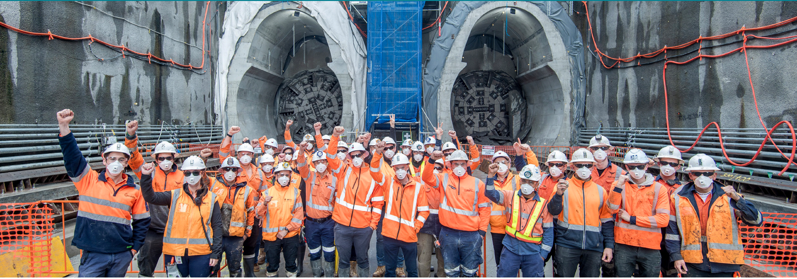
TBM breakthrough in North Strathfield station box.
