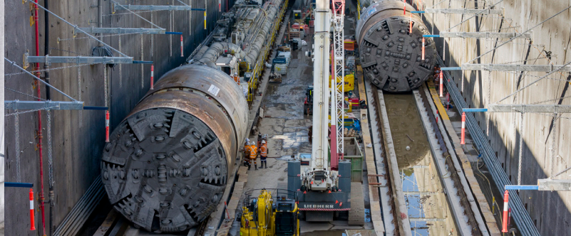
TBMs Daphne and Beatrice in North Strathfield station box.
