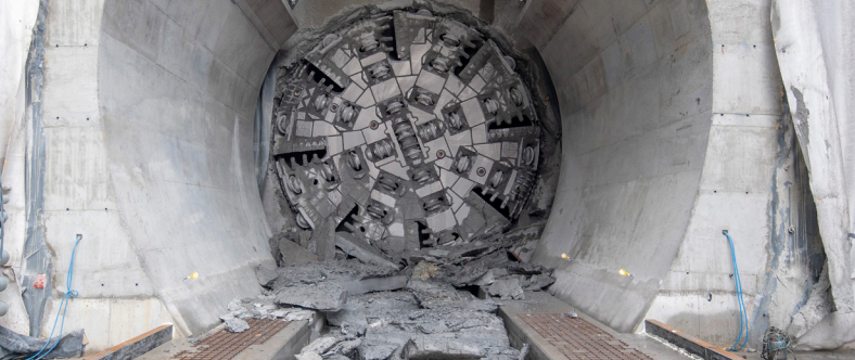
TBM Beatrice breakthrough in North Strathfield station box.
