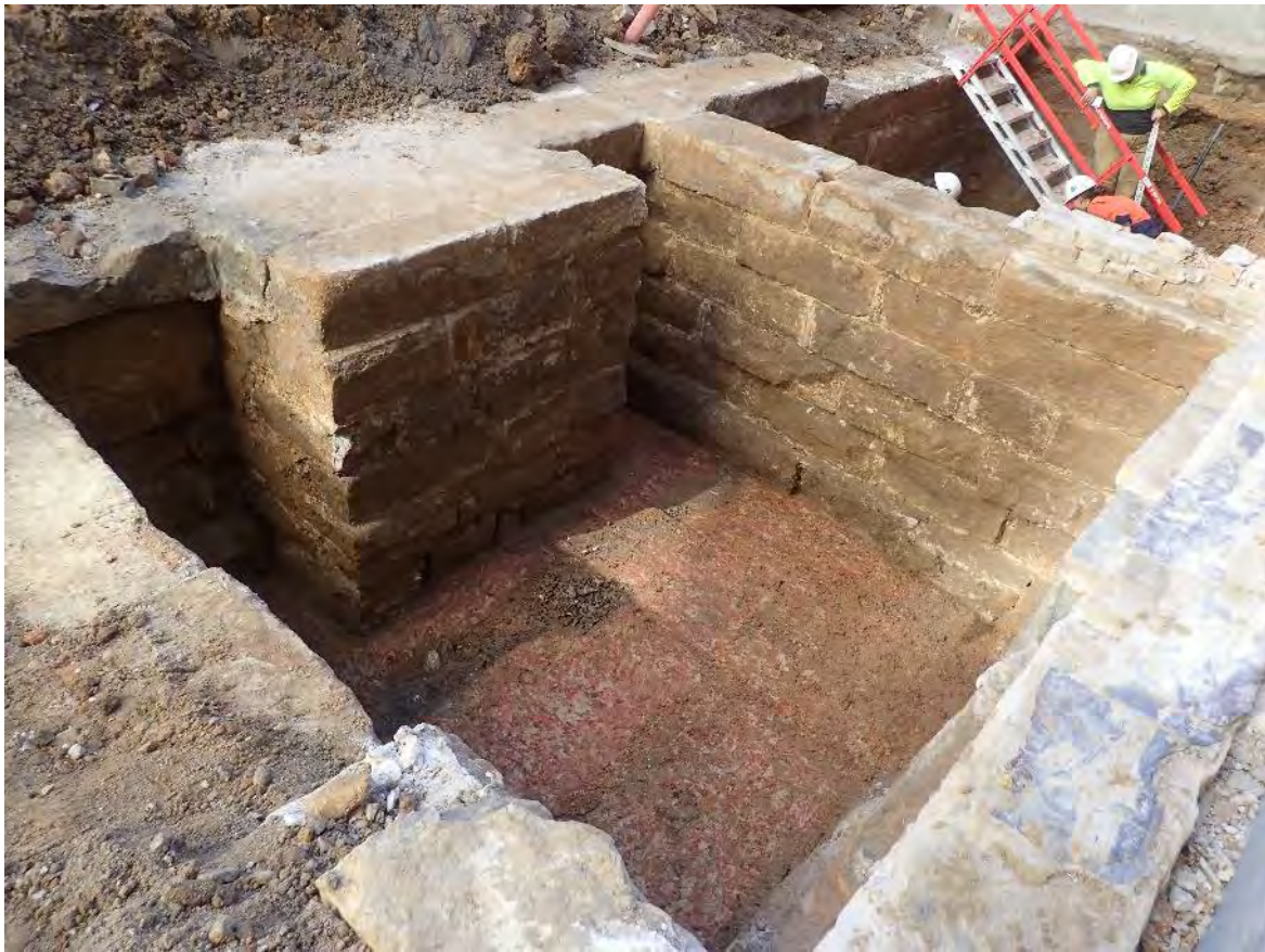
Figure 5.2 House 135, rooms 1 and 2 during excavation, view north-west.
