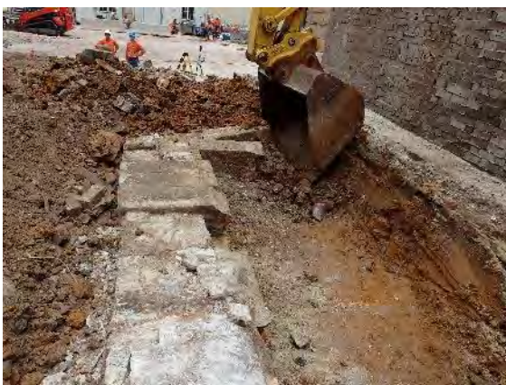
Figure 4.4 View south of sandstone blocks during excavation.
