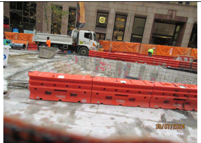
Martin Place: Works to remove existing tiles in the Martin Place stairs.
