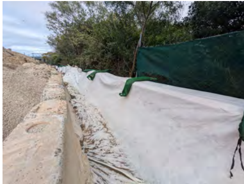
Stockpile controls and slurry management at the Belmore Triangle laydown.
