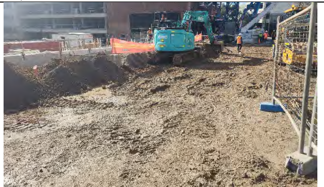
Hume Street Bridge – ongoing water accumulation in the work area had the potential for sediment tracking.
