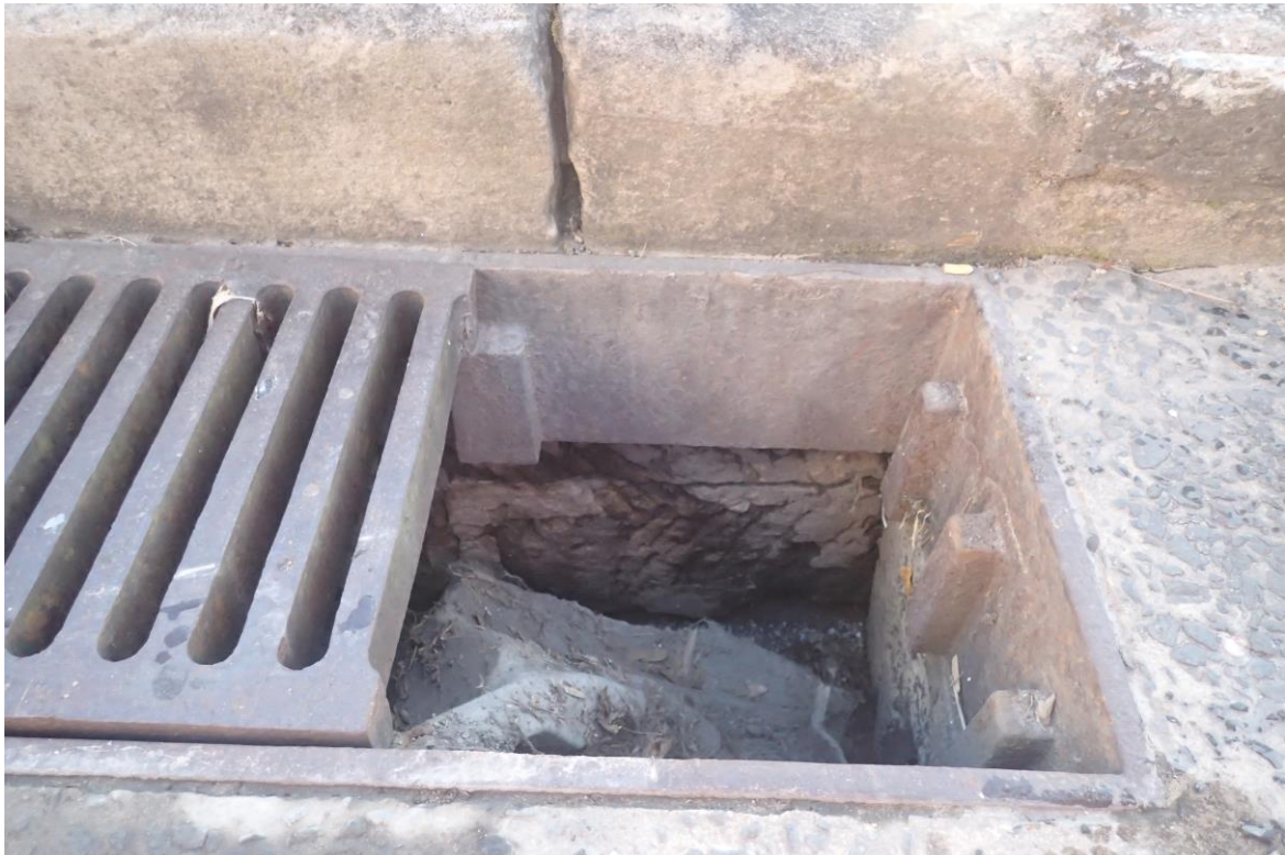
Figure 3.15: The sandstone wall below a course of dressed sandstone used as the footpath running down Blues Point Road.
