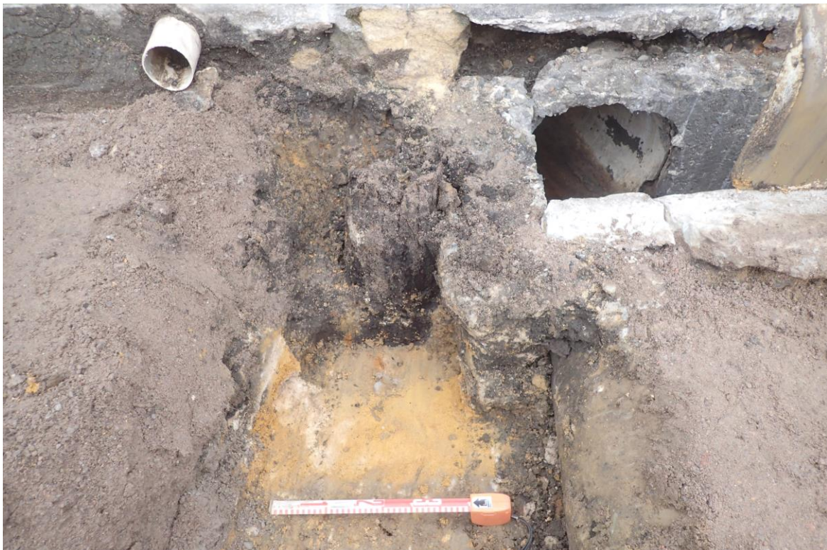
Figure 3.26: Detail of the remains of the wooden telegraph pole alongside the concrete drain with the plastic pipe.
