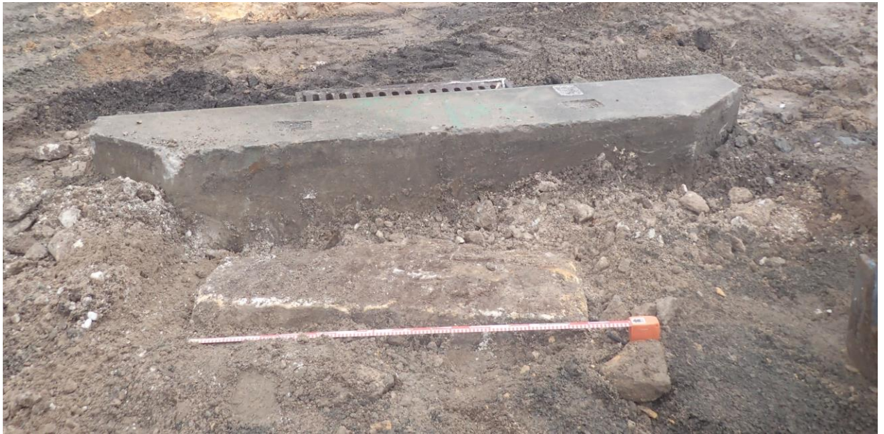
Figure 3.19: View to the west. A sandstone block likely from the 1857 sea wall [333] alongside the stormwater drain pre-excitation.
