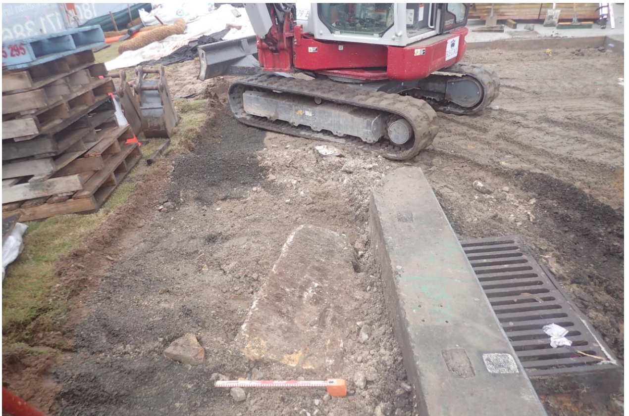
Figure 3.20: Isolated sandstone block potentially from the c.1850 sea wall alongside the stormwater drain and a modern concrete block. View to the south.
