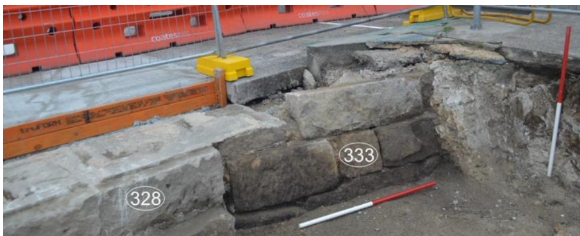
Figure 3.17: c.1800's seawall incorporated into a footpath along east side of Blues Point Rd and connecting to the earlier 1850's sea wall. View to north-west. Source: Casey & Lowe 2021. Figure 4.89.P.173.
