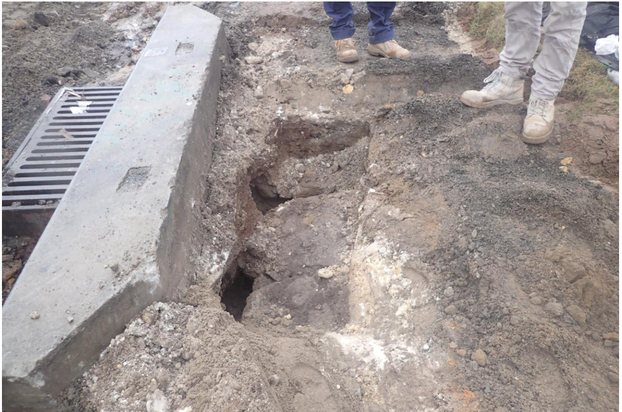
Figure 3.21: A second course of sandstone blocks, lying west-east witnessed below the isolated sandstone block potentially from the early seawall [328].
