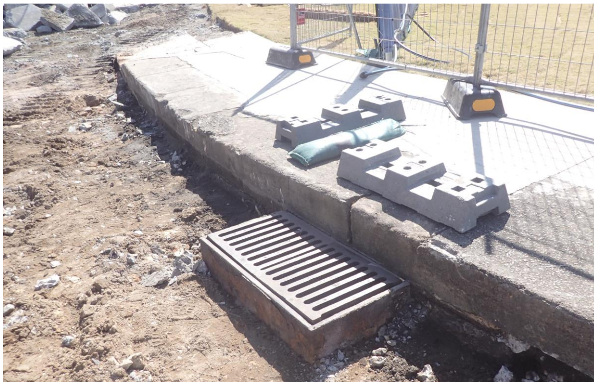
Figure 3.14: Partial footpath along Blues Point Road with sandstone kerbing still in use in 2022.
