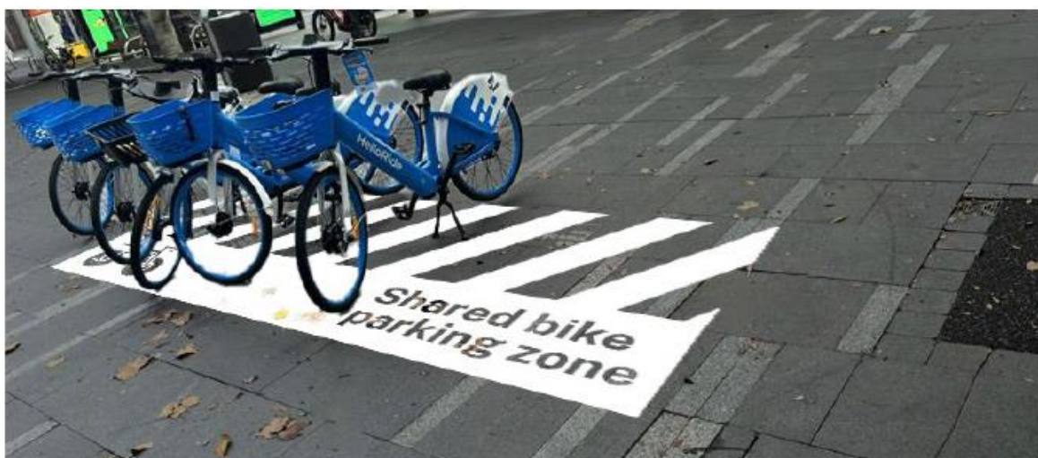
Figure 2 Example of pavement painting and line marking
