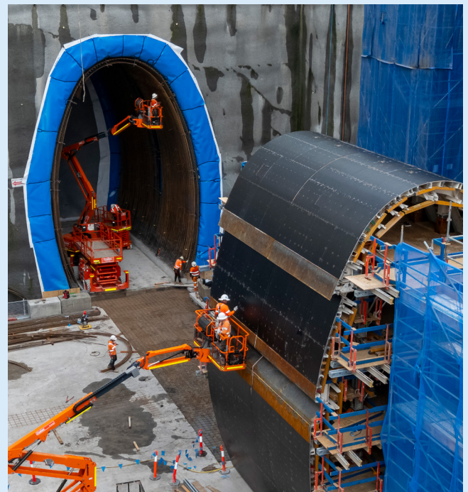
Tunnel nozzle excavation at Sydney Olympic Park Metro Station site
