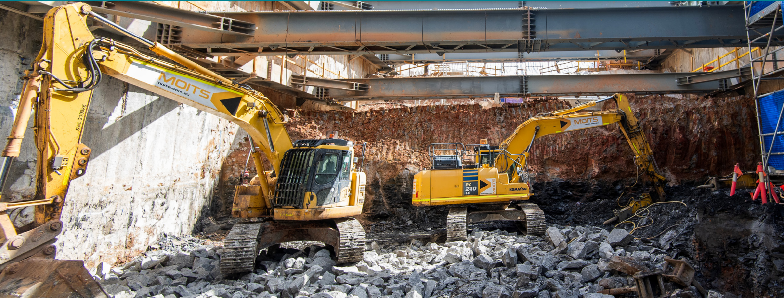
Station box excavation at Parramatta Metro Station site
