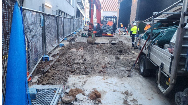
Clarke Lane North – Excavation of Clark Lane adjacent to a culvert without erosion controls installed.
