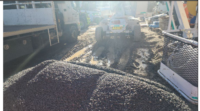
Hume St Bridge – Muddy area on Hume Street bridge requiring mitigation to prevent tracking.
