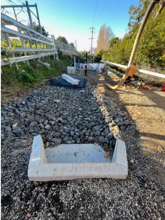
Installation of stormwater infrastructure, Ewart Street Dulwich Hill.
