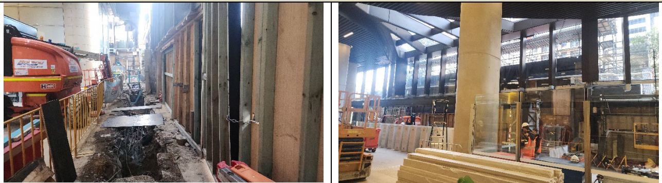
PSN – installation of bollards and Park Street entrance.
