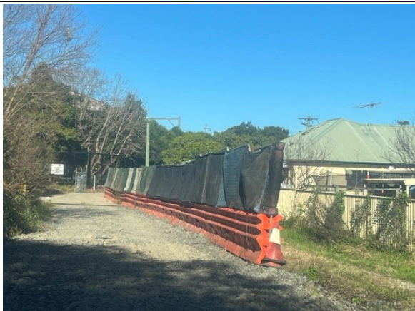
Maintenance of noise blanket wall at the Belmore Triangle site access.
