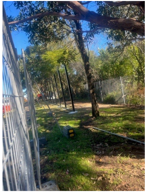
Ongoing redesign for tree retention, Wiley Park.
