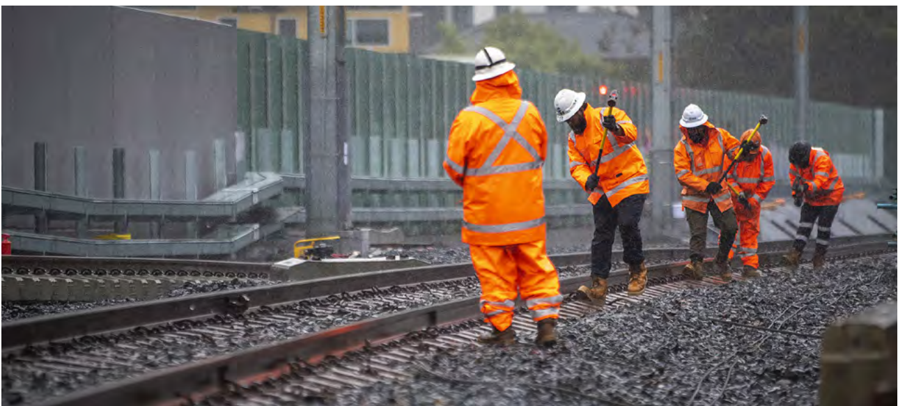
Track cutting works between Artarmon and Chatswood stations.
